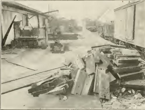
Fig. 15—Furnace for Melting Liners from Shoes and Wedges
