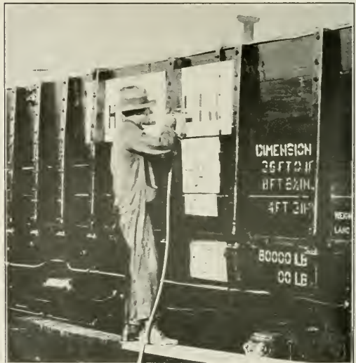
Fig. 3—Paint Sprayer Used for Stenciling.
