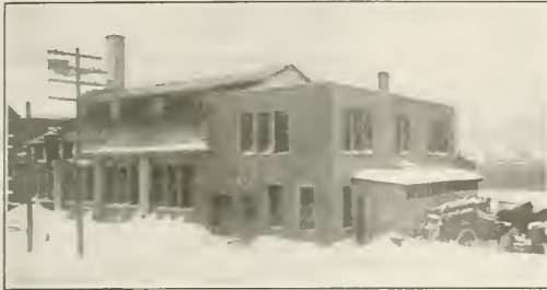
Fig. 1—Original Quarters of the Onondaga Steel Co., Inc., at Syracuse, N. Y.
