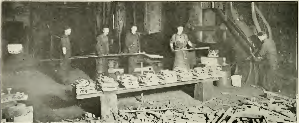
Scrap Iron Cut and Piled Ready for Heating
