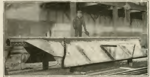
Fig. 2—Main Floor Member Being Assembled. Note Extension at End for Attachment to Center Sills
