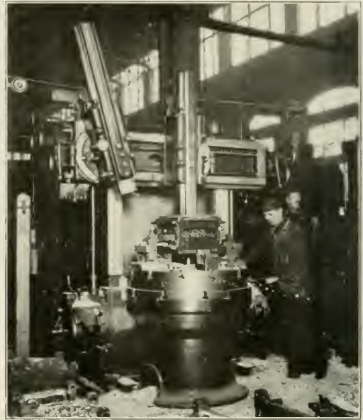
Fig. 9—Turning Driving Boxes on Gisholt Boring Mill
