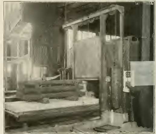
Fig. 2—Electric Furnace and Charging Car
