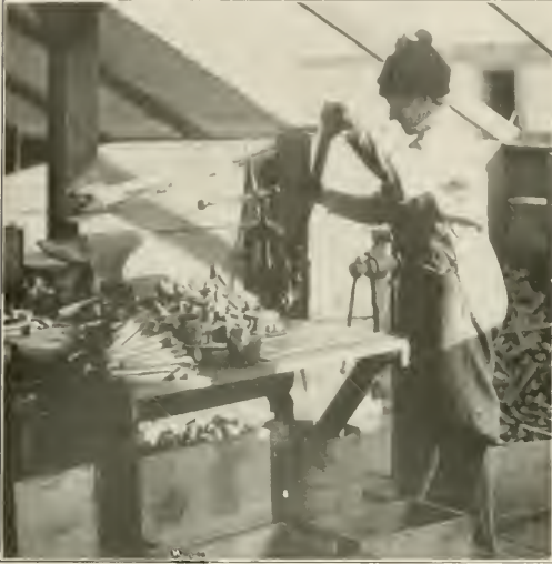
Fig. 7—Reclaiming Track Bolts
