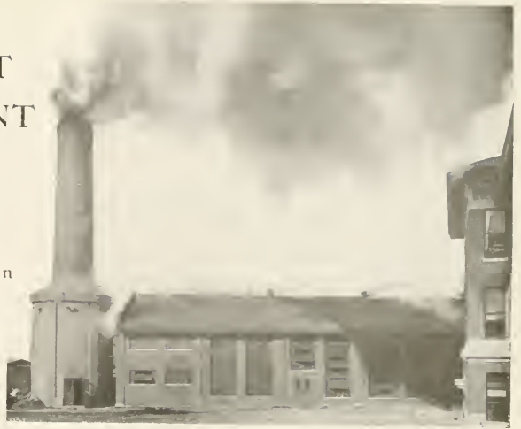
The University of Illinois Test Plant in Action
