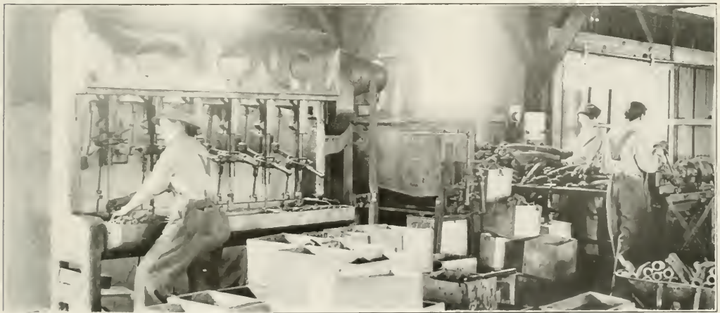
Fig. 5—Rethreading Nuts and Stripping Old Air Hose
