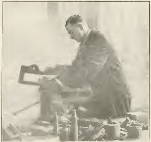
Third Year Apprentice Working in Link Gang
