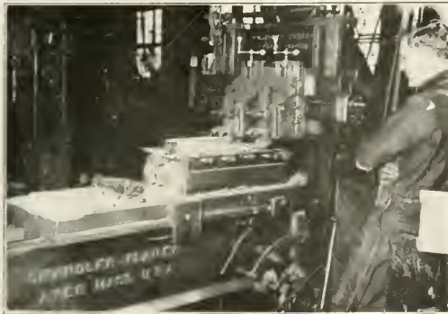
Fig. 12—Machining Shoes and Wedges
