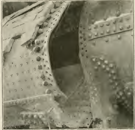
Wrapper Sheet Seam which Failed Due to Low Water
