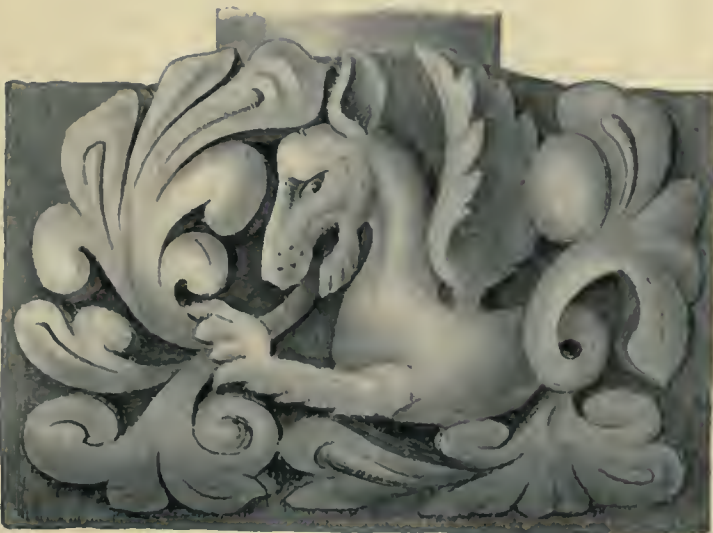
Corbel, South Arcade of Nave.
