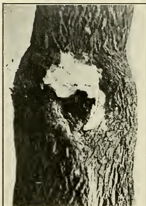
FIG. 307—HOW NOT TO COVER A CAVITY WITH CEMENT OR CONCRETE
