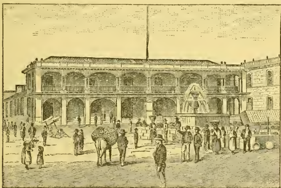
The Government Building, Quezaltenango.
