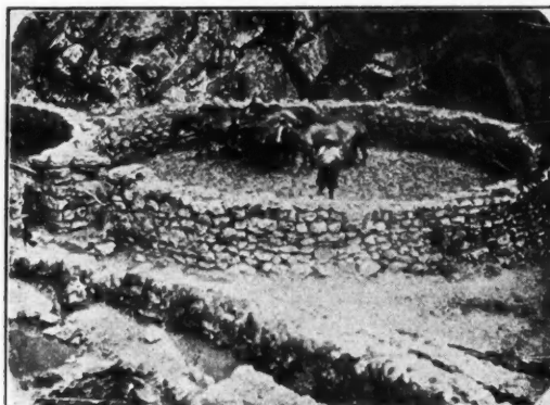
THE "ARRASTRA," FOR GRINDING ORE
