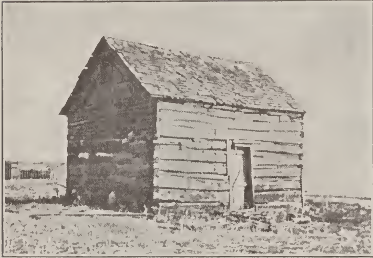
Poorly Ventilated House
