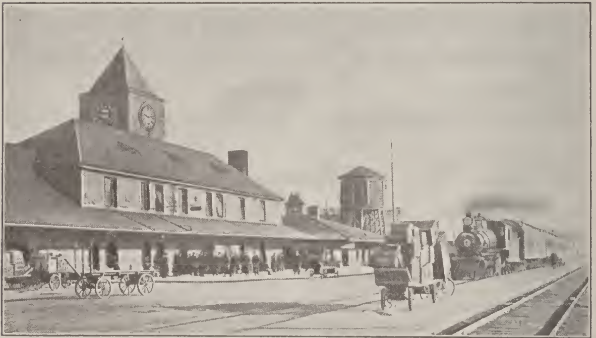
Great Northern Station
