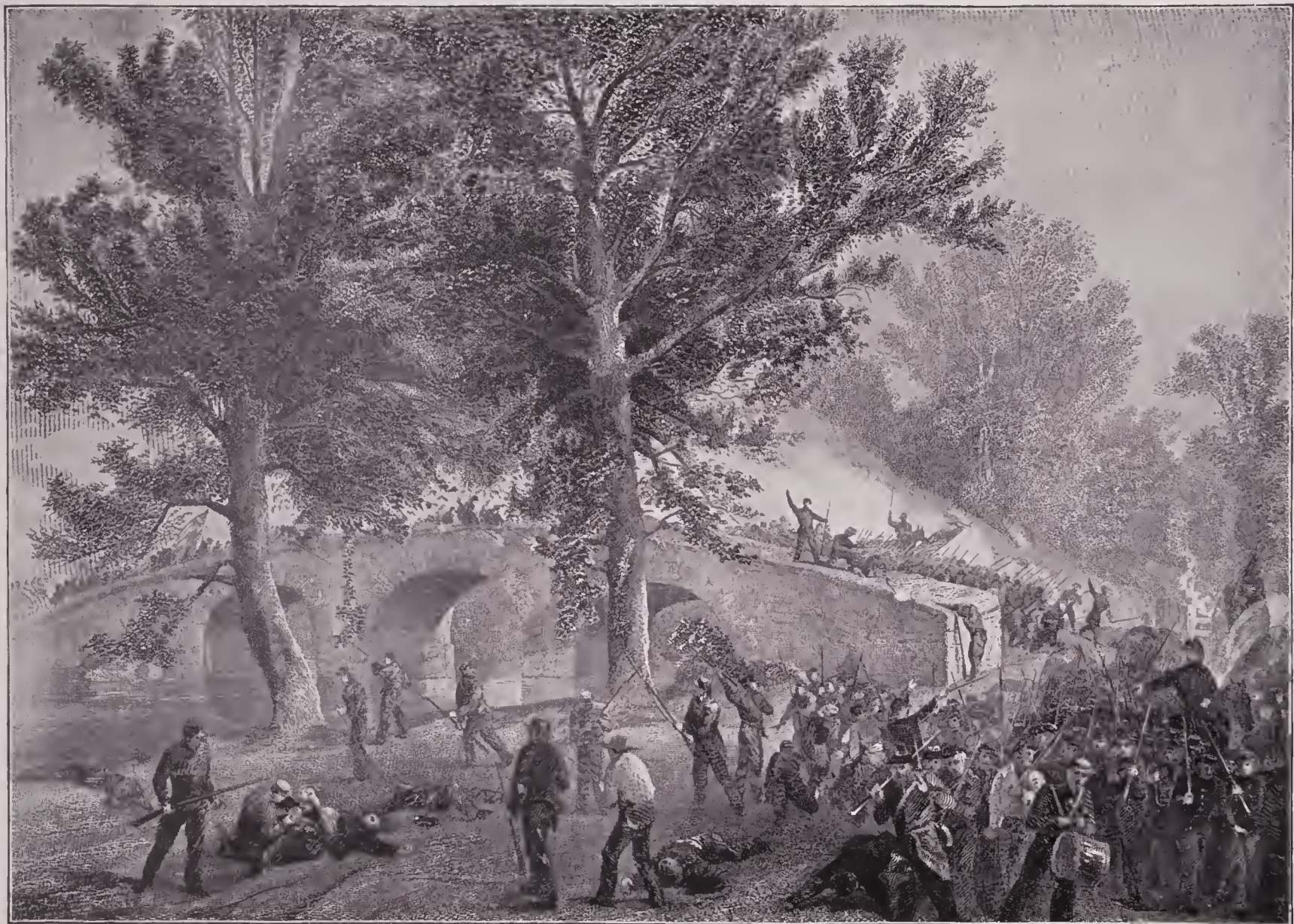
THE CHARGE ACROSS THE BURNSIDE BRIDGE.
