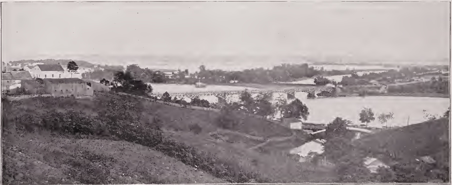
AQUEDUCT BRIDGE, POTOMAC RIVER.
