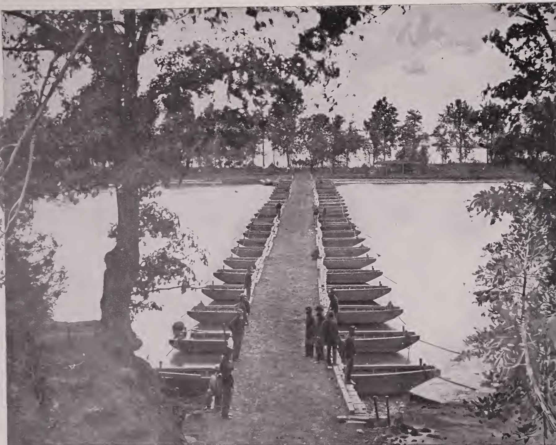
PONTON BRIDGE AT DEEP BOTTOM ON THE JAMES RIVER.
