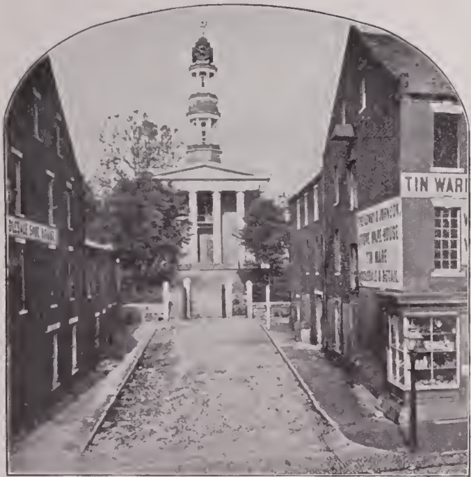
COURT HOUSE, PETERSBURG, VA.
