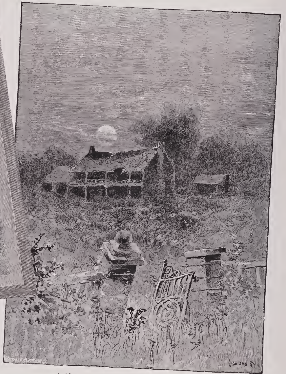
A SOUTHERN PLANTER'S RESIDENCE IN RUINS.
