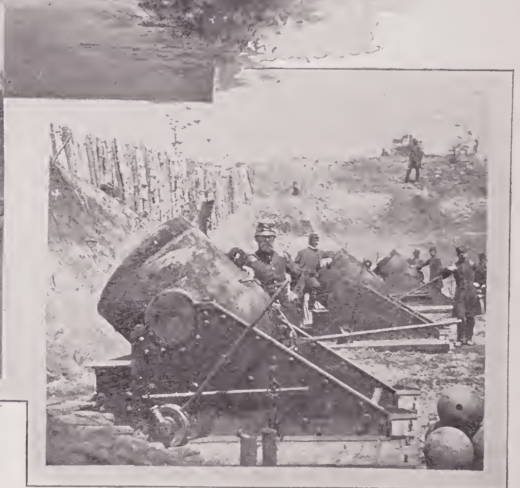
BATTERY No. 4 IN FRONT OF YORKTOWN.
