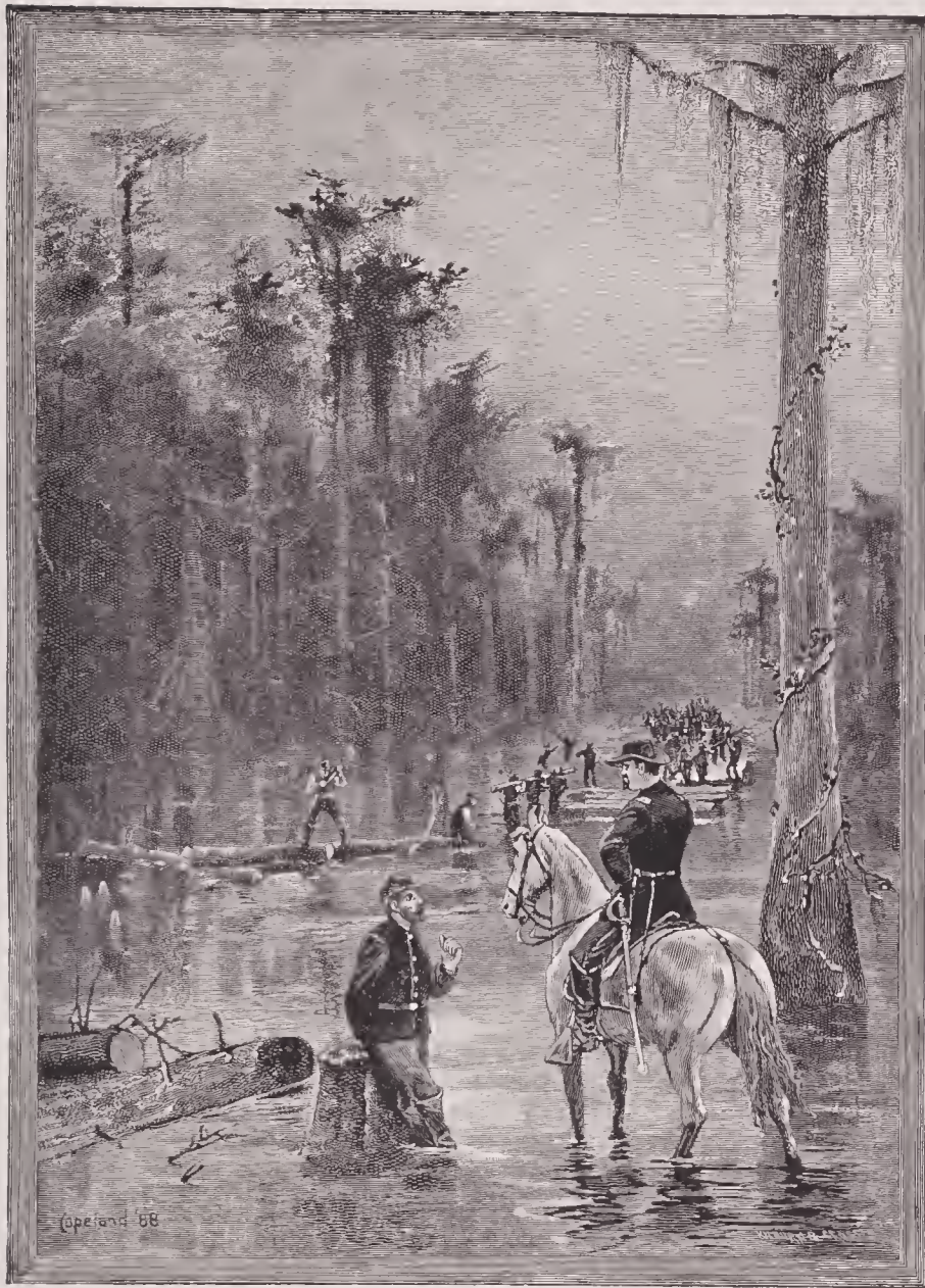
CONSTRUCTING MILITARY ROAD THROUGH SWAMP
