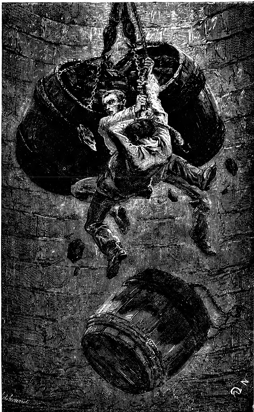
COLLISION OF TUBS IN A SHAFT.
