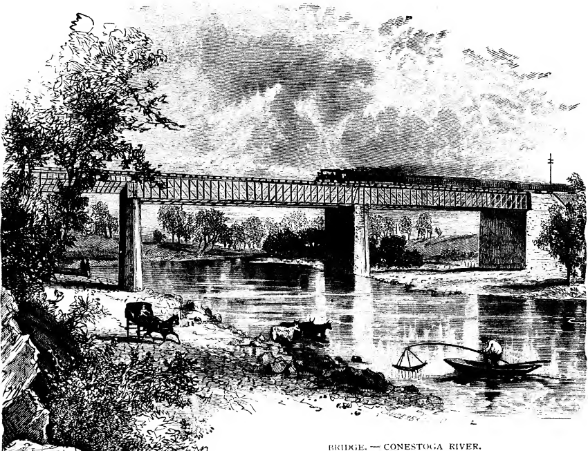
BRIDGE. — CONESTOGA RIVER.
