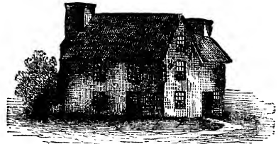
WHITEFIELD'S HOUSE, LOOKING SOUTH.
