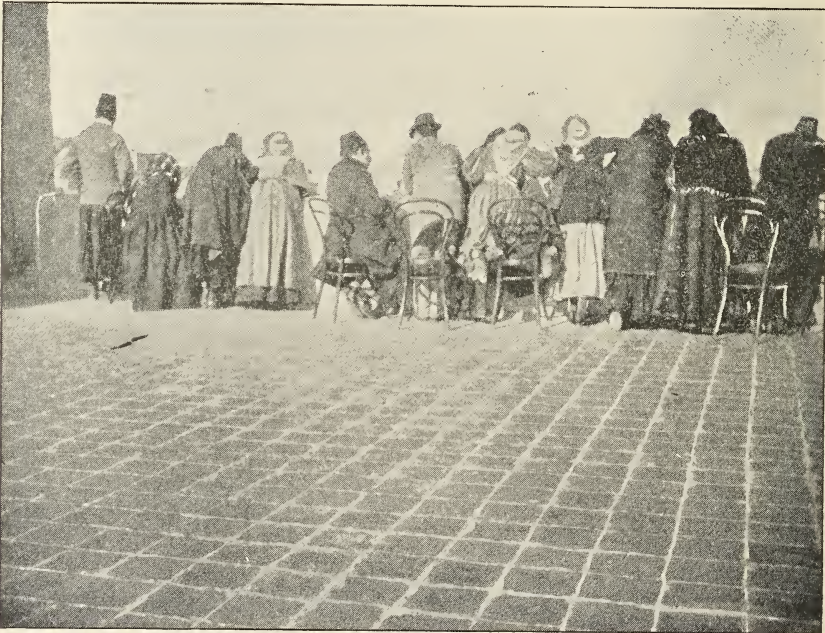
ON THE ROOF.
