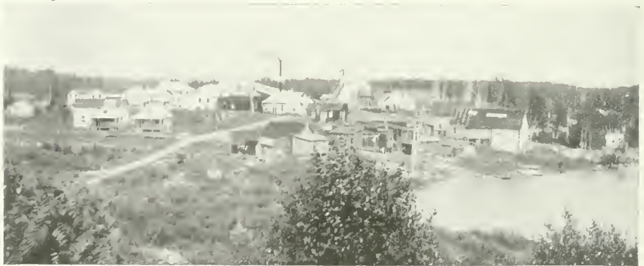
Teek-Hughes mine, June, 1919. The two buildings with verandahs in the foreground on the left belong to the Kirkland-Porphry.
