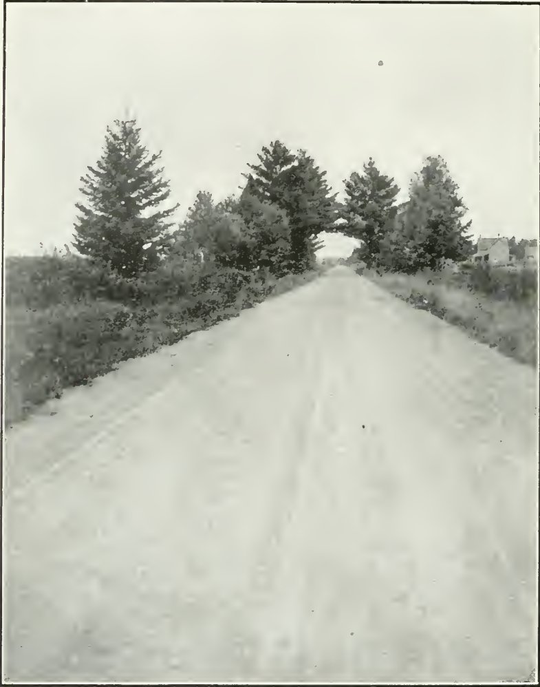
A view of the Trunk Road between the town of Pembroke and Petawawa Military Camp, showing a stone road re-surfaced with coarse gravel.
