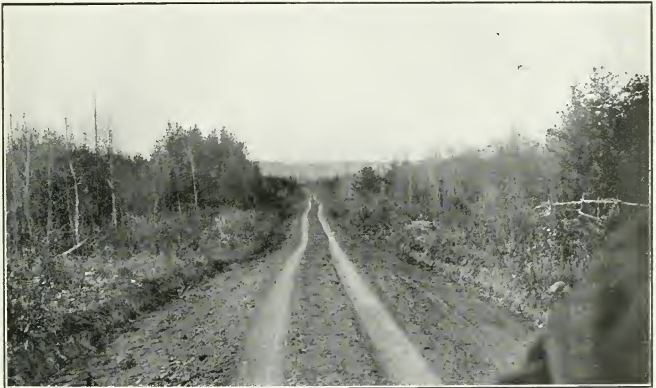
On the Oliver Trunk Road west of Port Arthur; road surfaced with shale.
