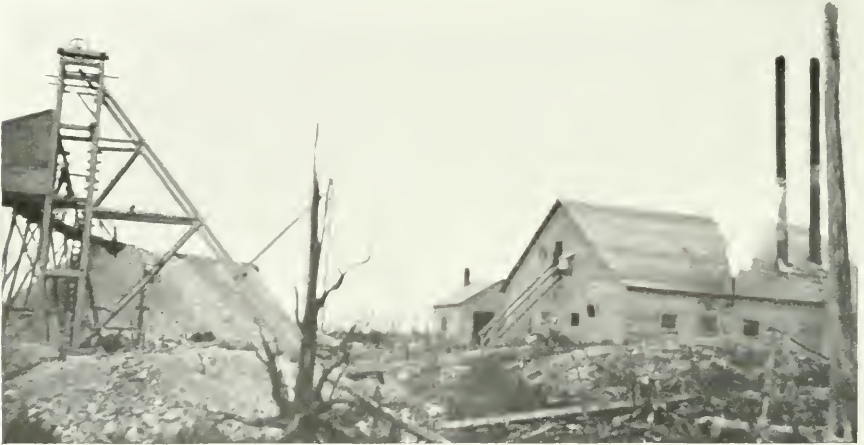
Fig. 45—Compressor building and shaft house, Raty claim, Rickard township.
