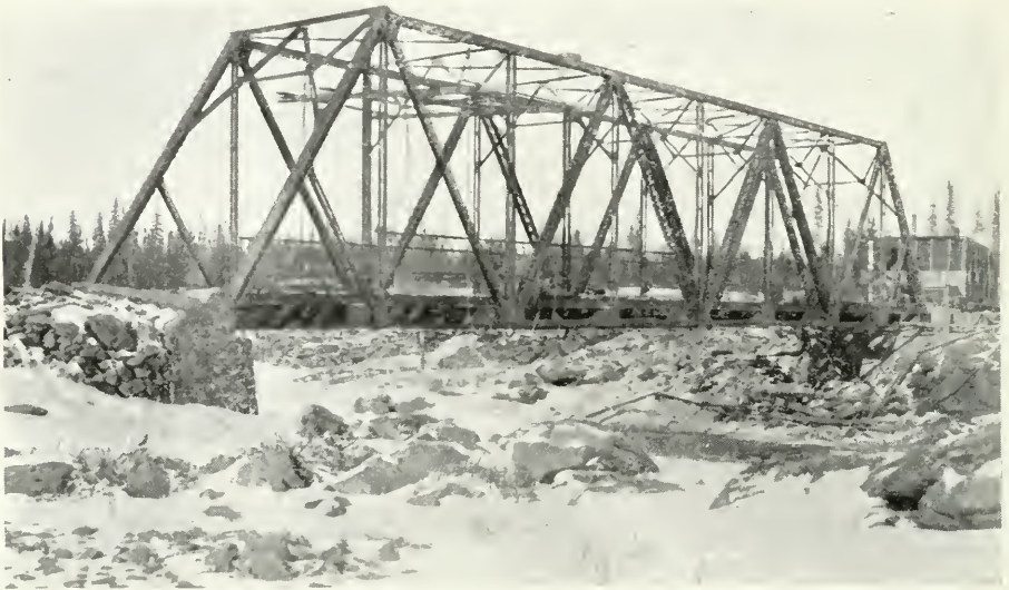
Steel bridge at Kapuskasing: erected 1919.
