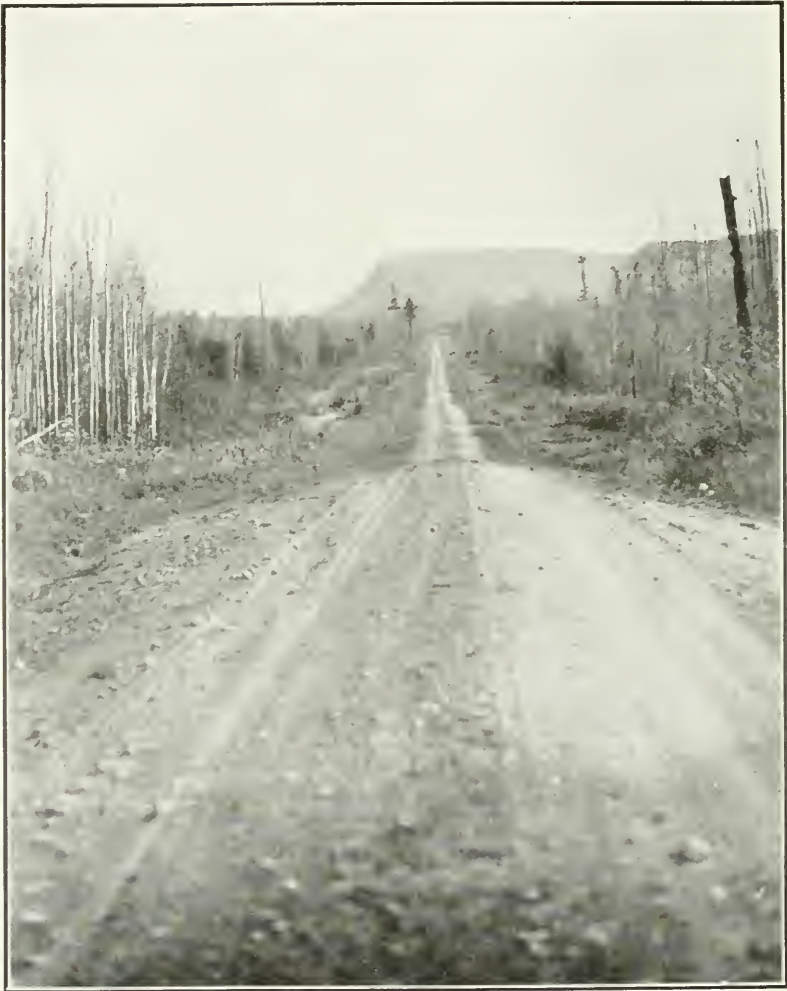
A view looking south on the International or Scott Highway, showing the mountain ranges overlooking Lake Superior.
