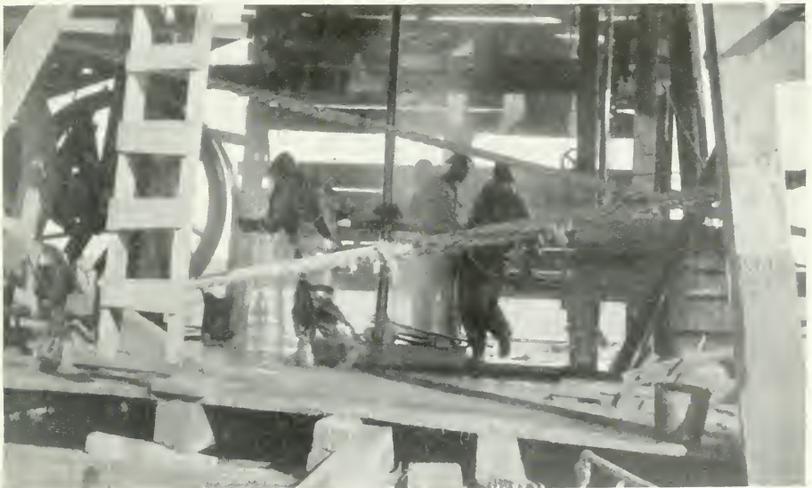
"Bucking up" the tubing. "No sleep until the well is closed in."
