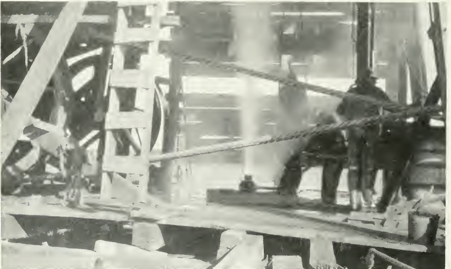
First operation of tubing a seven million well, 3-inch tubing being used.
