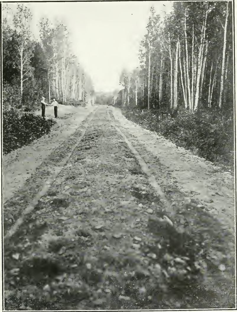
Gravelling a new road between Dryden and Wabigoon, in the District of Kenora.
