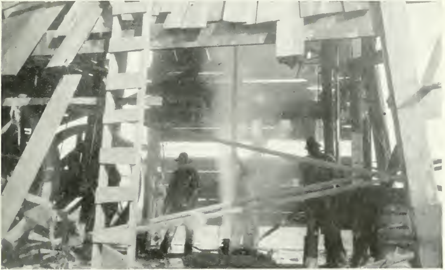
Swinging a length of 3-inch tubing to place over the high pressure gas flow.
