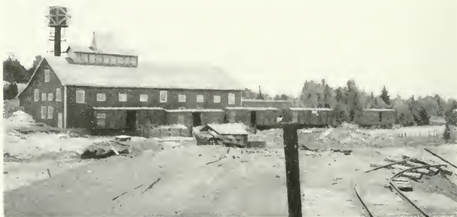
Electric furnace for producing ferro-chrome, Cordova Mines.
