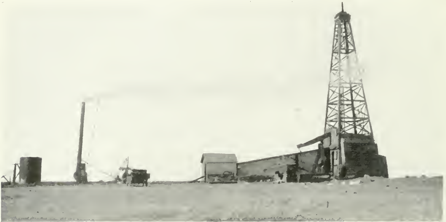
Drilling a gas well.
