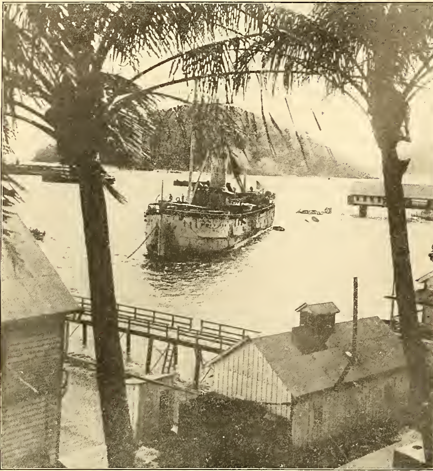
DEEP SEA DREDGE AT BALBOA
