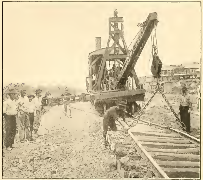
THE TRACK SHIFTER IN ACTION
