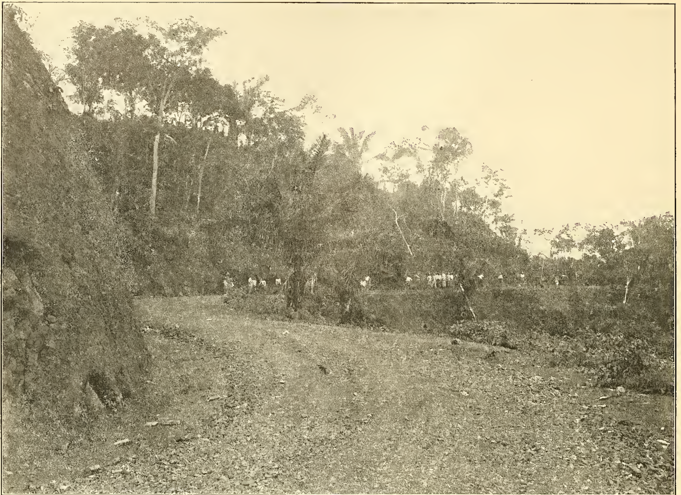
CONVICTS BUILDING A COMMISSION ROAD
