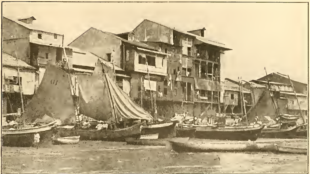
THE PANAMA WATER FRONT
