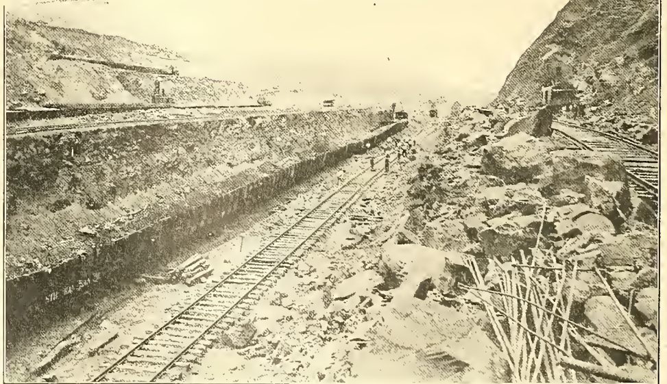
CUTTING AT BASE OF CONTRACTORS HILL
