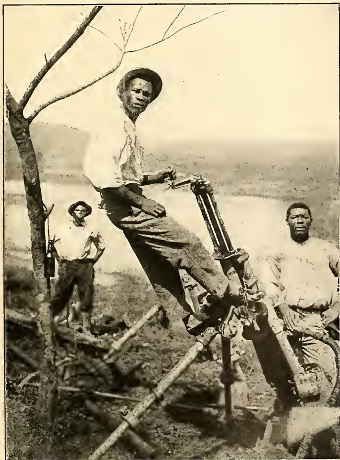
JAMAICANS OPERATING A COMPRESSED AIR DRILL,
