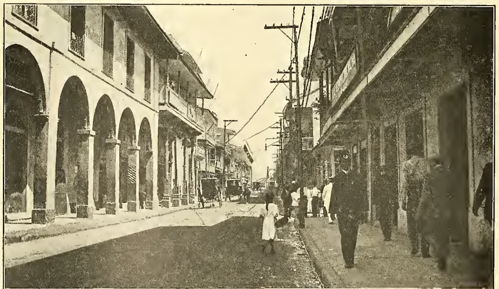
A STREET AFTER PAVING
