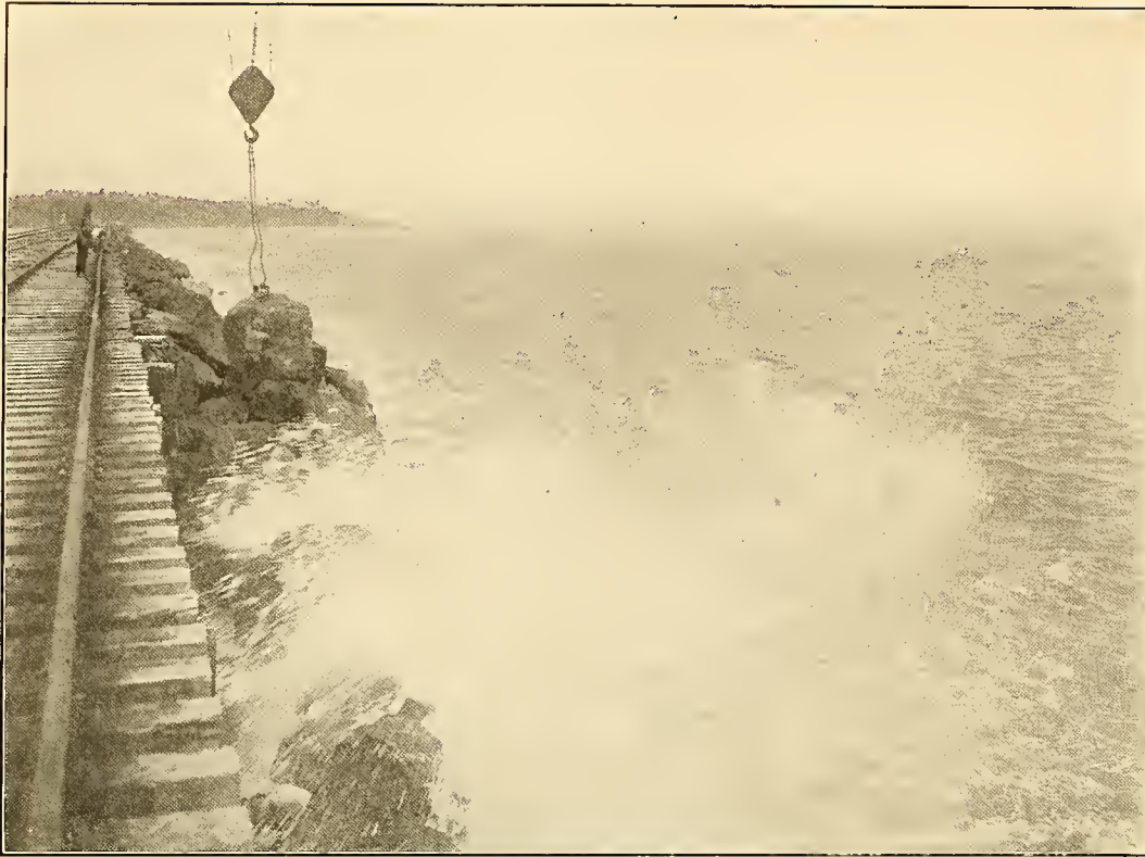
TORO POINT BREAKWATER
