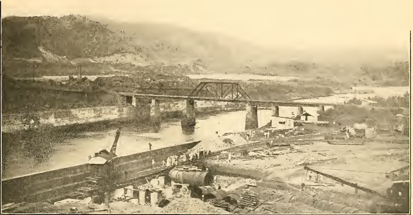
THE PANAMA RAILROAD BRIDGE AT GAMBOA
