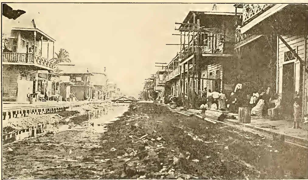
AN OPEN SEWER IN A COLON STREET
