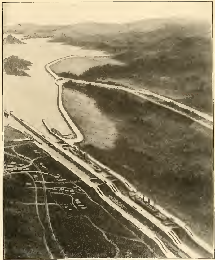
BIRD'S EYE VIEW OF GATUN DAM
