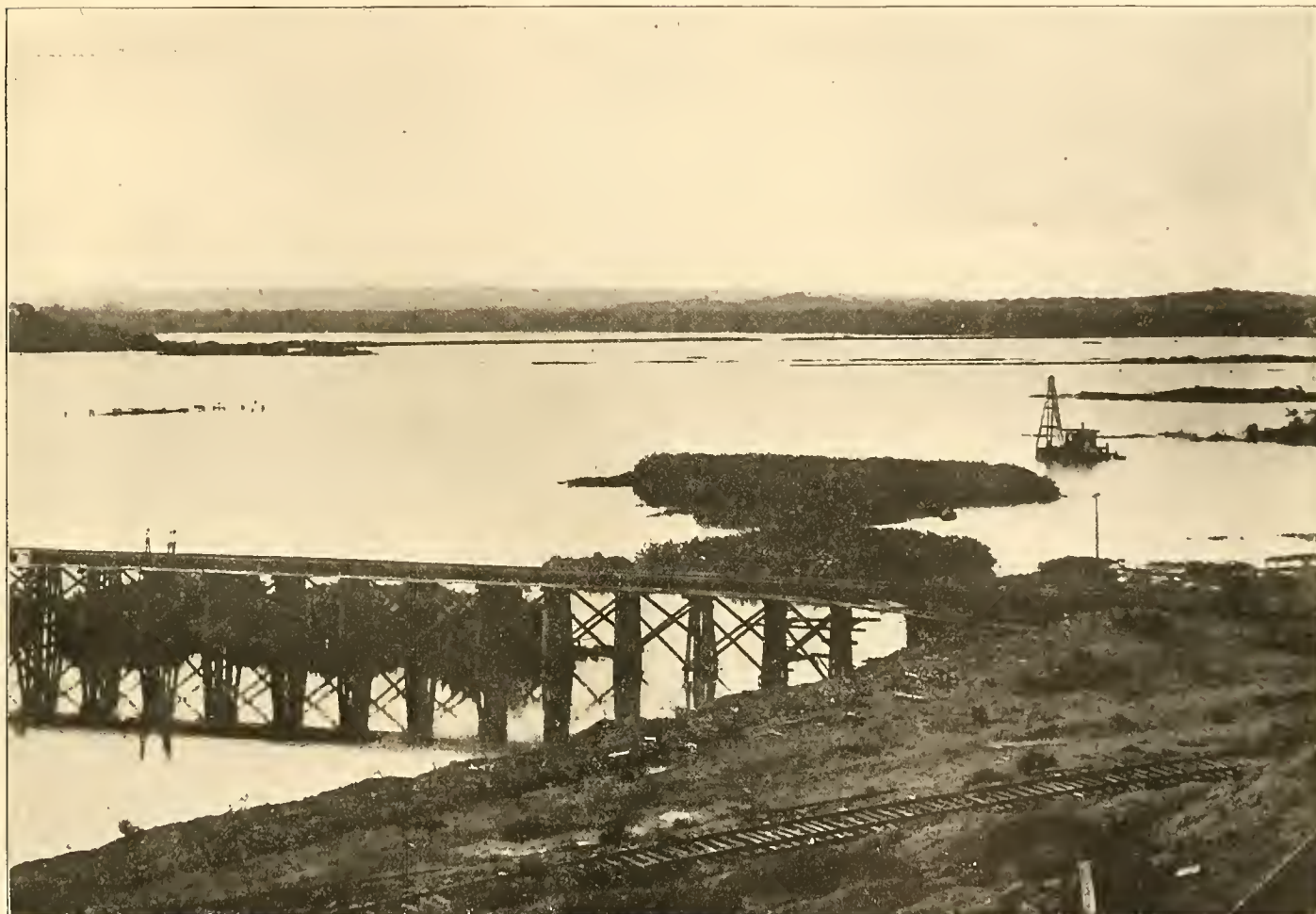
GATUN LAKE. FLOATING ISLANDS MASSED AGAINST TRESTLE
