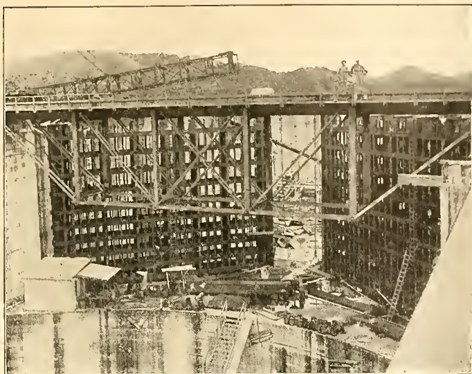
BUILDING AN UPPER TIER OF LOCKS
