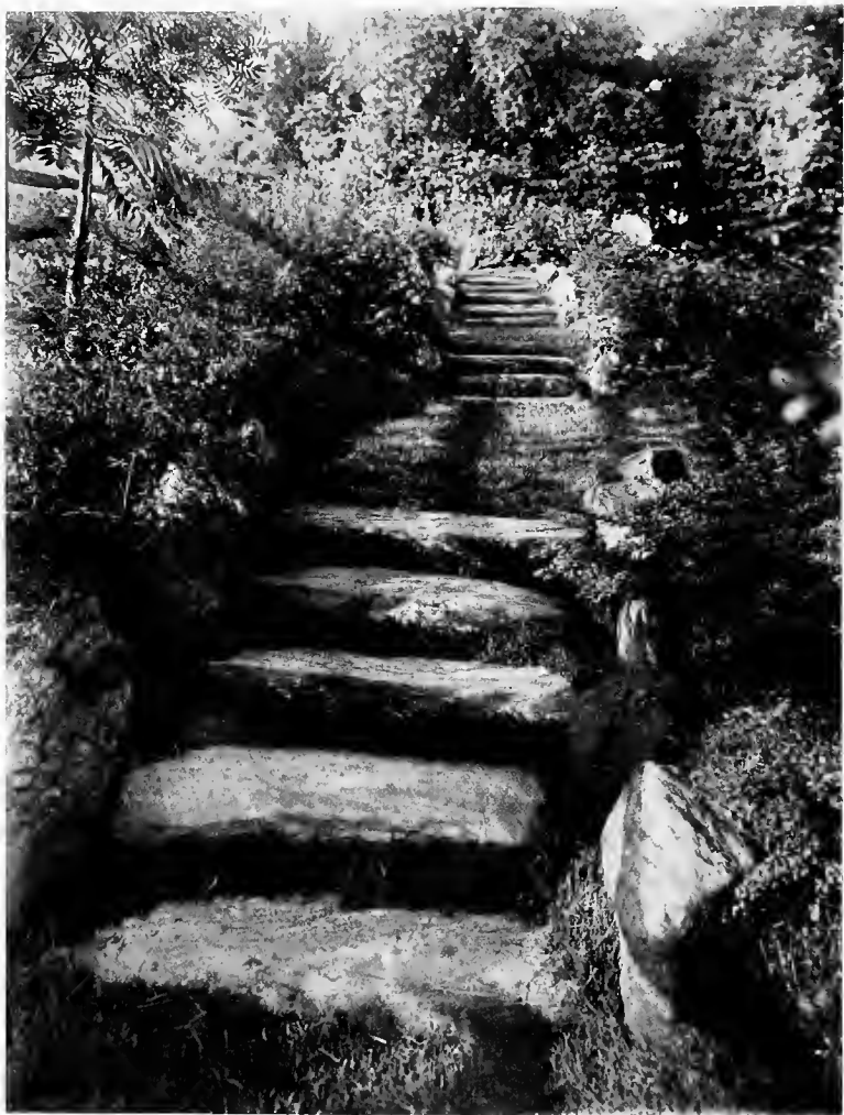
Fig. 176.—Stone steps making an interesting approach to the rock garden. Large field stones form the treads with earth risers. Sedum acre (Wall Pepper) is planted between the stones.—See page 229
