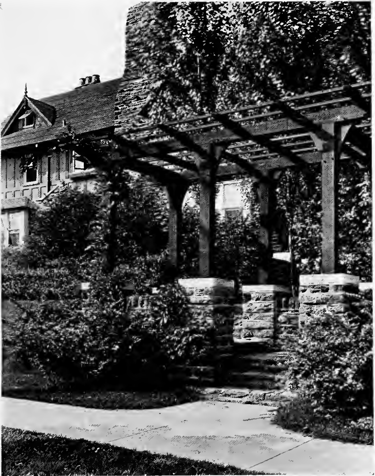
Fig. 33.—Entrance arrangement for house on a level just slightly higher than the pavement.—See page 39
