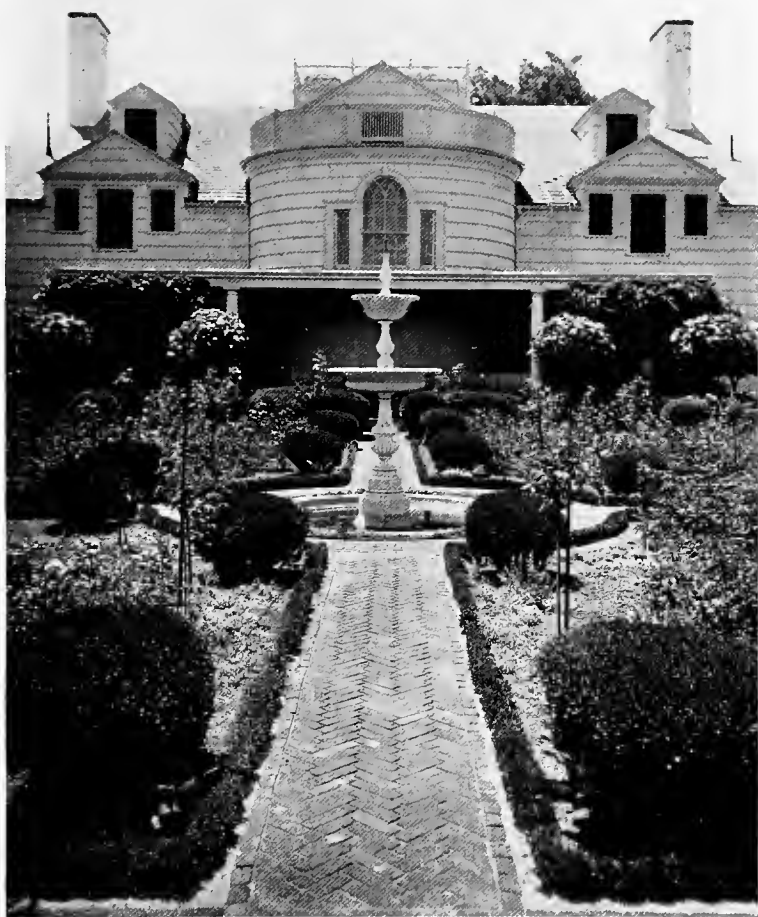
Fig. 129.—Brick garden walk, laid diagonally on edge and bordered with Box.—See pages 155, 156
