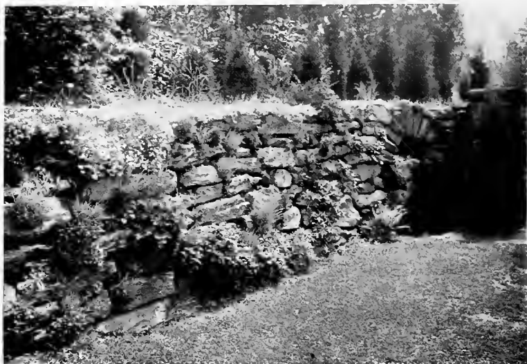
Fig. 172.—A dry retaining wall with pockets for plants, where the water feature adds greatly to the scene.—See page 226
