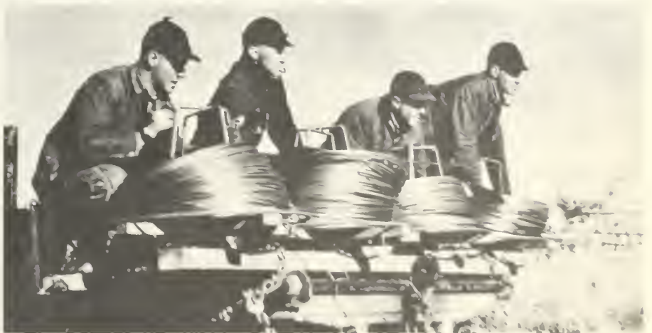
A series of crews was able to complete several miles of electric line each day. After previous crews had marked out the sites, dug holes, and erected the poles and hardware, the line was played out. Subsequent crews would attach the wires and hardware to the poles, and connect individual homes to the high line.
