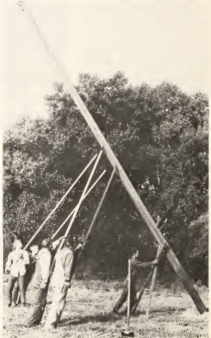
... and the new pole lifted and set into place.
