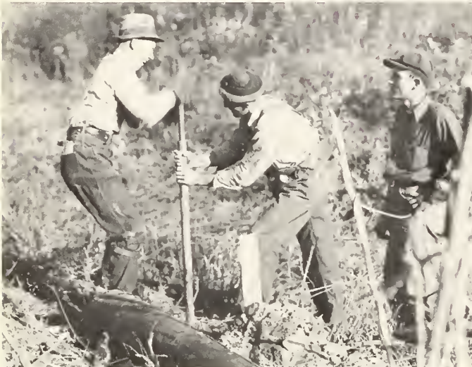
Early crews had few power tools to work with. Holes were dug by hand...
