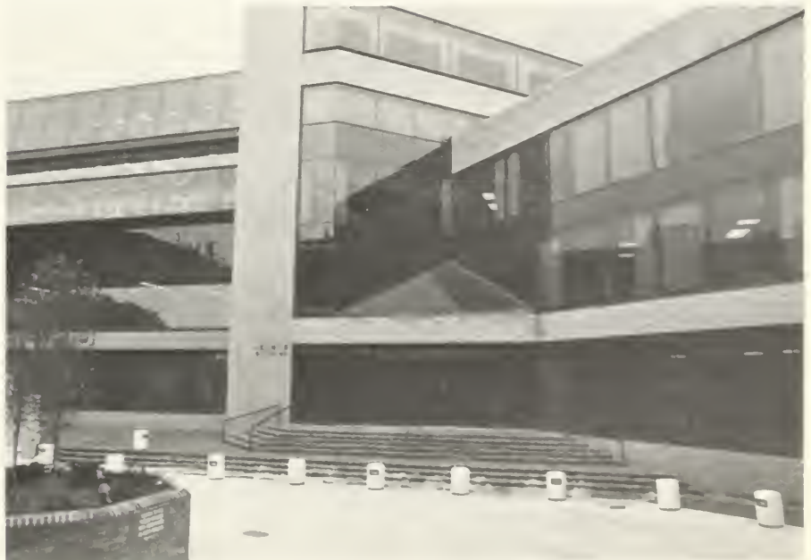
The National Rural Utilities Cooperative Finance Corporation (CFC), an independent, self-help credit institution, was created by rural electric systems to provide themselves with a supplemental finance source. By investing their own funds in CFC as seed capital, the rural systems created a basis for additional credit utilizing funds borrowed from other sources.
