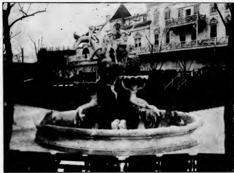
New Electric Fountain at Steeplechase Park, Coney Island, New York.
