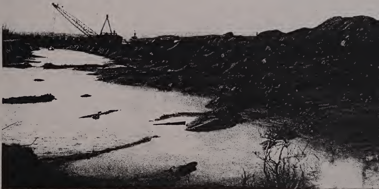
Land Excavator at Work on the High Land near Sagamore, April 1910.
