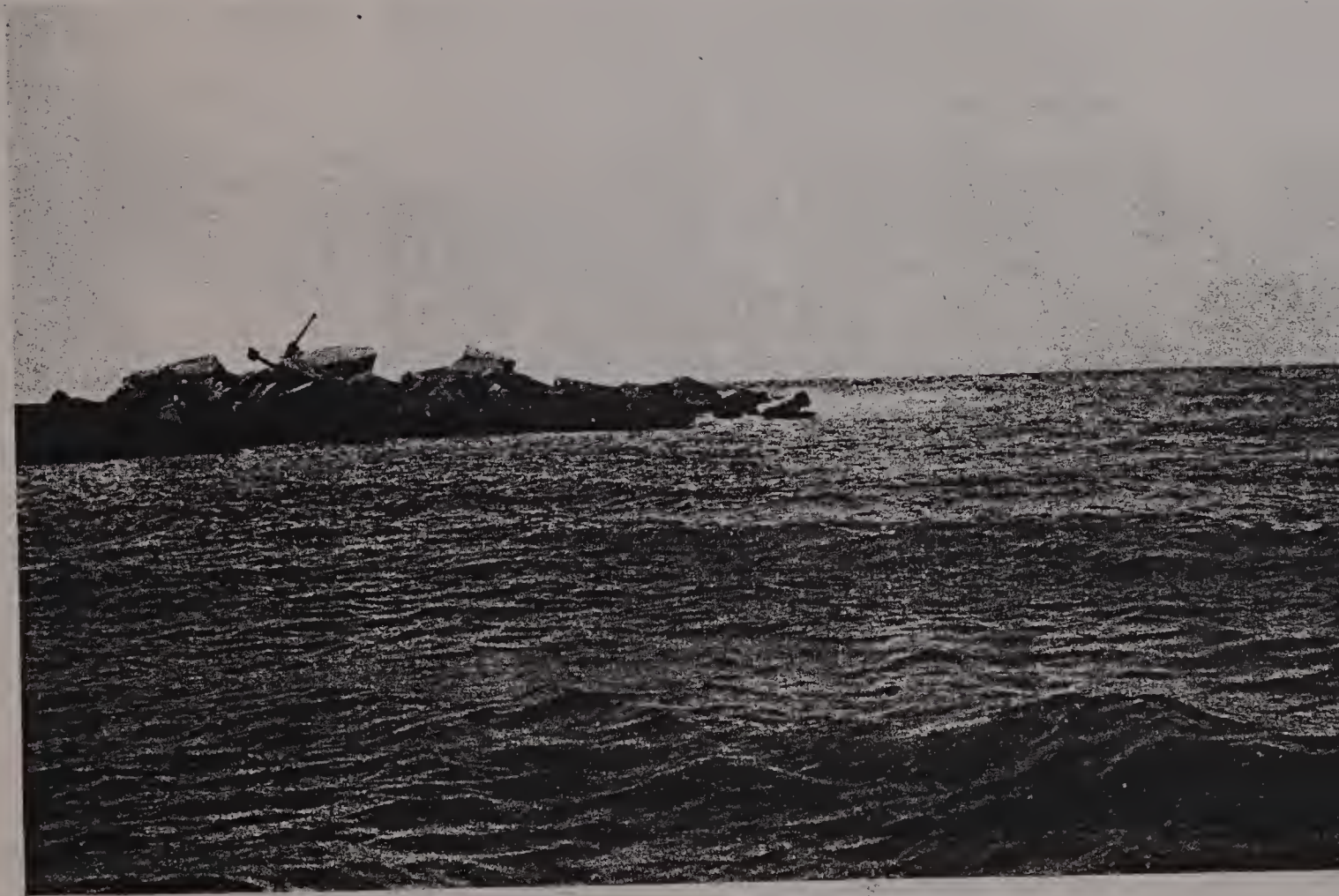
Outer End of Breakwater, Sept. 2, 1910.
