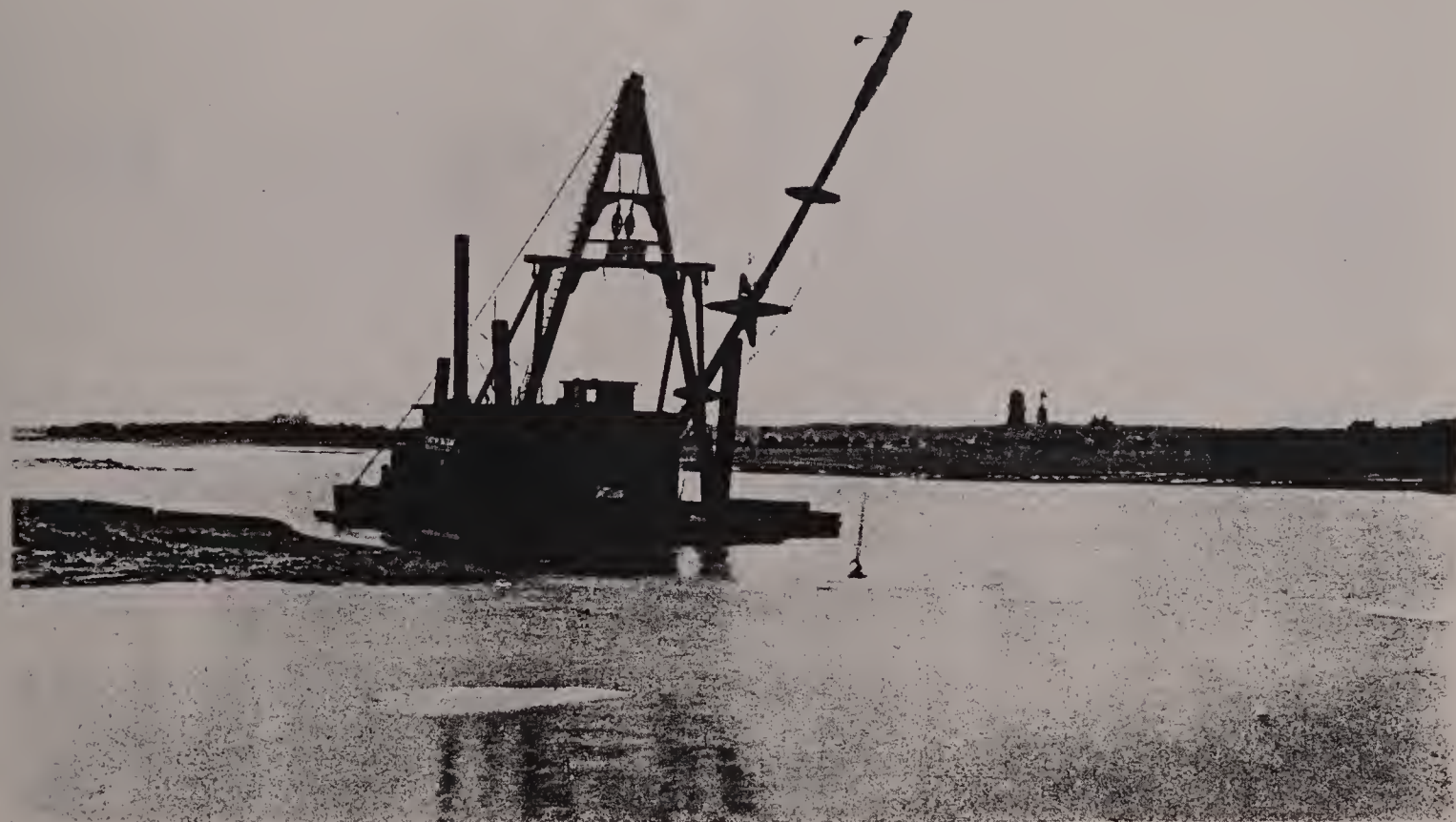
Deepening Channel on Buzzards Bay End of Canal to Admit Big Dredges.
