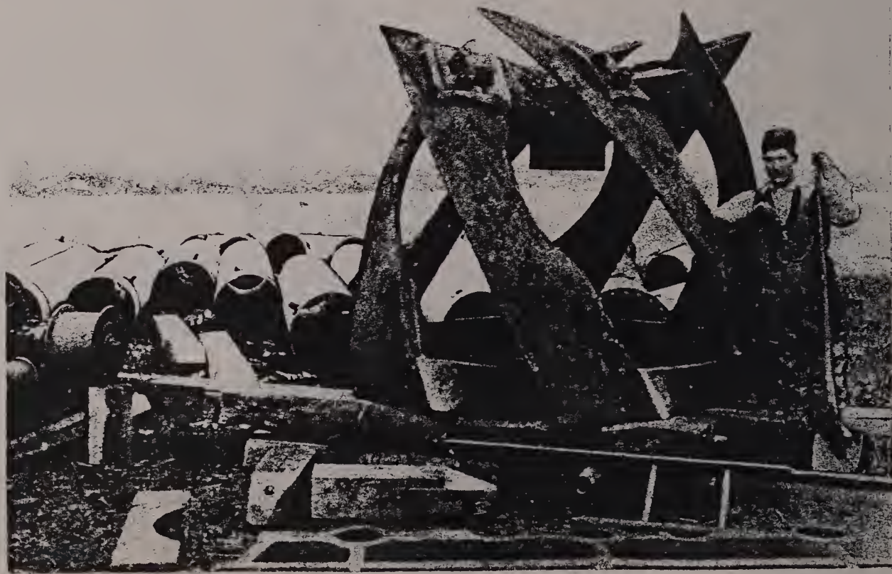
Giant Cutter of Dredge General Mackenzie.
