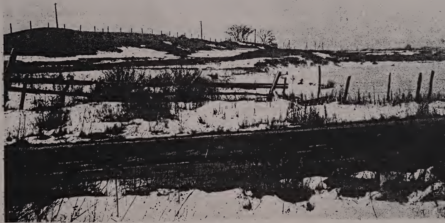
Where 500-Italians Began Work of Digging Canal With Wheelbarrows in Sandwich, near Town Neck in 1880.
