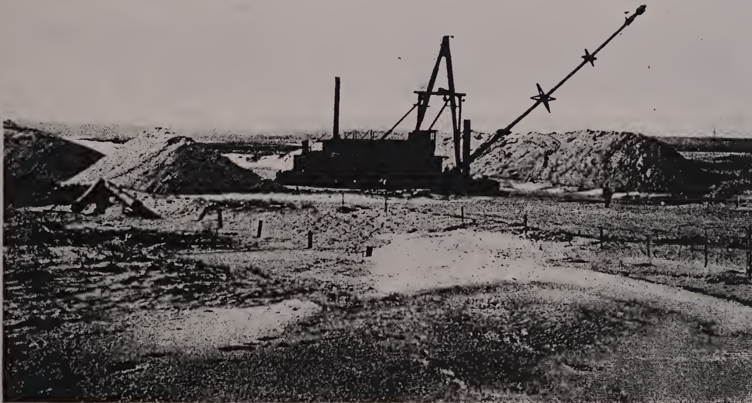
Dredge Nahant Finishing the Work of Cutting a Channel Through the Beach, Cape Cod Bay, Feb. 1910.
