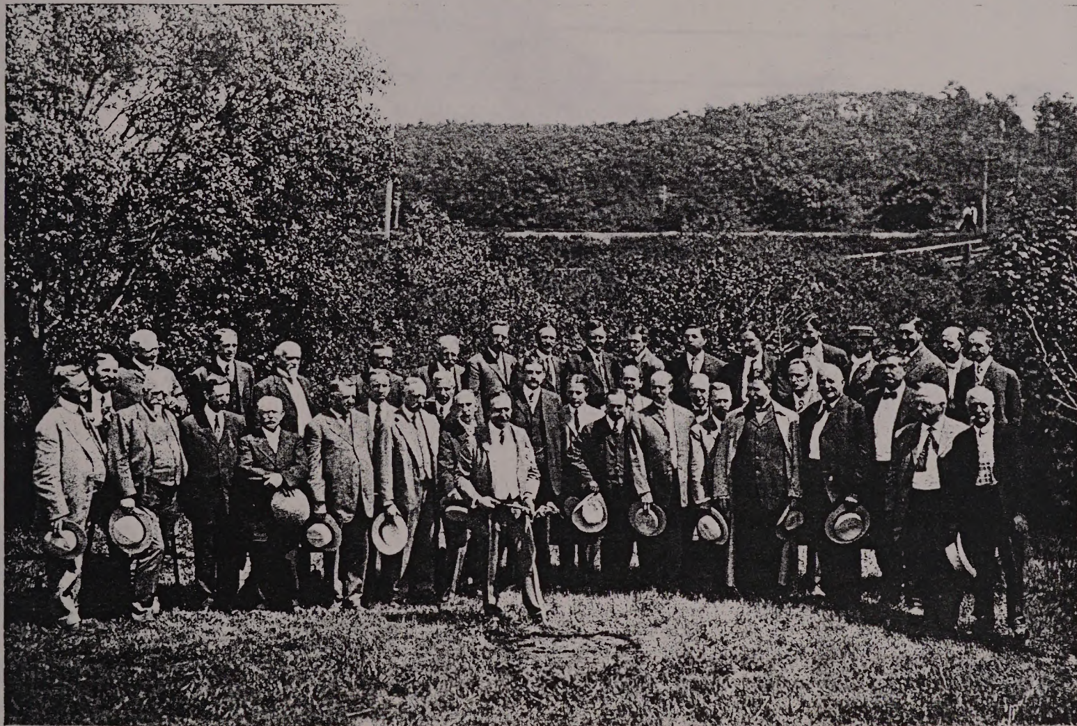
August Belmont Digging the First Shovelful of Earth on Line of the Canal at Bournedale June 21, 1909.
