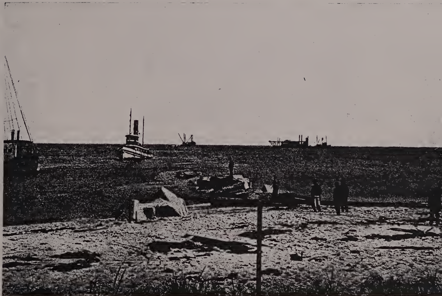
Building the Breakwater from the Shore End, 1909. Dredge General Mackenzie in Tow of Tug on the Way to Dig Through the Beach.
