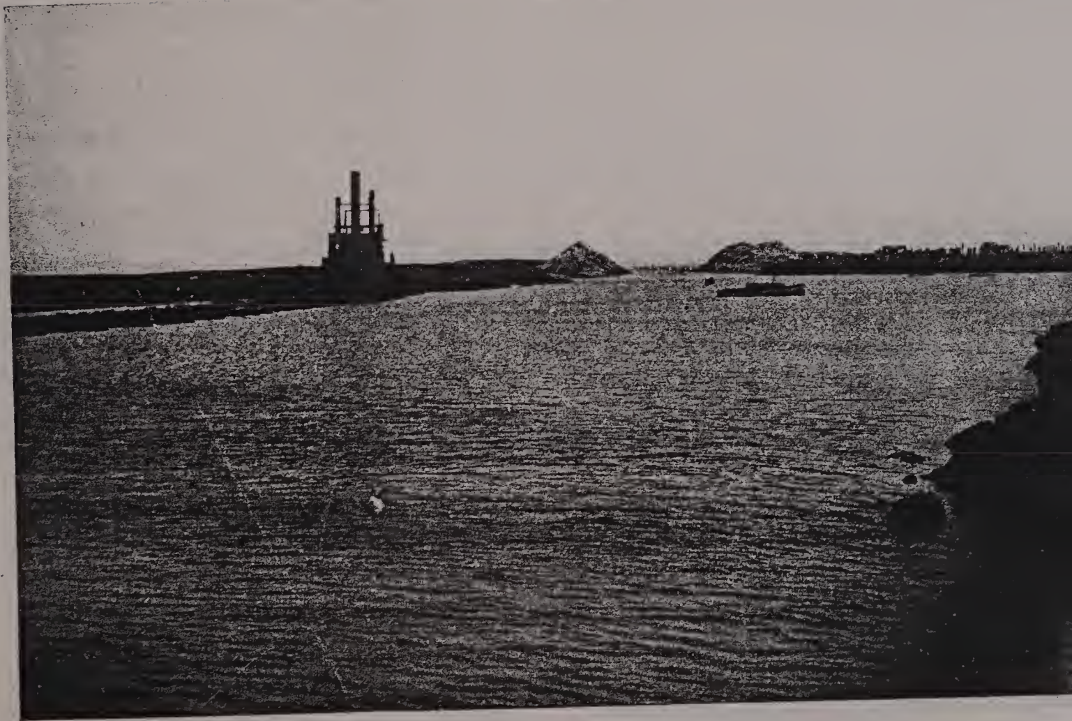
General View of the Canal Looking Towards Cape Cod Bay Before the Sand Hills at the Entrance Were Removed July 1
