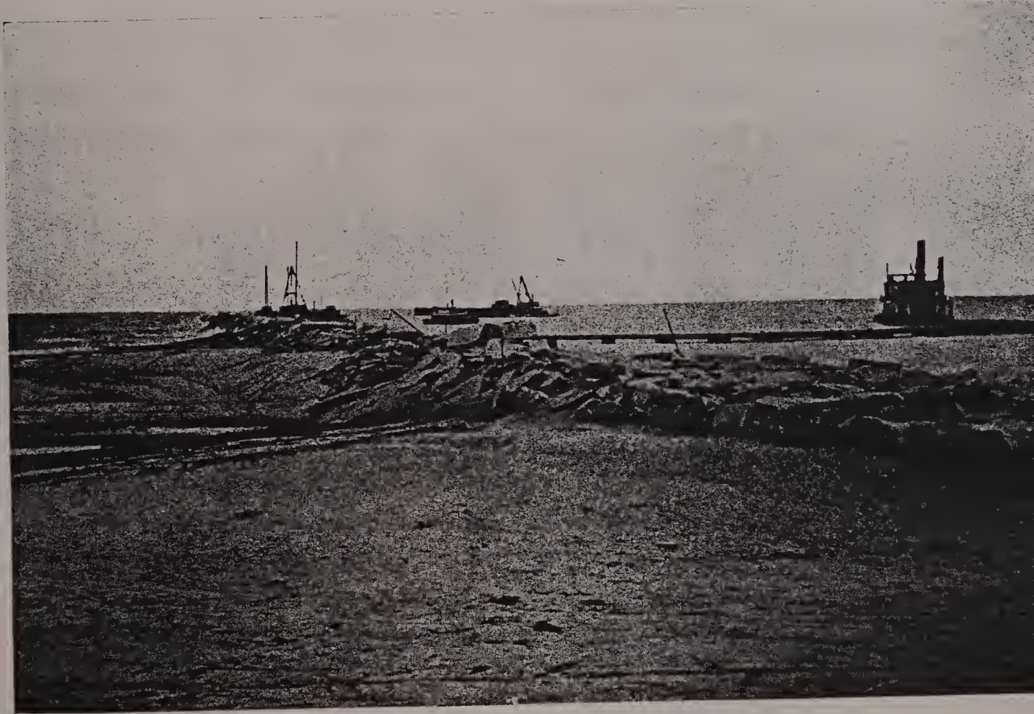
Dredge General Mackenzie Dredging Channel and Sending Material Over Breakwater, Sept. 1910.
