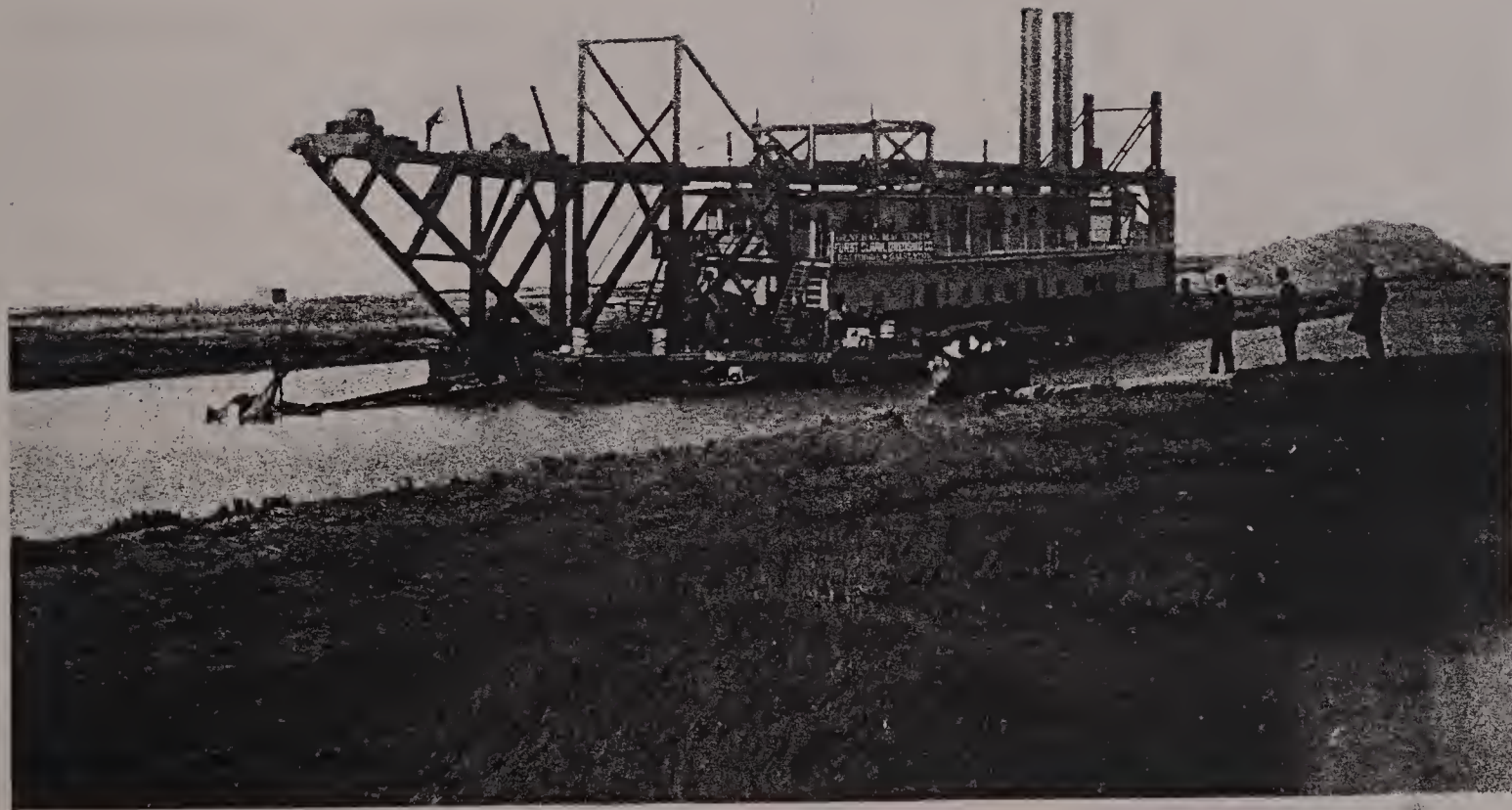
General Mackenzie Inside the Beach Ready To Begin Work of Digging the Canal, April 10, 1910.
