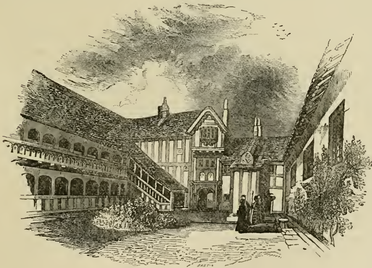
Leicester's Hospital, Warwick.
