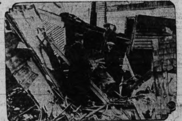
YES—WINTER'S HERE —A leaky gas range—a lighted match—blow! And that's what every Winter brings. Photo shows graphically what happened to a house in Scranton, Pa., where leaking gas and lighted match came in contact.
