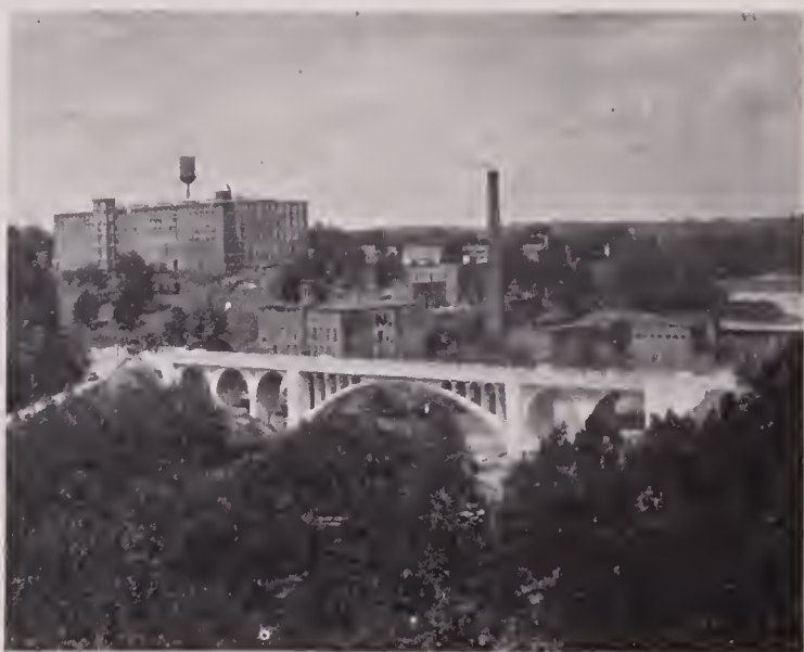
BRIDGE OVER PACOLET RIVER AT CONVERSE (Hurricane Shoals)
