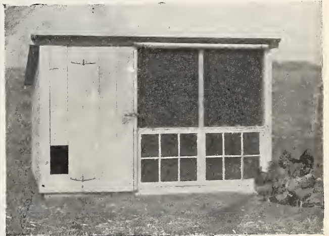
D. W. Rich small shed-roofed colony pattern open-front house.
