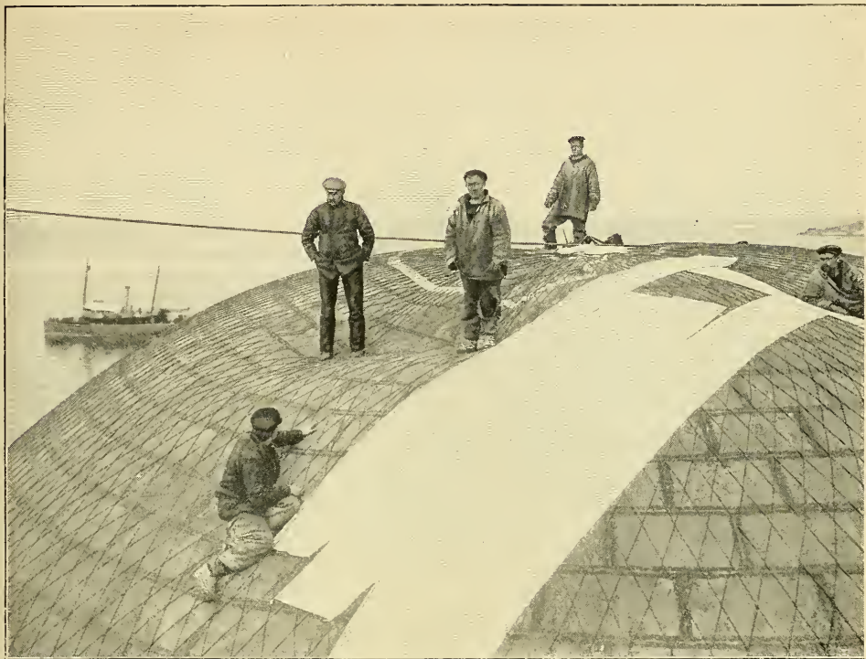
EXAMINING THE BALLOON FOR LEAKS.
