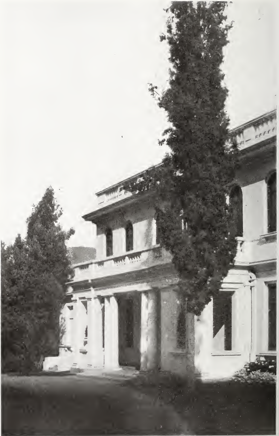
HOUSE OF DR. ADALBERT FENYES, PASADENA, CALIFORNIA. Robert D. Farquhar, Architect.
