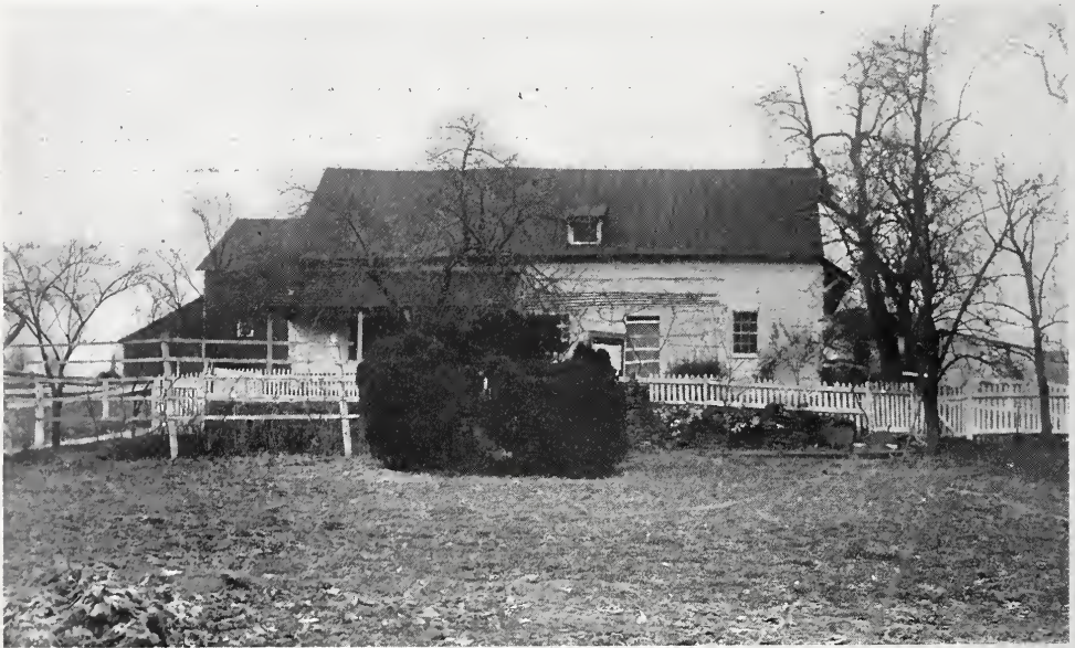
AN 18TH CENTURY HOUSE—THE WALLS ARE OF LOGS WITH A COURSE OF STONE LAID OVER THE TOPS OF THE WINDOWS AND THE WHOLE WHITWASHED.
