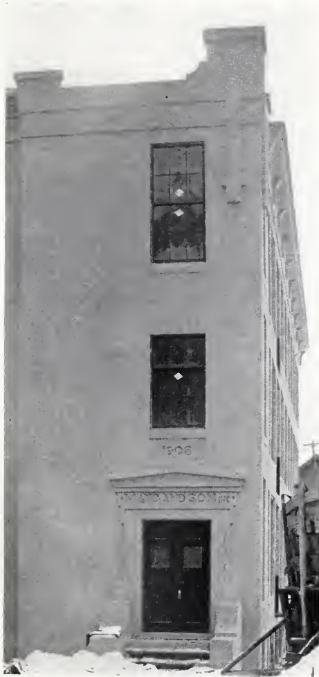
FIG. 6. SKILFUL TREATMENT OF A CONCRETE CORNICE.
