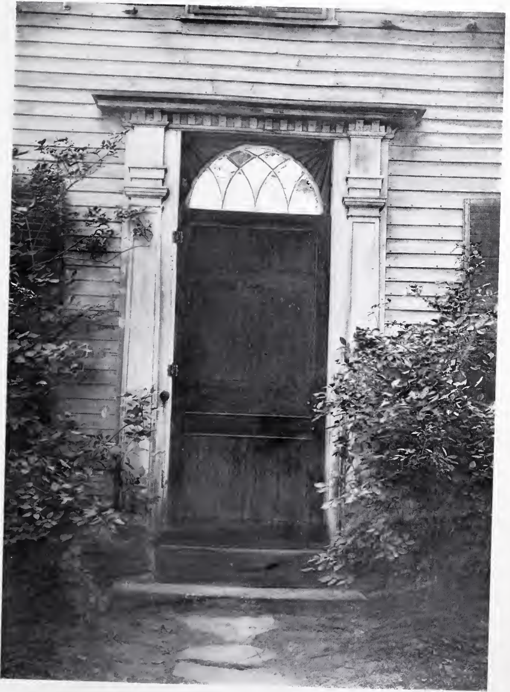
A 1770 entrance in Deerfield. The very extenuated doorway would appear less so if the spandrels over the arch had been painted white instead of dark, as no doubt they were originally. It is interesting to note that even in this unpretentious doorway, the pilasters have a most subtle entasis.
