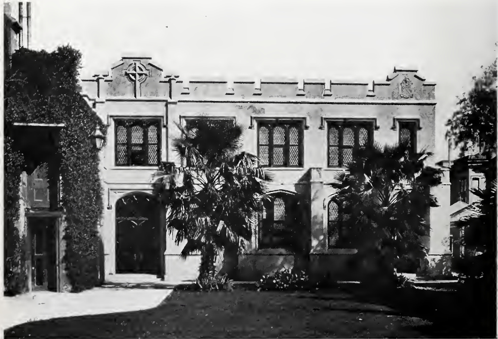
HOWCOTT MEMORIAL—TRINITY PARISH HOUSE.
