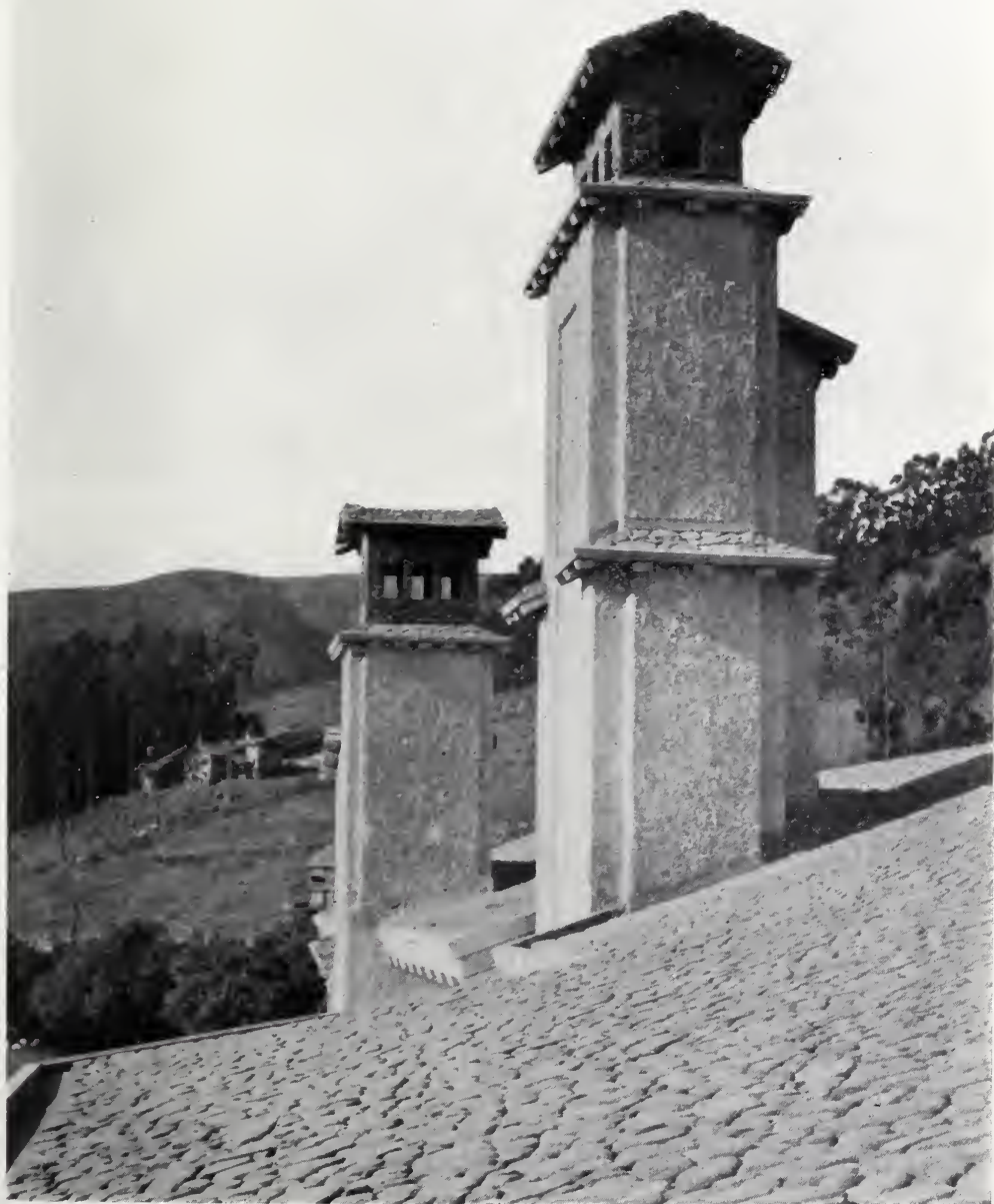
CHIMNEY DETAIL—RESIDENCE OF HENRY W. TAYLOR, ESQ., CLAREMONT PARK, BERKELEY, CAL. LOUIS C. MULLGARDT, ARCHITECT.
