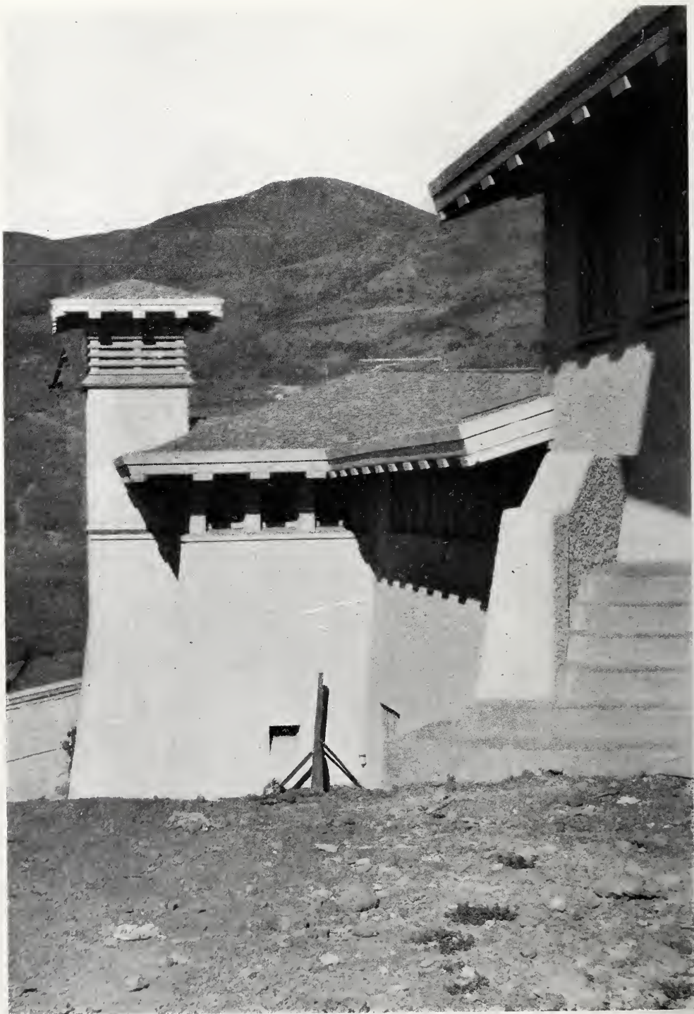
DETAIL—RESIDENCE OF HENRY W. TAYLOR, ESQ., CLAREMONT PARK, BERKELEY, CAL. LOUIS C. MULLGARDT, ARCHITECT.
