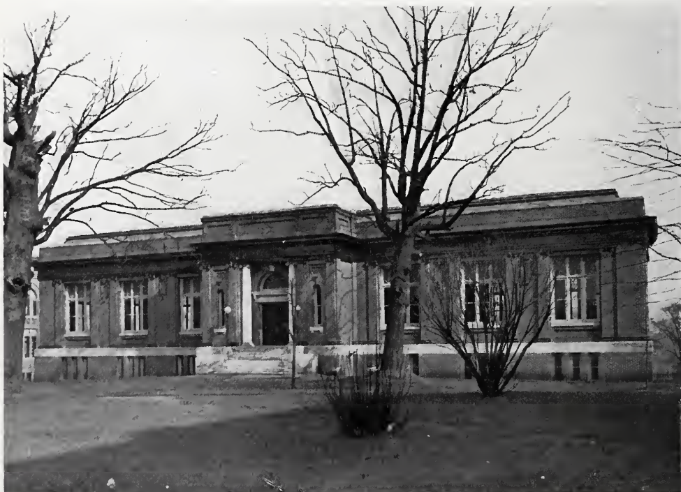
PEABODY LIBRARY BUILDING—UNIVERSITY OF GEORGIA (1903). Athens, Ga. Haralson Bleckley, Architect.
