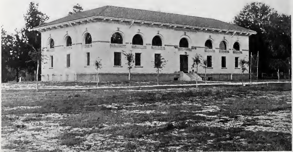
LIBRARY AND ADMINISTRATION BUILDING—ROLLINS COLLEGE.
