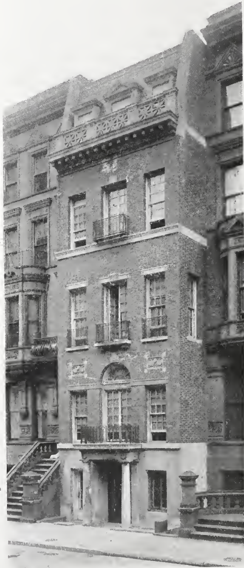
FIG. 14.—NO. 26 EAST 76TH STREET. Chas. E. Birge, Architect.
