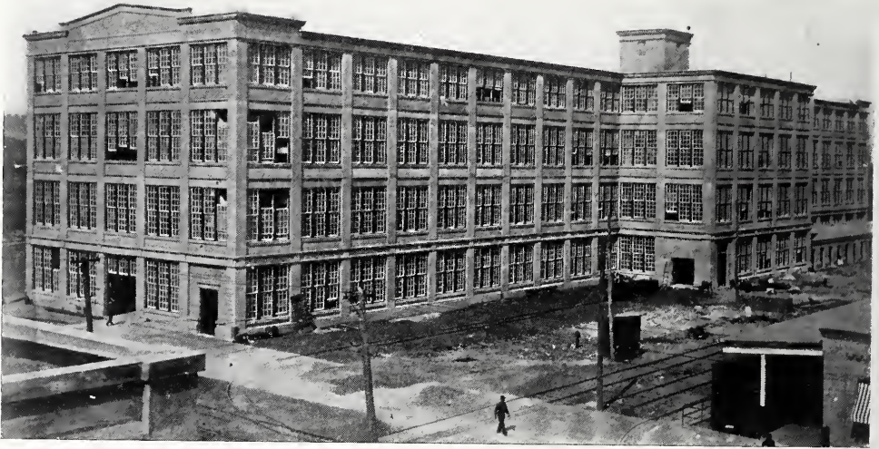
FIG. 4. A REINFORCED CONCRETE FACTORY BUILDING.
