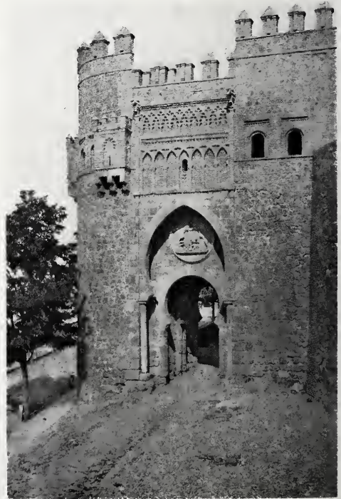
The Gate of the Sun, with Roman and Spanish Stone Work, Mudéjar Brick Work, and Visigothic Columns.
