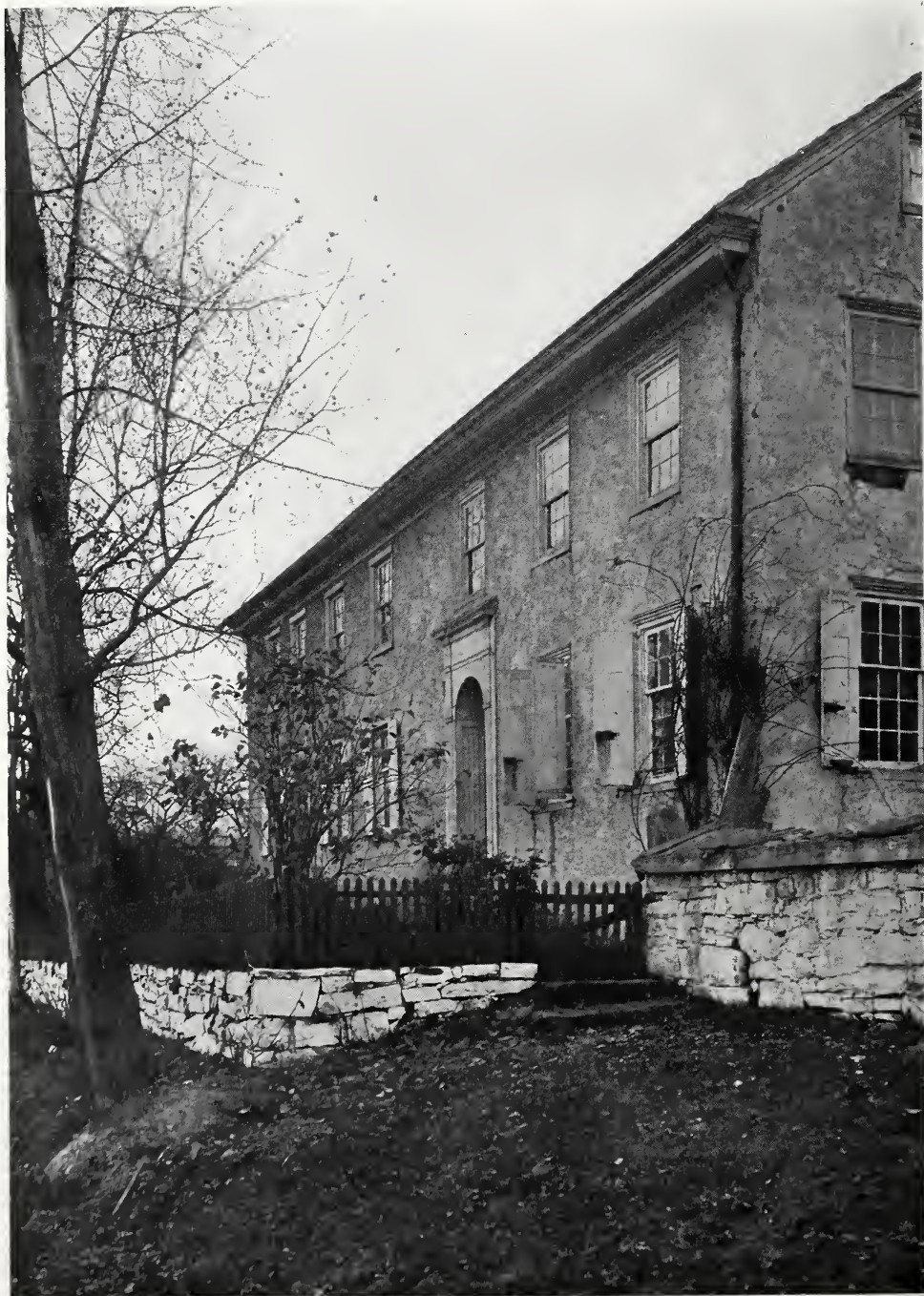
DETAIL OF MAIN DOORWAY AND FRONT OF STUCCO-COVERED STONE HOUSE BEYOND GLASGOW—MOST OF THESE HOUSES, EACH ABOUT 130 YEARS OLD HAS A DELICATELY COVERED WOOD CORNICE IN GOOD CONDITION.
