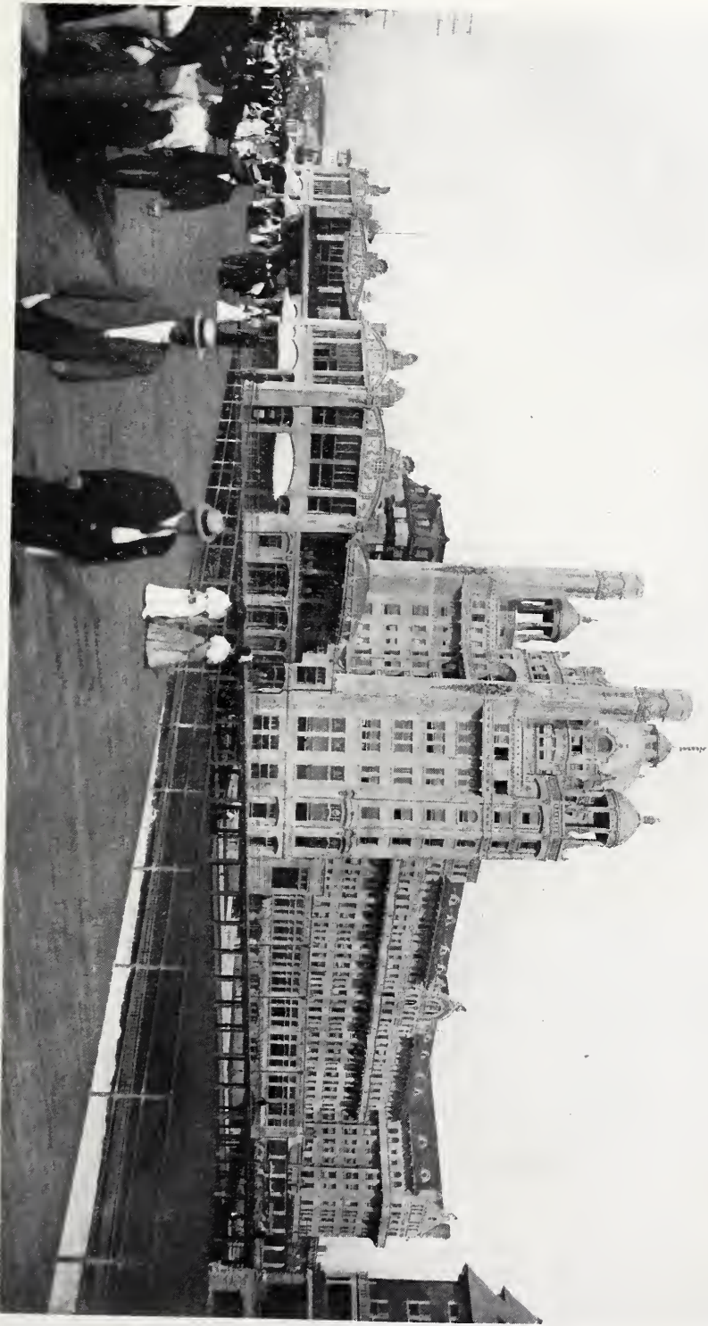
FIG. 12—THE MARLBOROUGH-BLENHEIM HOTEL, ATLANTIC CITY, N. J.—CONCRETE DECORATED WITH INLAID COLORED TILES.
