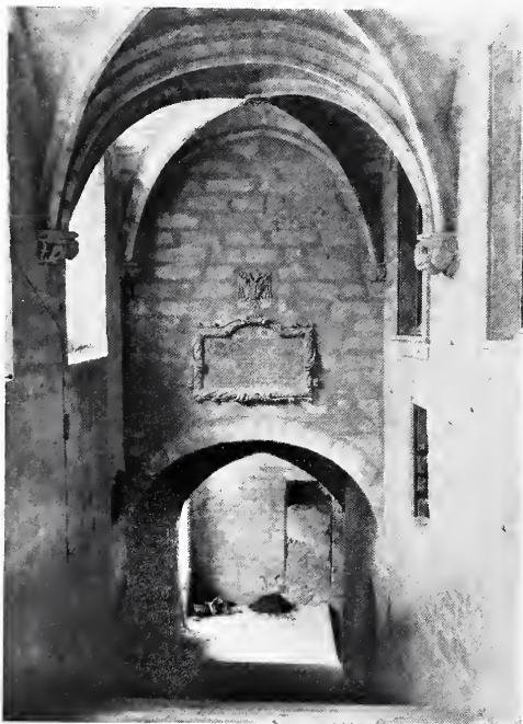
STAIRCASE LEADING TO THE PONTIFICAL CHAPEL OF CLEMENT VII—RESTORED IN 1859.
