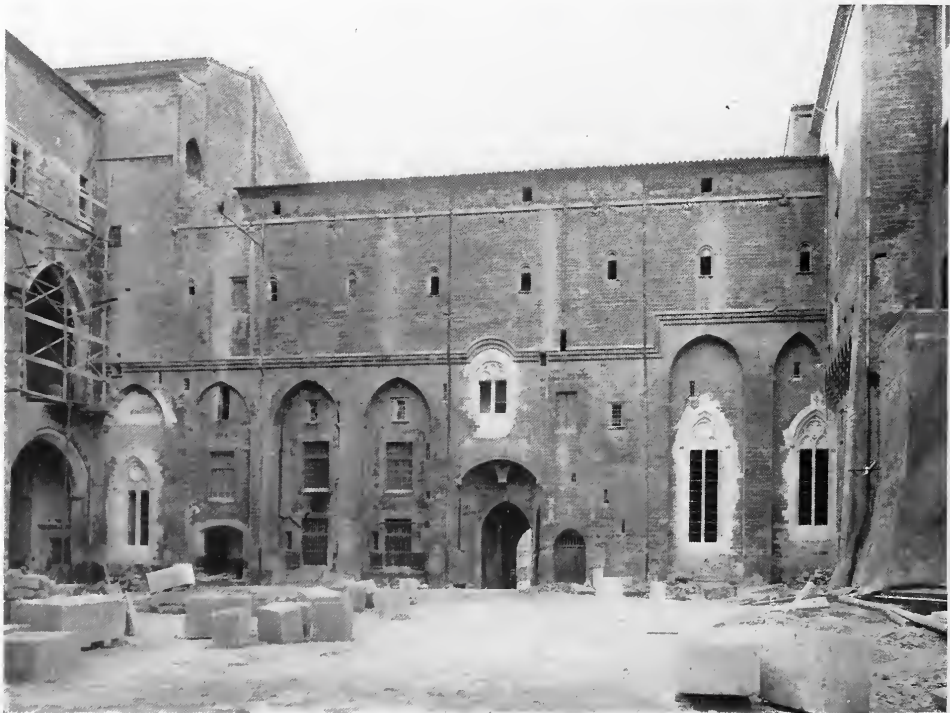
WESTERN FAÇADE FACING COURTYARD.
