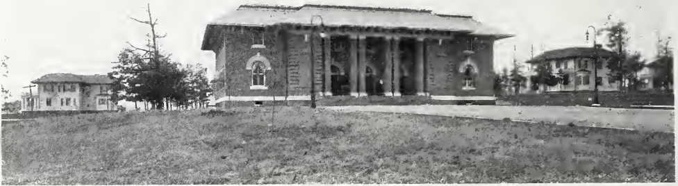
The Administration Building.
