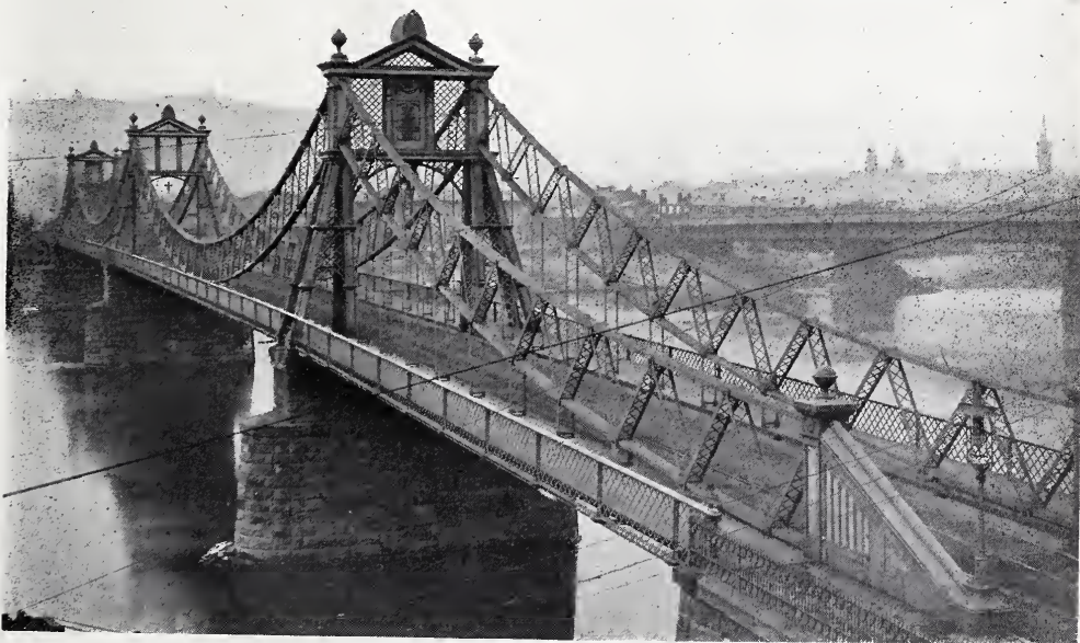
THE SEVENTH STREET BRIDGE, PITTSBURGH, PA. Gustav Lindenthal, Engineer.
