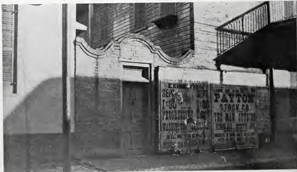
A COURTYARD ENTRANCE.
