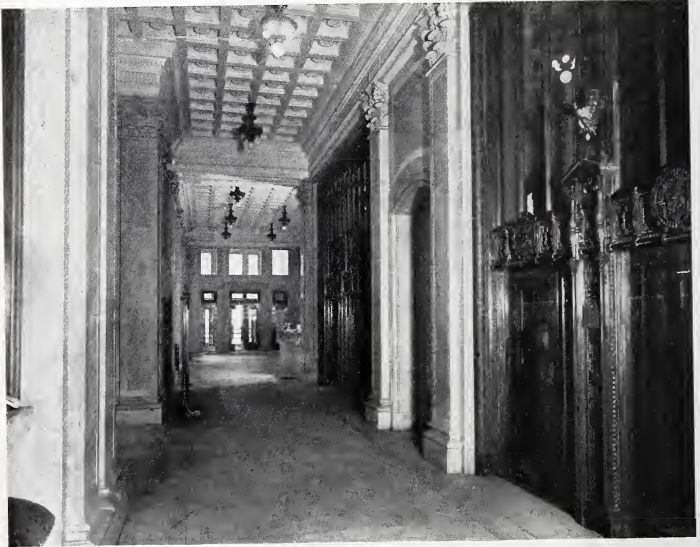
ELEVATOR LOBBY, LOOKING TOWARDS ENTRANCE—THE WHITNEY CENTRAL NATIONAL BANK BUILDING.
