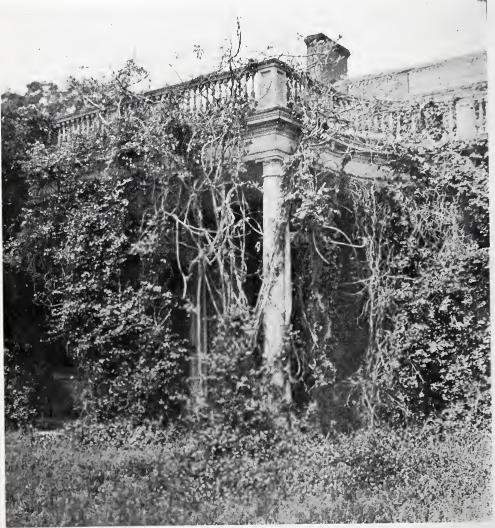
PORCH DETAIL, "MONTEBELLO." BALTIMORE, MARYLAND.
