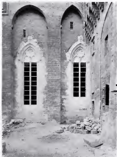
RESTORED WINDOWS TO THE RIGHT OF THE ENTRANCE IN THE COURTYARD.
