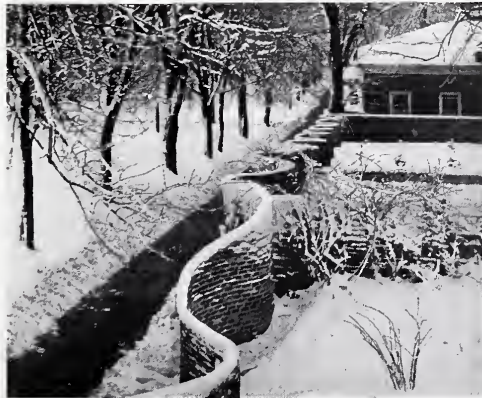
JEFFERSON'S FOUR-INCH BRICK FENCE.
