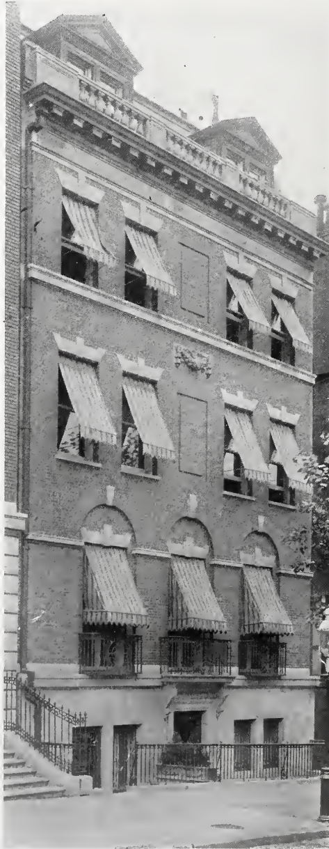
FIG. 9.—754 PARK AVENUE. Geo. H. De Gersdorff, Architect.
