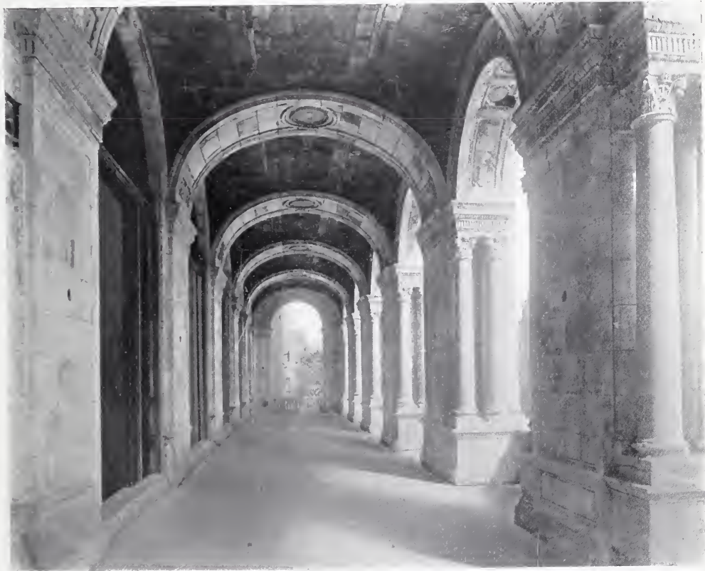
LOGGIA DETAIL—THE HERMITAGE HOTEL.
