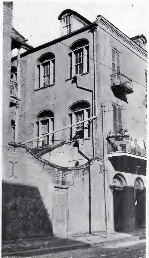
A COURTYARD ENTRANCE
