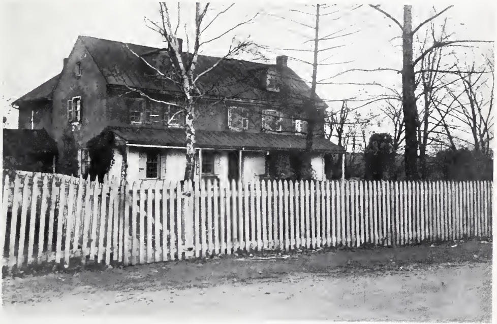
A HOUSE NEAR POTTSTOWN, PA., BEARING DATE 1804.
