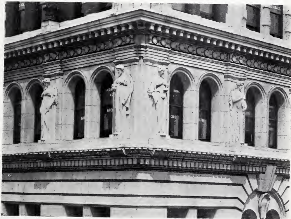
DETAIL OF THIRD STORY—FARMERS' BANK BUILDING.
