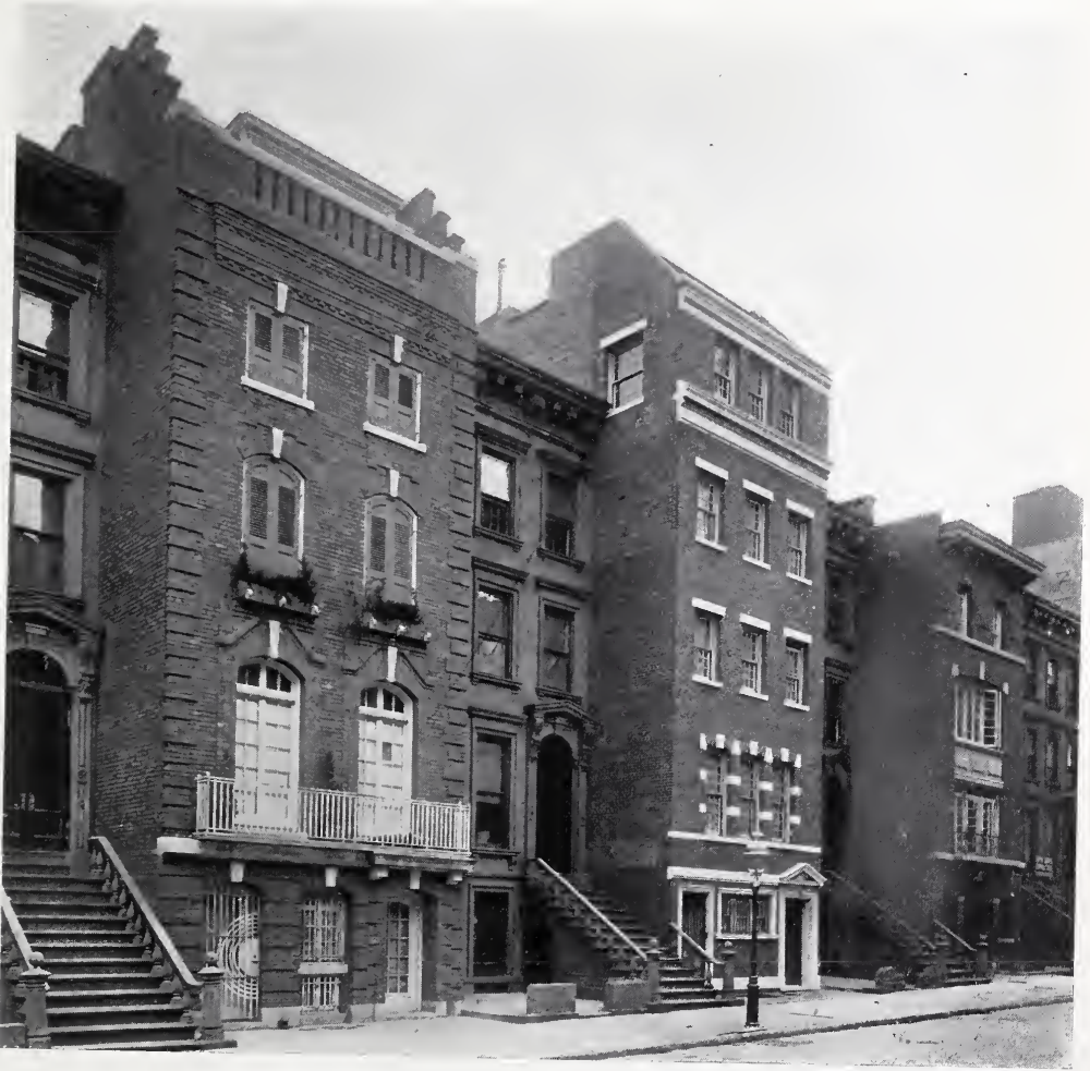
FIG. 13.—NOS. 122-126-130 EAST 80TH STREET. Schwartz & Gross, Architect.
