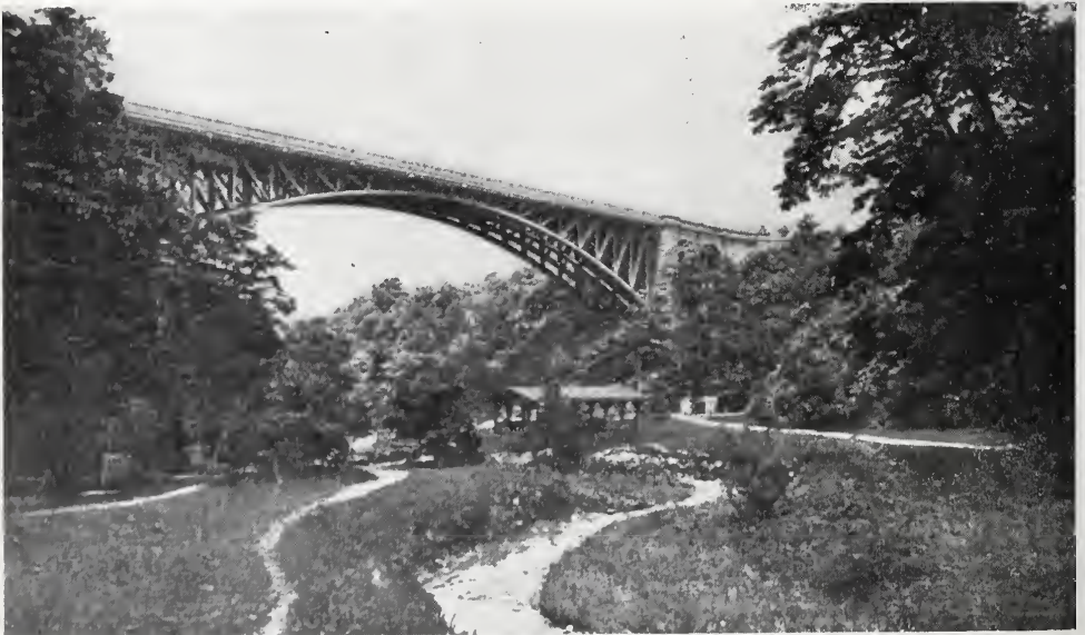
THE PANTHER HOLLOW BRIDGE.
