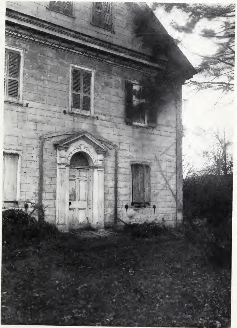
DOORWAY OF A WOODEN HOUSE NEAR DOUGLASVILLE, PA., ALMOST FALLEN TO DECAY—THE WOODEN WALLS WERE BUILT IN THE MANNER OF CUT-STONE WORK—THE REMAINS OF AN ARBOR ARE STILL SEEN AROUND DOORWAY.
