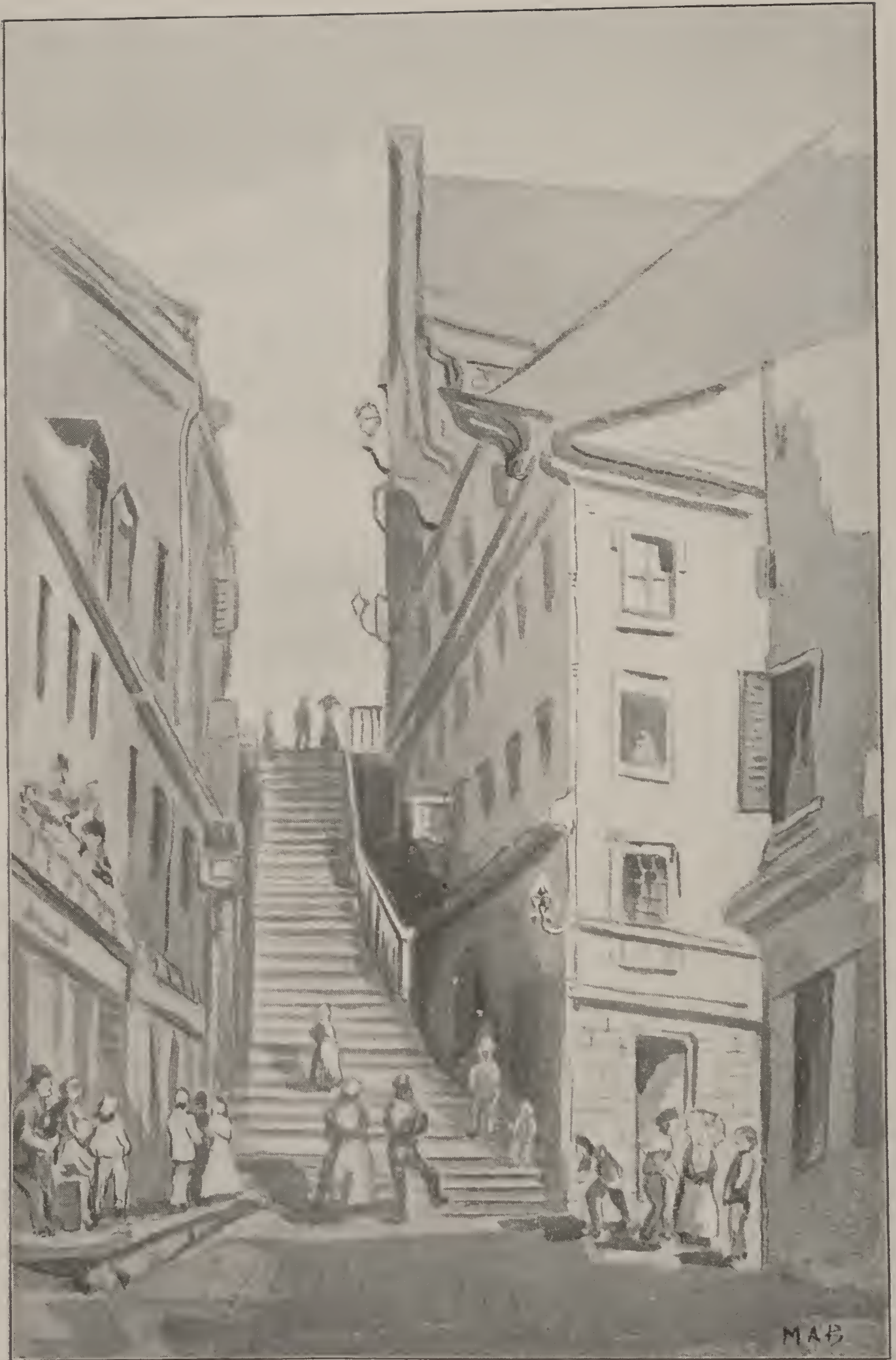
"BREAKNECK" STAIRS, CITY OF QUEBEC
