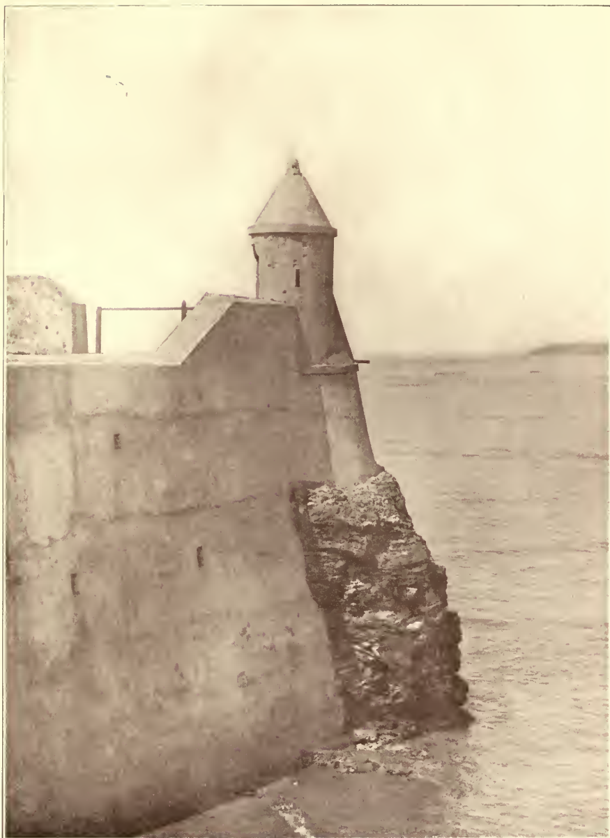
A "look out" tower on the city walls looking on the Pacific.
