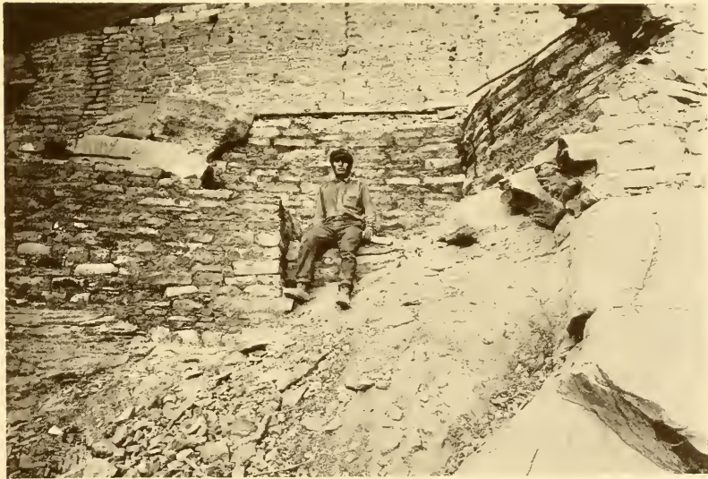
FIG. 121.—New foundation of Tower from in front. All masonry below dark lines is portion of repair work.
