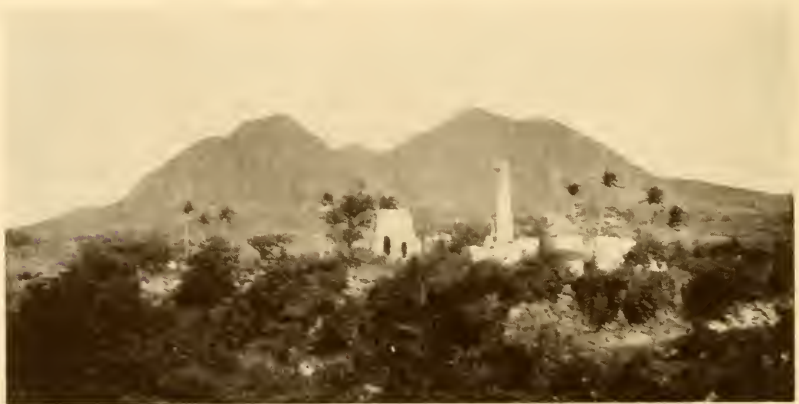
FIG. 45.—Ruined sugar mill, Montserrat. Ruined windmills—abandoned in favor of modern machinery—are as characteristic of the Lesser Antillean landscape as the old watch towers are of that of the Mediterranean coast of Europe.
