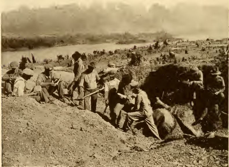
FIG. 117.—Excavators at work on shell mound at mouth of Town Creek, near Muscle Shoals, Colbert County, Alabama.
