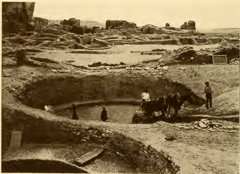
FIG. 100.—Excavating one of the major kivas of Pueblo Bonito. The flat roof of the subterranean room, 44 feet in diameter, had been supported by four wooden pillars. (Photograph by O. C. Havens. Courtesy of the National Geographic Society.)
