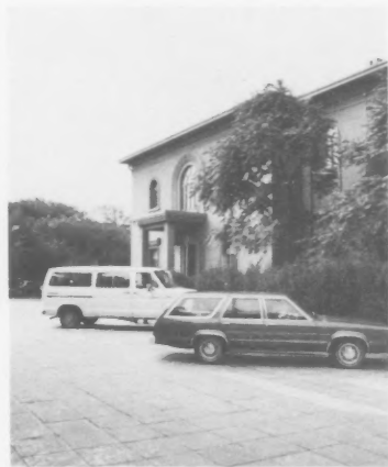
The Bruce Building, also known as Erban, or Embassy Compound No. 2.
