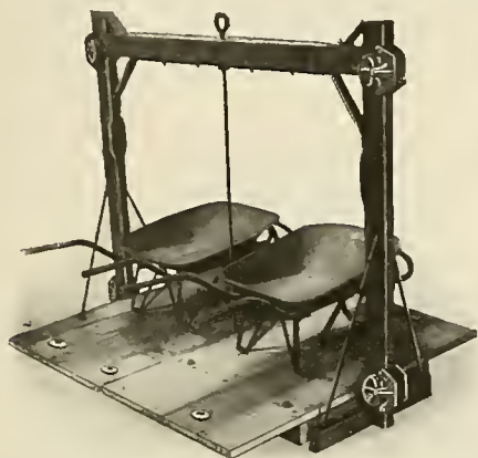
Elevator Rigged for Wheelbarrows
