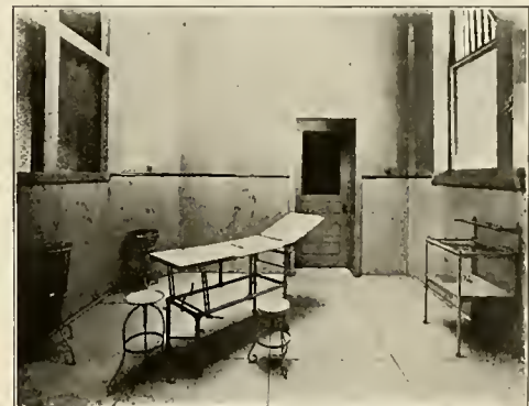
OPERATING ROOM, NEW ORLEANS SANITARIUM Walls, Floor and Sanitary Base of "Novus" Glass Toledano & Wogan, Architects, New Orleans, La.
