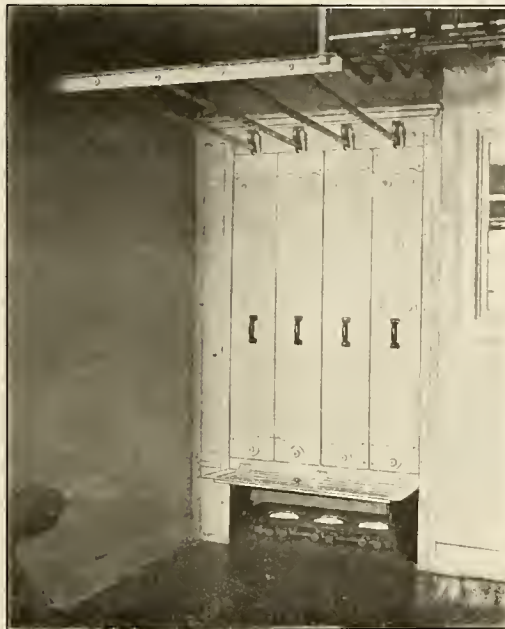
FIG. 3. DRYER HEATED BY GAS DIRECT So Arranged with Deflecting Pan, etc., that all Odors and Impurities do not come in Contact with Clothes
