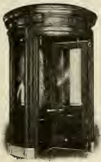
U. S. P. O., ELKHART, IND. Walls, ceiling and wings of quartered oak, special hardware; marble bases. Sliding doors on exterior.
