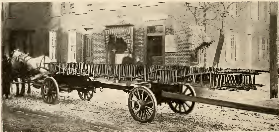
FIG. 4. GIRDER FRAMES Ranging from 20 to 30 feet long, delivered as a "Unit" (PATENTED)
