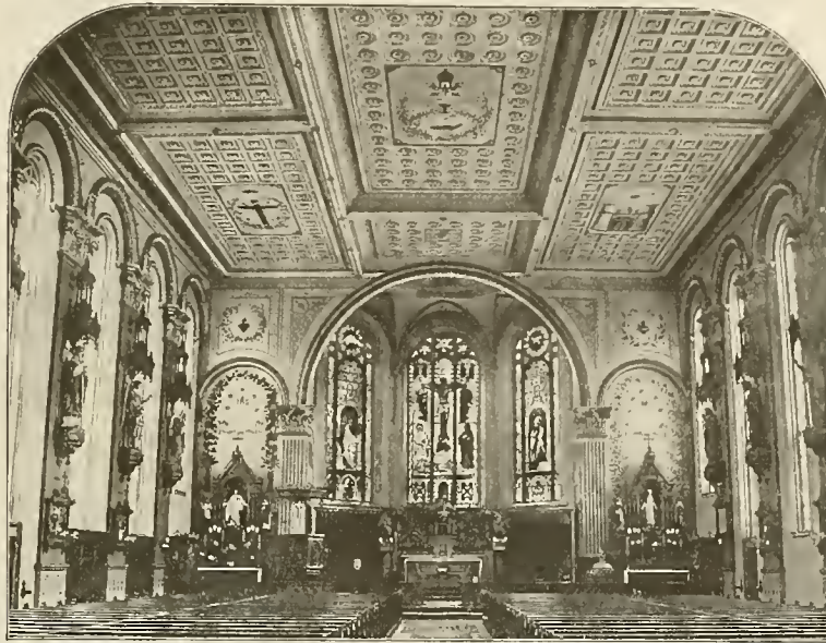
Interior of SS. Peter and Paul's Church, Rochester, N. Y. "WHEELING CEILINGS" used, Designs No. 1203 and No. 1244. Designs suitable for rooms of any size or style.
