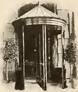
WALDORF-ASTORIA HOTEL, NEW YORK CITY Walls, ceiling and wings are of mahogany, conical roof of metal.
