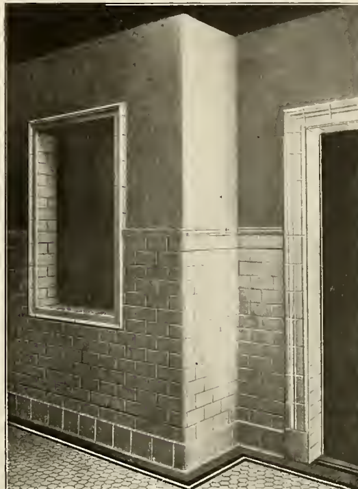
APPLICATION OF BATH ROOM TILE
