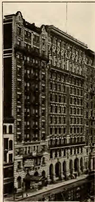
BUILDINGS Nos. 3 to 15 EAST 27th STREET, NEW YORK CITY In which our Material is Installed
