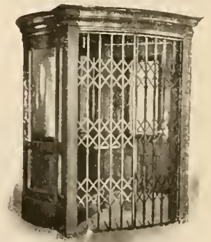
PHILLIPSBURG BUILDING, YONKERS, N. Y. Walls, ceiling and wings of quartered oak, folding gates for locking purposes, fold in pockets adjoining jambs of curved walls.
