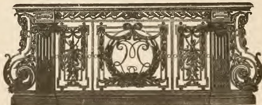
ONE OF THE ORNAMENTAL CAST AND WROUGHT IRON RAILS BETWEEN STAIRWAY ARCHES ON FIRST FLOOR. Minnesota State Capitol, St. Paul, Minn. Cass Gilbert, Architect
