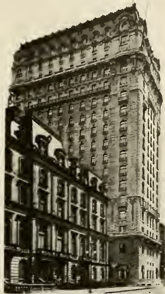
ST. REGIS HOTEL, NEW YORK Mason Work, Engineering and Steel Skeleton only, done by this Company
