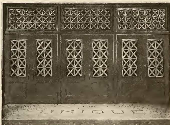
COPPER ENTRANCE DOORS, UNIQUE THEATRE, MINNEAPOLIS Bertrand & Chamberlain, Architects
