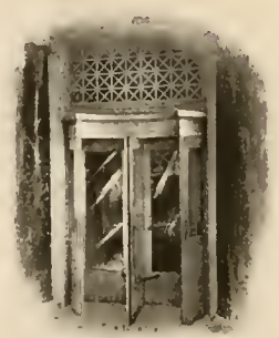
KNICKERBOCKER TRUST CO. NEW YORK CITY Walls, ceiling and wings of Enuphyll bronze construction finished in color to harmonize with all other work.
