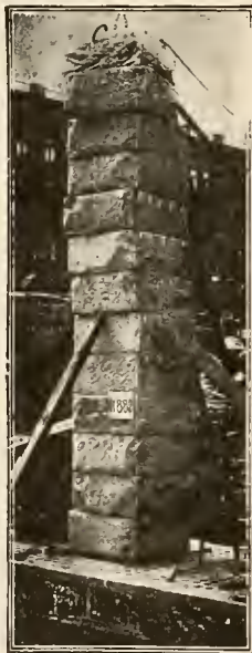
Official tests made by Engineers of N. Y. Rapid Transit Commission. Load of 11882 pounds concentrated in centre of slab 4' 2" x 5' 0".
