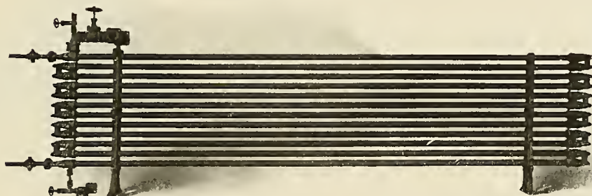
DOUBLE PIPE COUNTER-CURRENT AMMONIA CONDENSER
