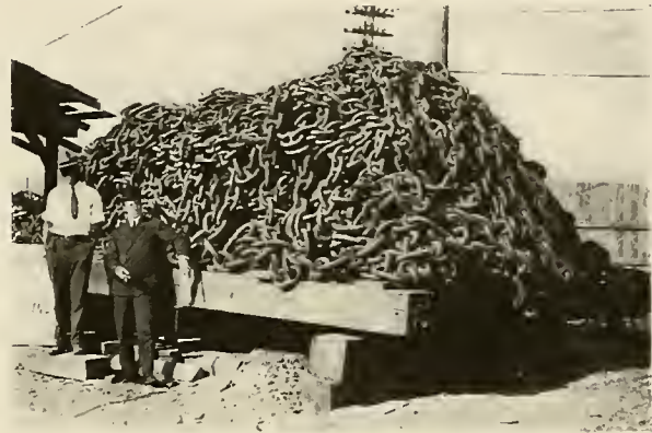
FIG. 6. RAYMOND CONCRETE PILE Test Made at Annapolis, Md. 133,270 lbs., no settlement.
