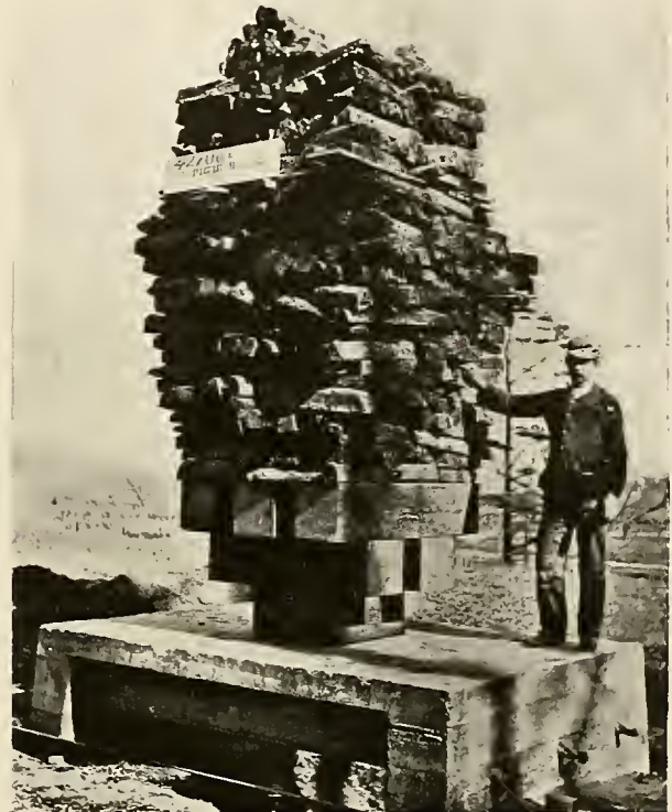
TESTING MCKEAN ST. CONCRETE SEWER, PHILADELPHIA, PA. 2200 Feet Built with Whitehall Portland Cement according to the Ransome System, by the Ransome Construction Co., Philadelphia.
