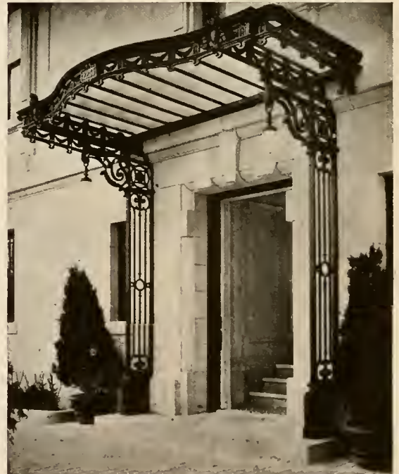
WROUGHT AND CAST-IRON MARQUISE Chas. L. Fitzhugh's Residence, Washington, D. C. Wood, Donn & Deming, Architects
