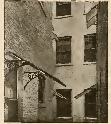
FIG. 7. COURT OF FLAT BUILDING WITH PRISM CANOPIES OVER WINDOWS
