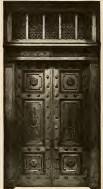
BRONZE DOORS, TRANSOM AND CASING Northwestern National Bank, Minneapolis, Minn. Kees & Colburn, Architects
