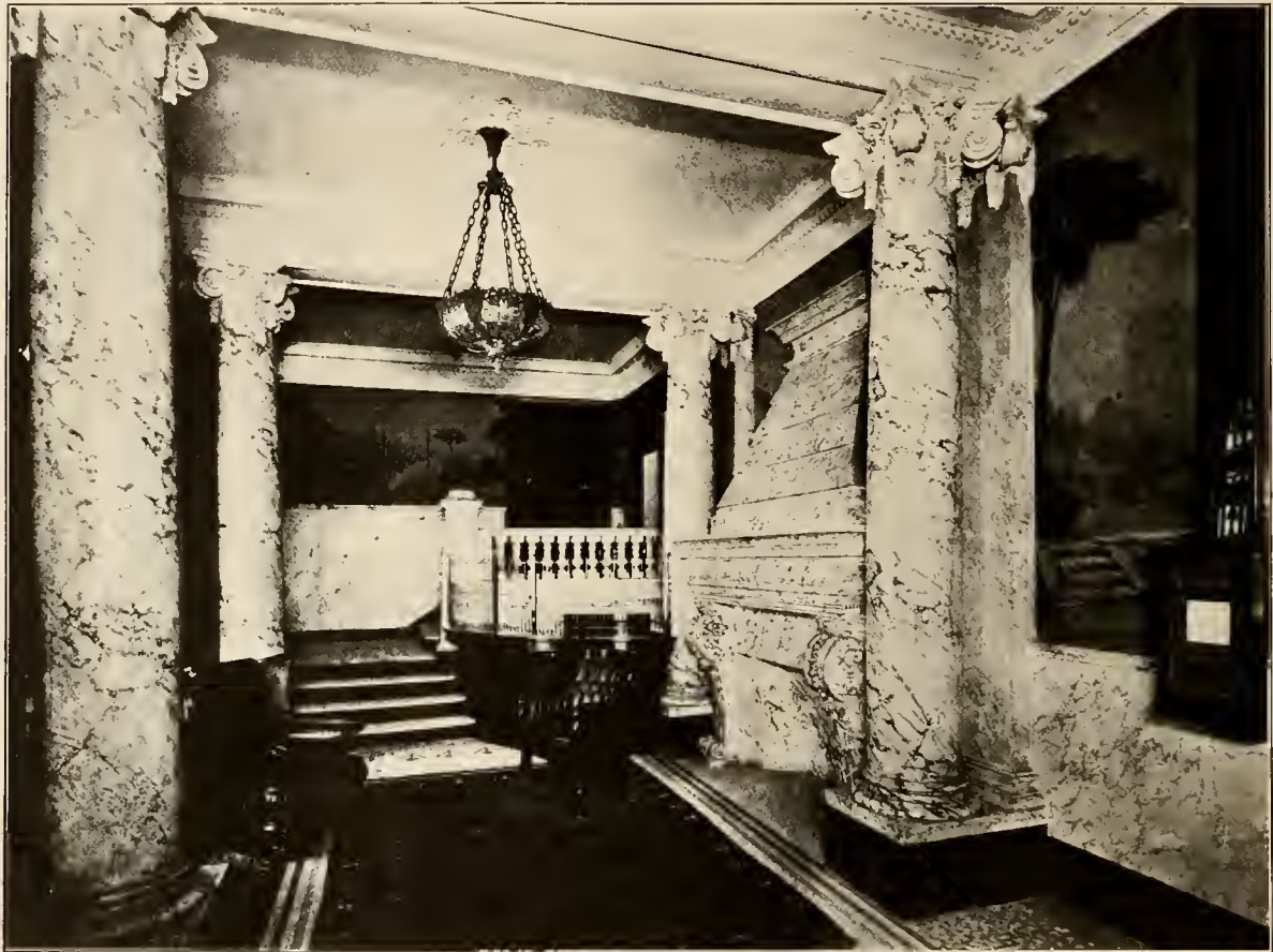
A CORNER IN THE MAIN HALL OF THE SCHUYLER ARMS HOTEL, NEW YORK CITY, N. Y. Artificial Pavonazzo Marble Columns, Pilasters, Mantels, Wainscoting, Newel-Posts and Balustrade executed by us
