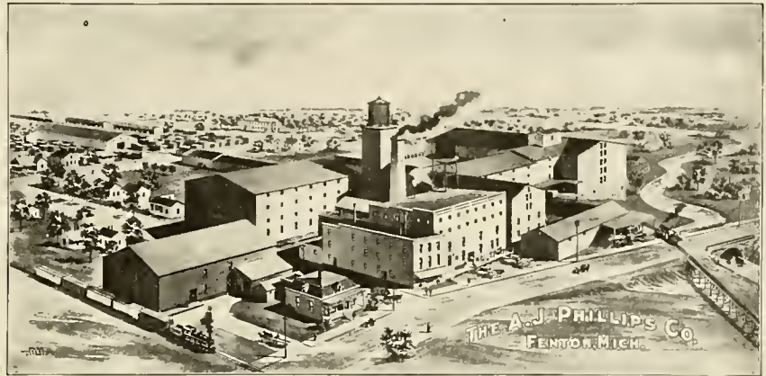
GROUNDS AND FACTORY OF THE A. J. PHILLIPS CO., FENTON, MICH.
