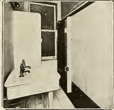
TOILET ROOM IN BELLEFIELD DWELLINGS, PITTSBURG, PA. Walls, Floors and Partitions of "Novus" Glass Carlton Strong, New York, Architect
