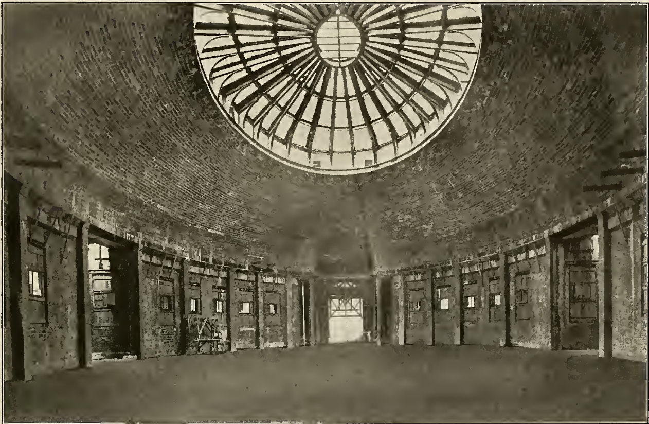
ELLIPTICAL RODUNTA DOME, 130 Ft. by 75 Ft. SPAN, NEW YORK CUSTOM HOUSE Cass Gilbert, Architect
