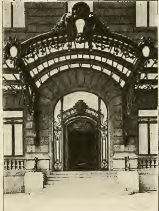
BRONZE MARQUISE, HOTEL ST. REGIS, NEW YORK TROWBRIDGE & LIVINGSTON, Architects
