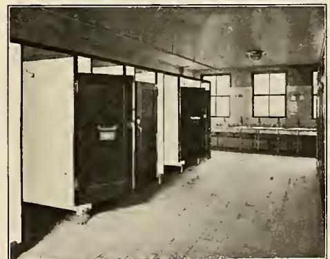
LADIES' TOILET ROOM, JOSEPH HORNE CO., DEPARTMENT STORE, PITTSBURG, PA. Walls, Floor and Partitions of "Novus" Glass Struthers & Hannah, Architects
