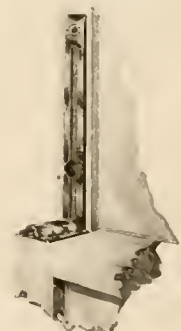
FIG. 4. WINDOW VENTILATING LOCK Patented May 23d, 1905
