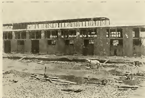
FIG. 3 SECTION OF CAR SHOPS D. L. & W. R. R. UNDER CONSTRUCTION
