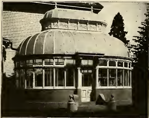
FIG. 5. PALM HOUSE, U BAR CONSTRUCTION
