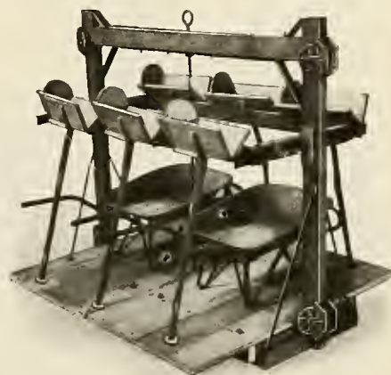
Elevator Rigged for both Hods and Wheelbarrows
