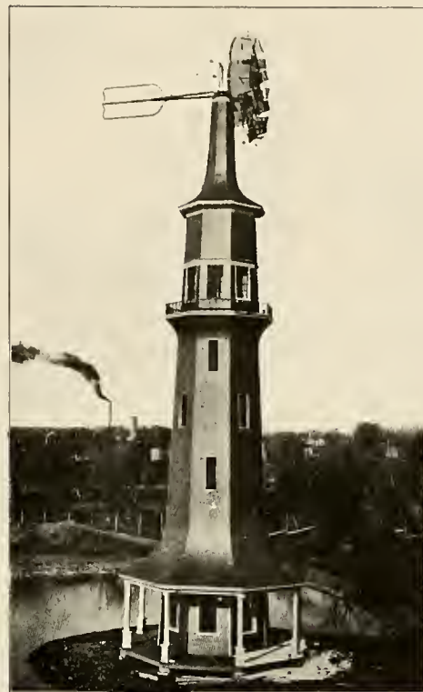
HALLADAY WINDMILL 20 feet in diam.; 90-foot steel tower covered with slate, 5000-gal. tank
