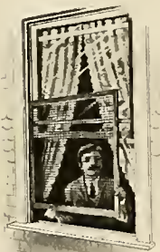
METHOD OF REMOVING SLIDING SCREEN
