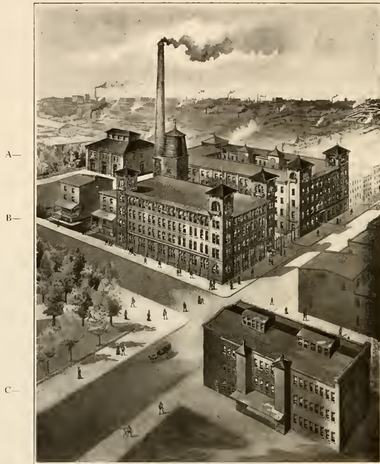
FIG. 13. NEW BUILDINGS OF THE VICTOR TALKING MACHINE COMPANY, CAMDEN, N. J. Buildings "A," "B" and "C" of Concrete reinforced with "Unit" Girder Frames
