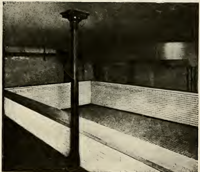
SWIMMING POOL, SAINT CHRISTOPHER HOUSE Barney & Chapman, Architects New York City Tiffany Enameled Bricks Used.
