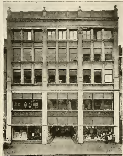
FIG. 5. STORE OF GILCHRIST & CO., BOSTON Luxfer Prisms in first Four Floors
