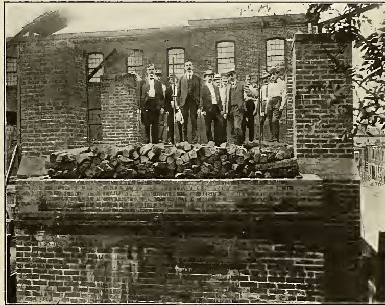
FIG. 12. LOADED CONCRETE ROOF AFTER FIRE TEST
