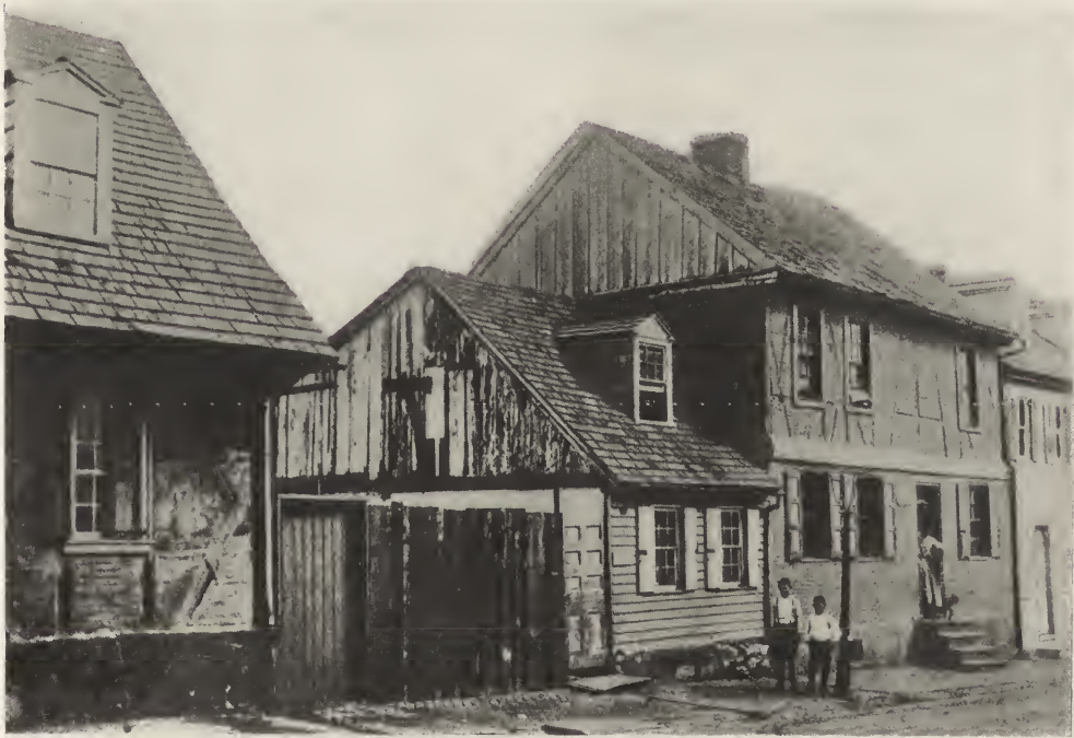
HOUSES FORMERLY STANDING ON EAST SIDE OF MIDDLE STREET, LANCASTER, PA., SHOWING HALF TIMBER CONSTRUCTION.
