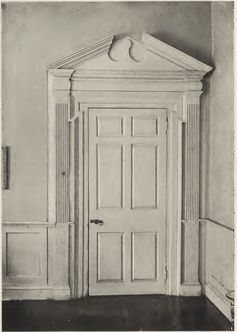
INTERIOR DOORWAY—EPHRAIM BLAINE HOUSE, CARLISLE, PA., 1796.
