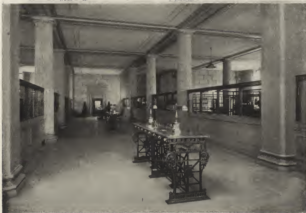
REAR END OF BANKING ROOM, MAIN AXIS—FIFTH AVENUE GUARANTY BUILDING, NEW YORK. CROSS & CROSS, ARCHITECTS.
