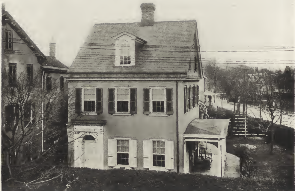
HOUSE AT 6105 MAIN STREET, GERMANTOWN, PA.
