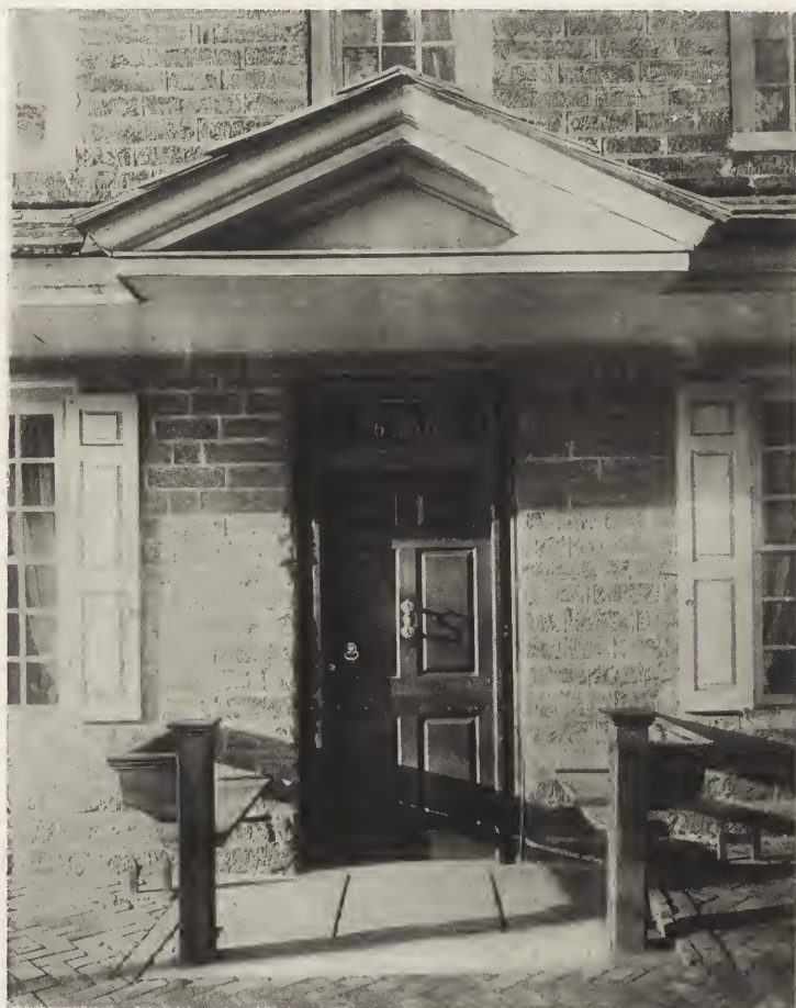
MAIN ENTRANCE—JOHNSON HOUSE, 6306 GERMANTOWN ROAD, GERMANTOWN, SHOWING CHARACTERISTIC HOOD AND "STOEP."
