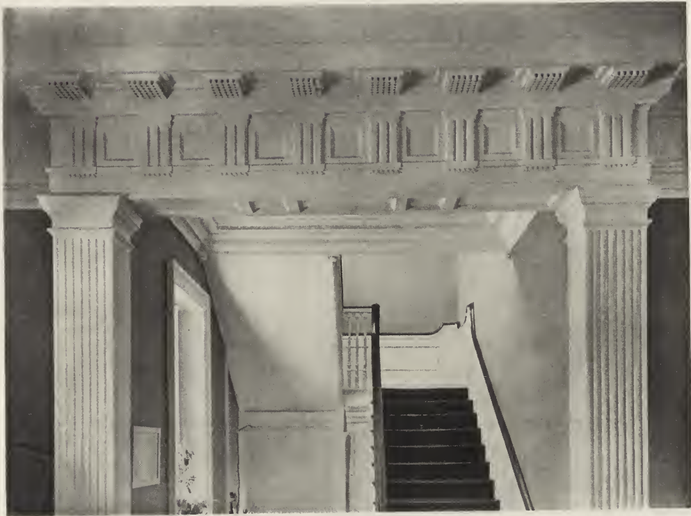
DETAIL SHOWING CORNICE AND STAIR HALL—MOUNT PLEASANT, FAIRMOUNT PARK, PHILADELPHIA, PA.
