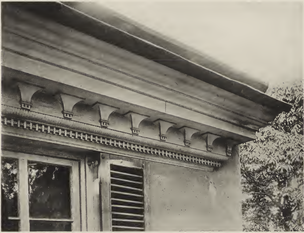
CORNICE DETAIL, ROXBOROUGH, PHILADELPHIA.
