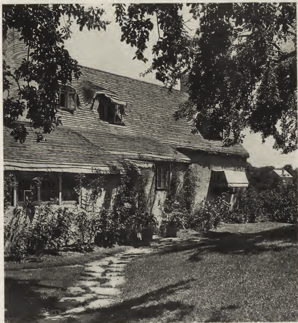
ENTRANCE FRONT—"LITTLE OR- CHARD FARM," WHITE PLAINS, N. Y. FRANK J. FORSTER, ARCHITECT.
