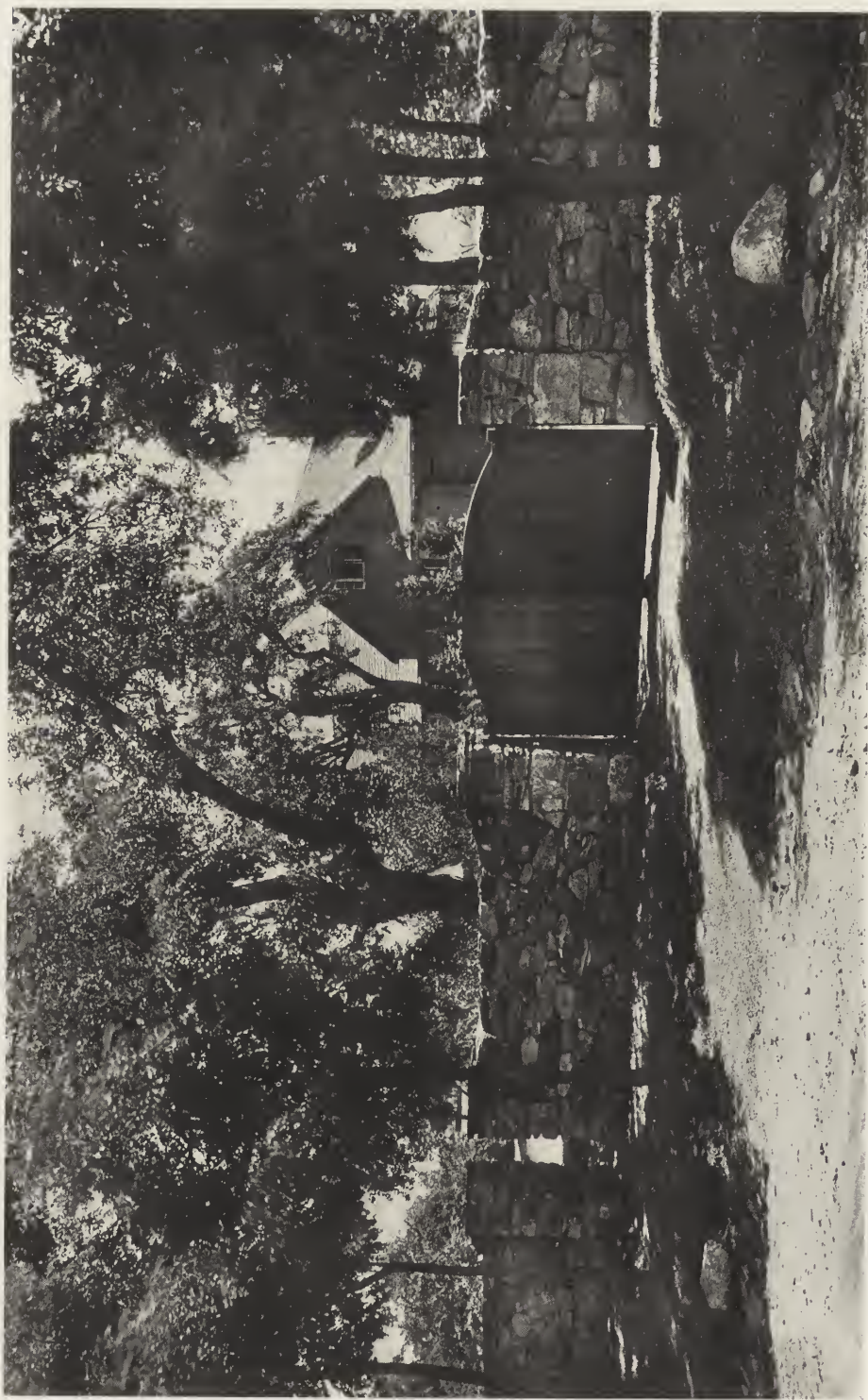
ENTRANCE GATES—"LITTLE OR- CHARD FARM," WHITE PLAINS, N. Y. FRANK J. FORSTER, ARCHITECT.
