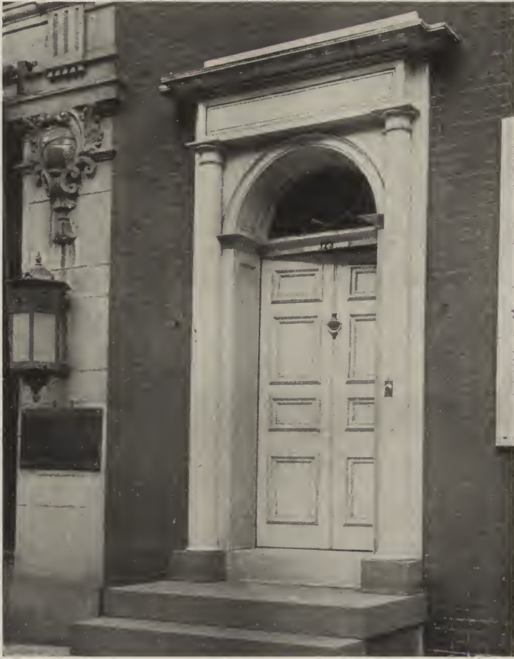
MAIN ENTRANCE AT 123 MARKET STREET, YORK, PA.
