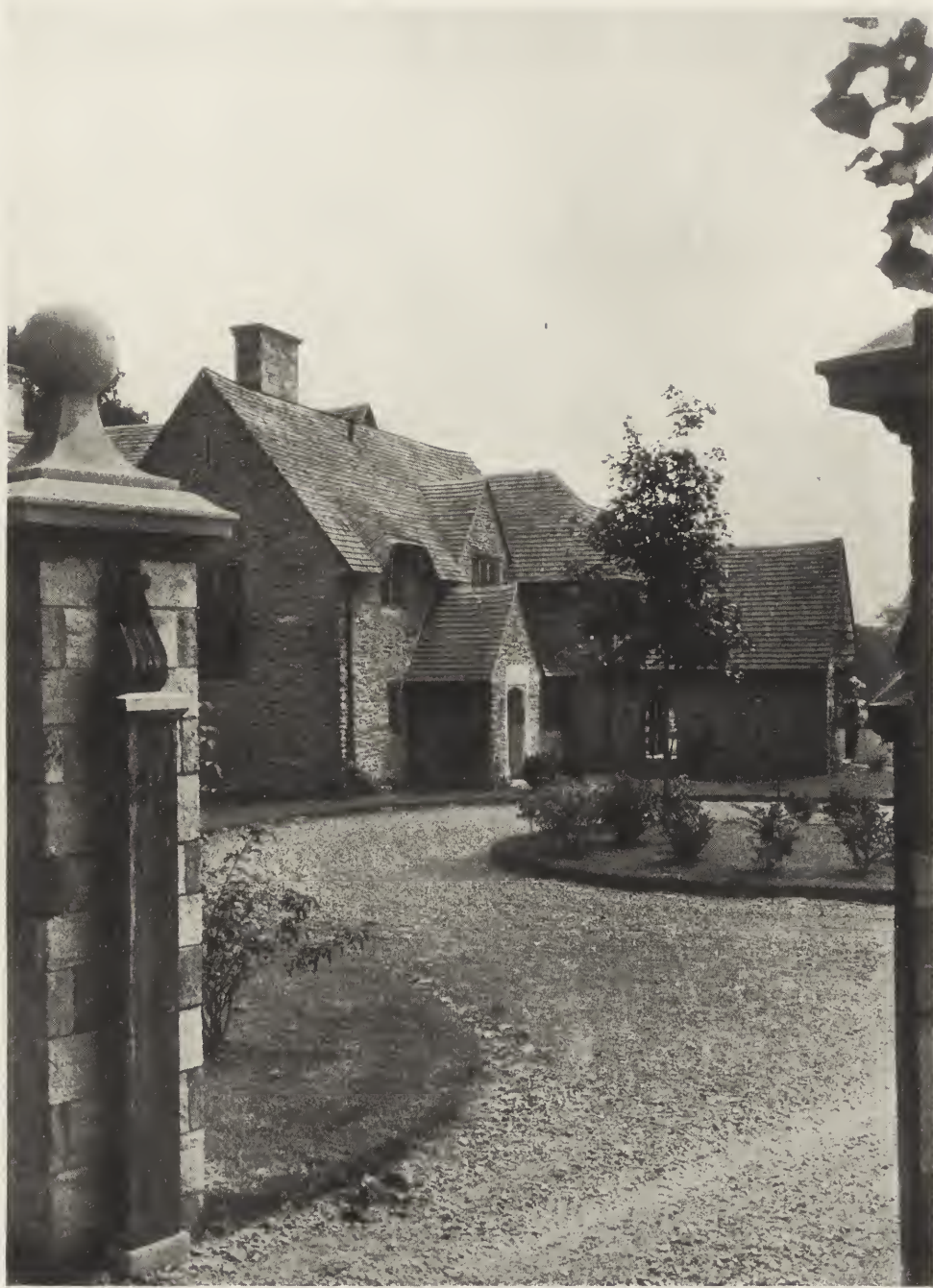
THE ENTRANCE COURT, FROM THE SERVICE GATE— RESIDENCE OF HEATLY C. DULLES, ESQ., VILLA NOVA, PA. MELLOR, MEIGS & HOWE, ARCHITECTS.
