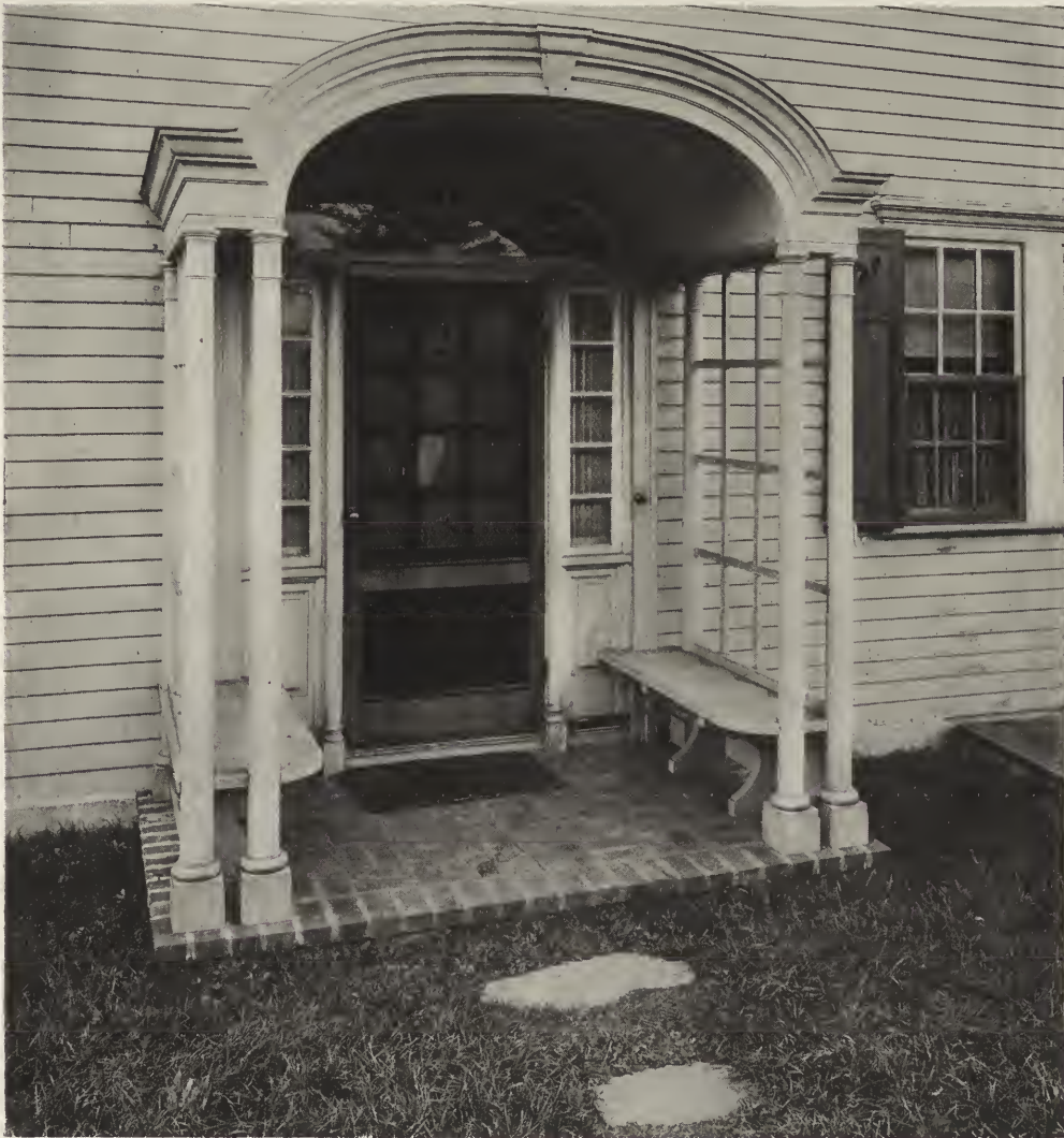
SOUTH DOOR—RESIDENCE OF HERBERT S. DREW, ESQ., BELMONT, MASS. GRANDGENT & ELWELL, ARCHITECTS.
