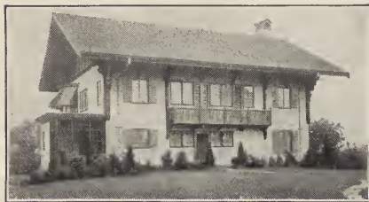
Res.—Mrs. Wm. B. Green, 133 Steele Road, W. Hartford, Conn. Architect—Russell E. Barker, 43 Ann St., Hartford, Conn. Gen'l Cont.—W. A. Wilcox, 327 Trumbull St., Hartford, Conn. Stucco Contractor—Peter Leone Bishopric Stucco Base used on Exteriors
