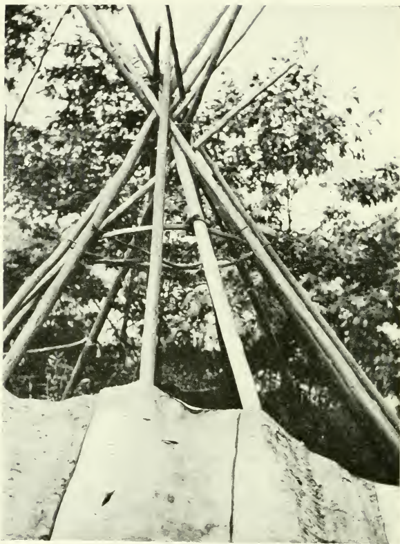
BIRCH-BARK WIGWAM OF THE CAPE BRETON MICMAC. SHOWING FEATURE OF THE HOOP AND THE INSIDE POLES FROM WHICH COOKING VESSELS ARE SUSPENDED AND CLOTHES HUNG TO DRY
