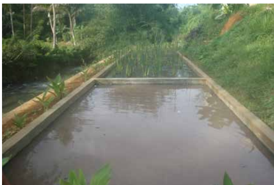
Figure 7.1.4 Artificial constructed wetland. Photo ©APCE
