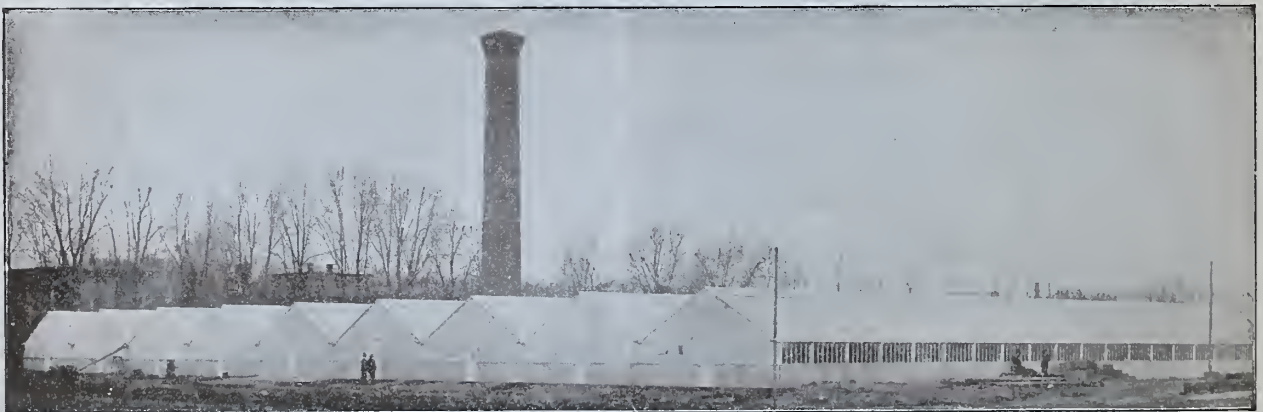
Outside view of the New Range of Palm Houses, containing 53,000 square feet of glass, erected in 1895. A similar block to this, also for Palms, was erected in 1896.
