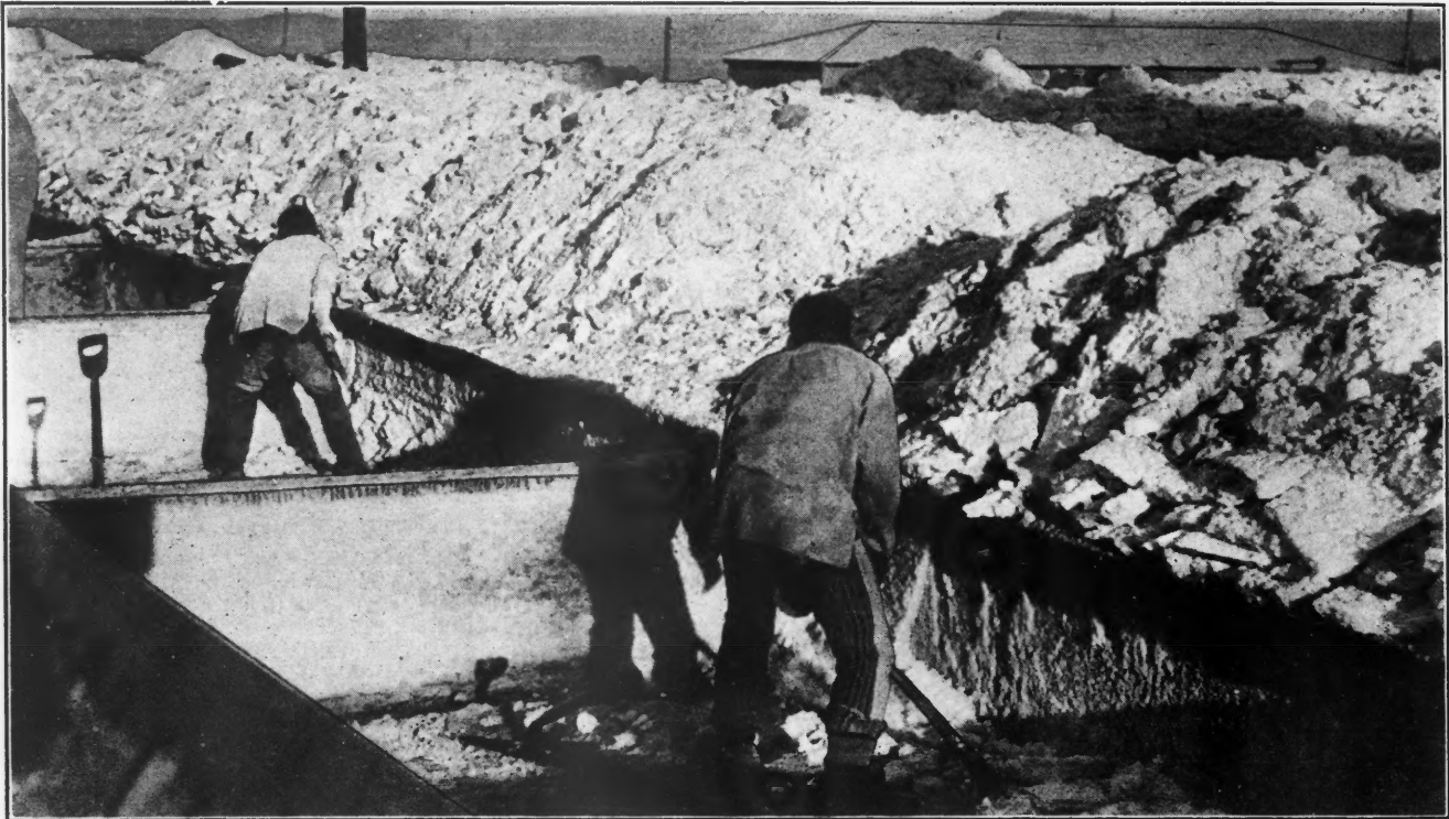
Copyright by Underwood & Underwood CHILE'S GREATEST EXPORT TRADE IS IN NITRATE. THE INDUSTRY IS DEPRESSED AT PRESENT, DUE TO HIGH PRICED STOCKS AVAILABLE ABROAD, AND THE DROP IN SALES. MORE THAN HALF THE OFICINAS HAVE SUSPENDED OPERATIONS, RESULTING IN UNEMPLOYMENT AND DISTRESS. THESE MEN ARE SHOVELING NITRATE, BENEATH A SCORCHING SUN, FROM A TANK ONTO A DRAINAGE BOARD
