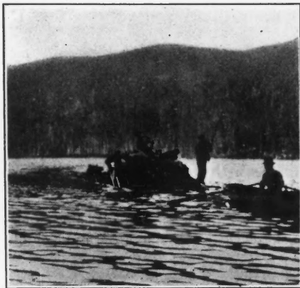
RAFT CARRYING DRILL OUTFIT PROPELLED BY DRILL ENGINE
