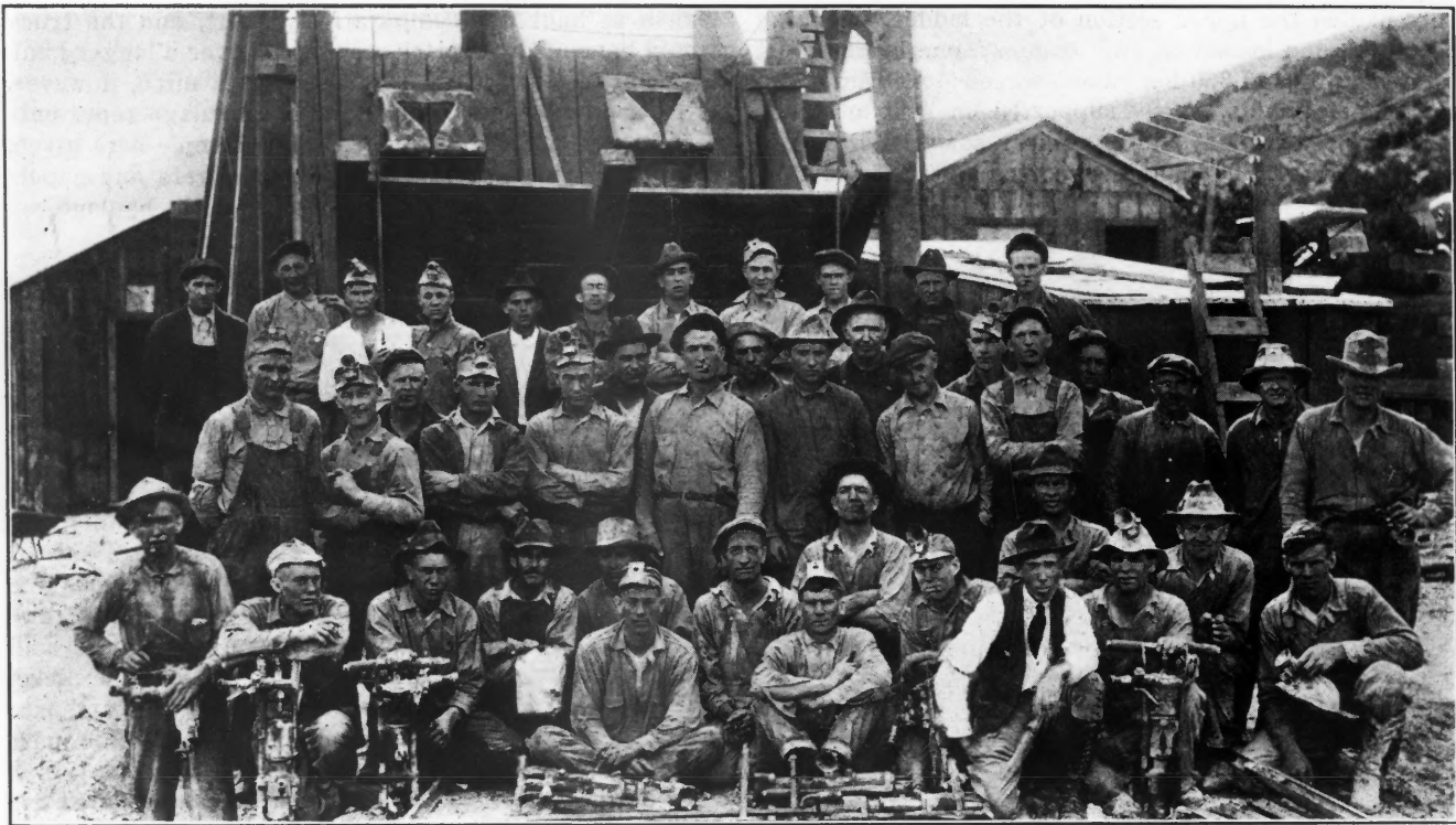
SHAFT SINKING CREW, WATER LILY SHAFT, EUREKA, UTAH
