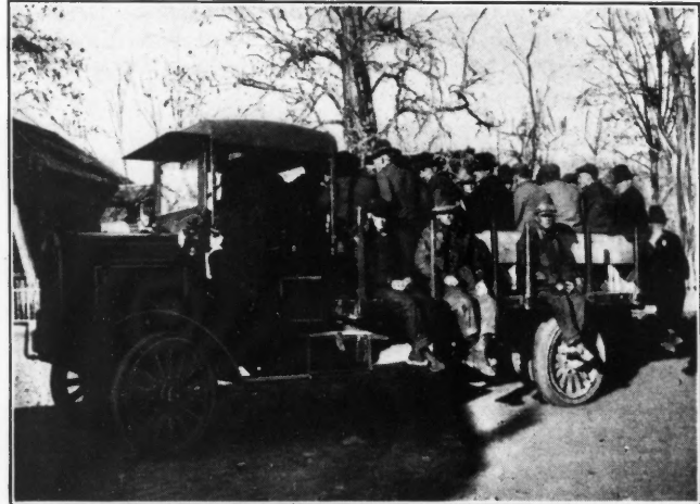
HAULING ERECTION CREW BETWEEN DAYTON AND DREDGE SITE
