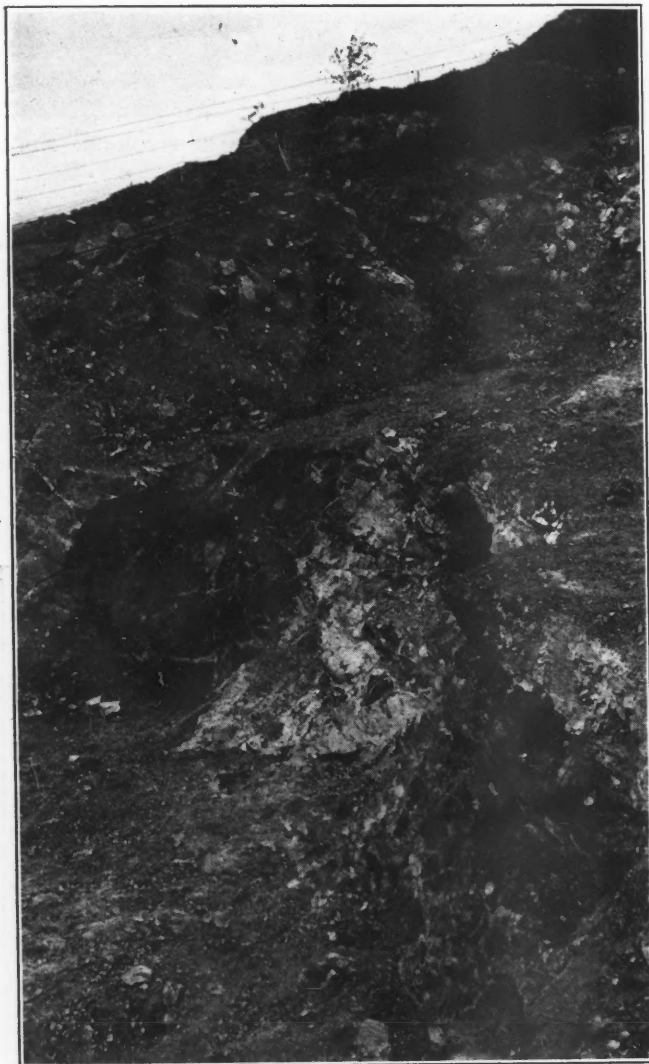
NO. 6 PIT OF BLACK LAKE ASBESTOS & CHROME CO. VEINS OF SERPENTINE SHOWING IN BENCH FACE. CABLES OF DERRICKS IN UPPER PART
