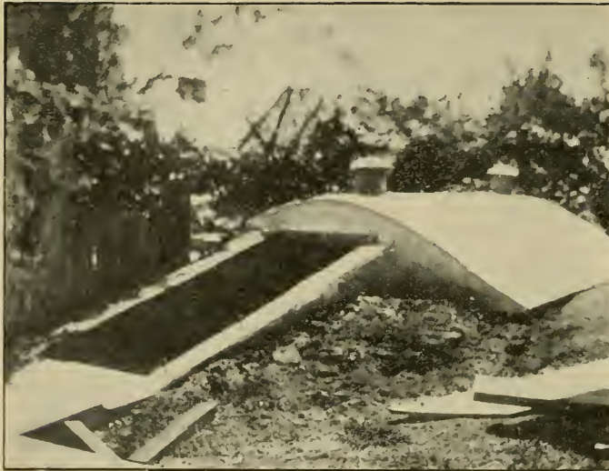
Cellar built entirely of concrete, including floor, walls, and roof.
