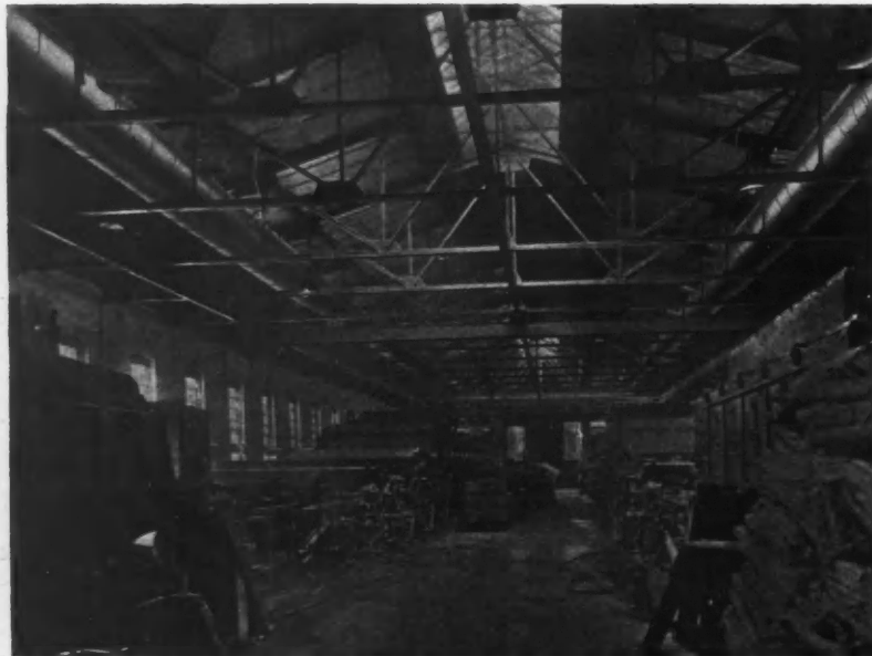
PARKER YOUNG CO., LINCOLN, N. H. REMOVING THE VAPOR AND AIR THROUGH THE ROOF WITHOUT THE USE OF HOOD AND SUPPLYING WARM DRY AIR MOSTLY AT THE ROOF LINE
