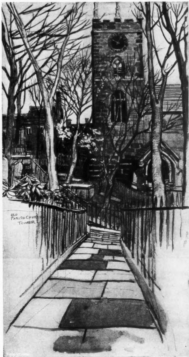
The Old Parish Church Tower.
