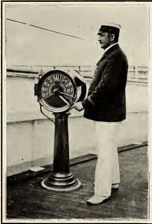
THE TELEGRAPH SIGNALS TO THE ENGINE ROOM.
