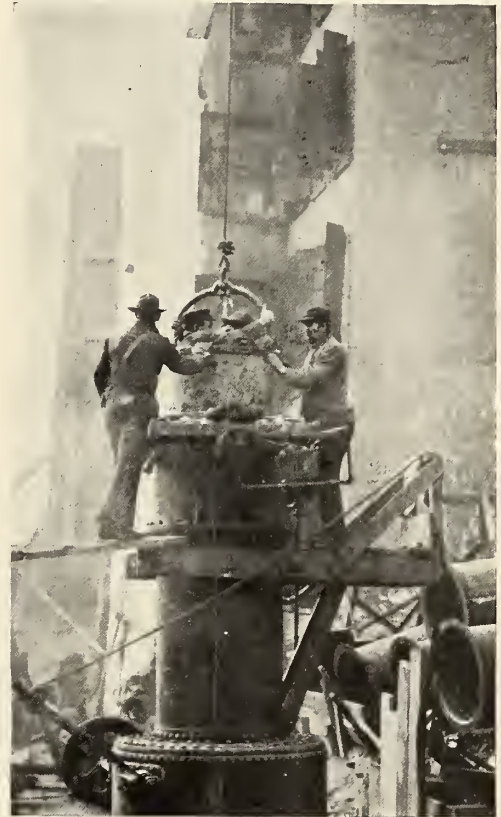
TWO MEN IN A BUCKET ENTERING A CAISSON.
