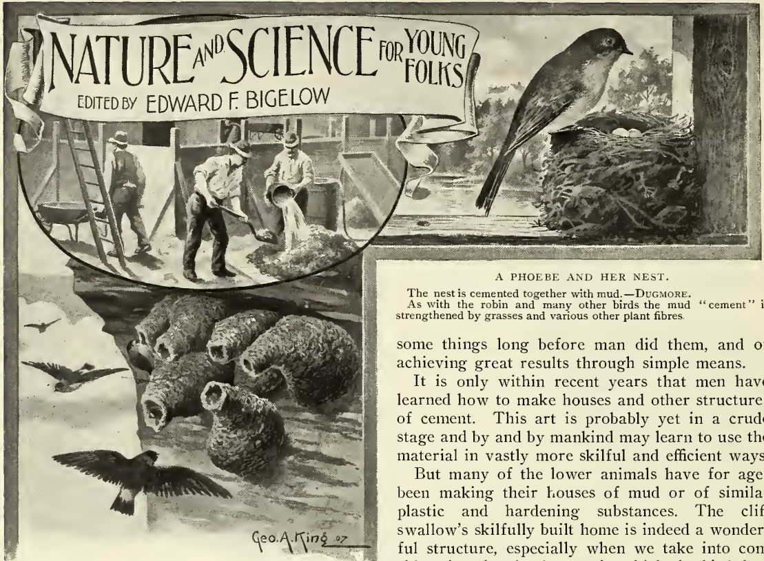
WORKMEN MIXING CEMENT FOR A BUILDING.
