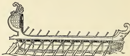
FIG. 3. A ROMAN GALLEY OF ONE TIER OF OARS, INTRODUCING THE RUDDER.
