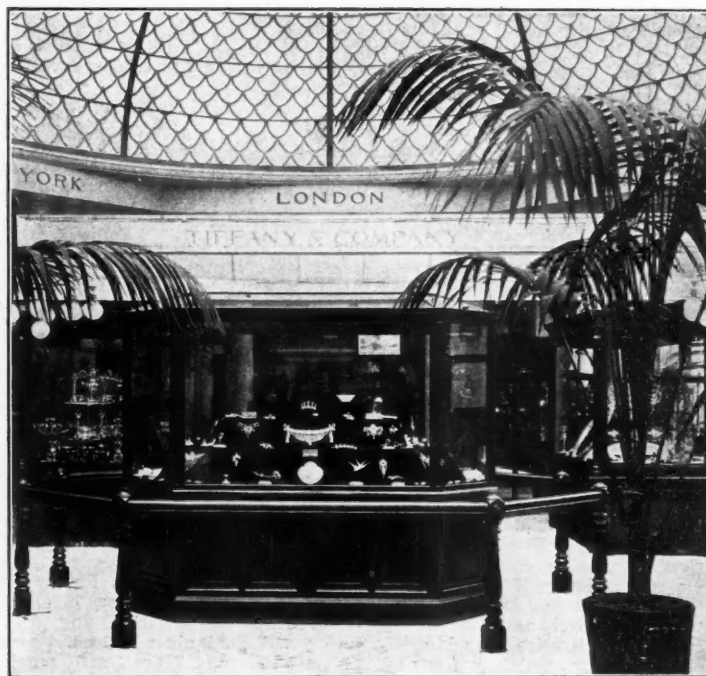
TIFFANY PAVILION IN MANUFACTURES BUILDING.
