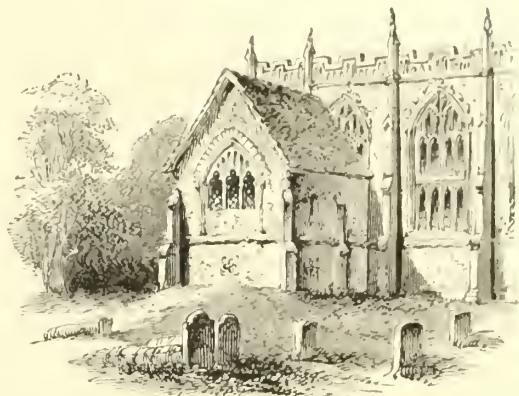
EXTERIOR OF THE CHARNEL HOUSE, STRATFORD.
