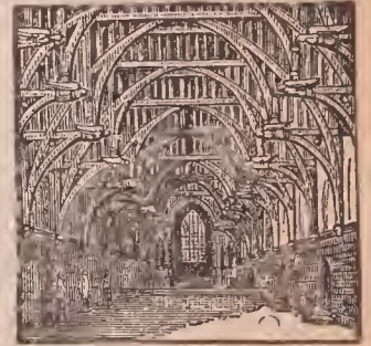
Roof-trusses, Westminster Hall, London.
