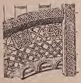
Reticulated-molding. (From Norman Arch, Tower of St. Peter's, Northampton, England.)
