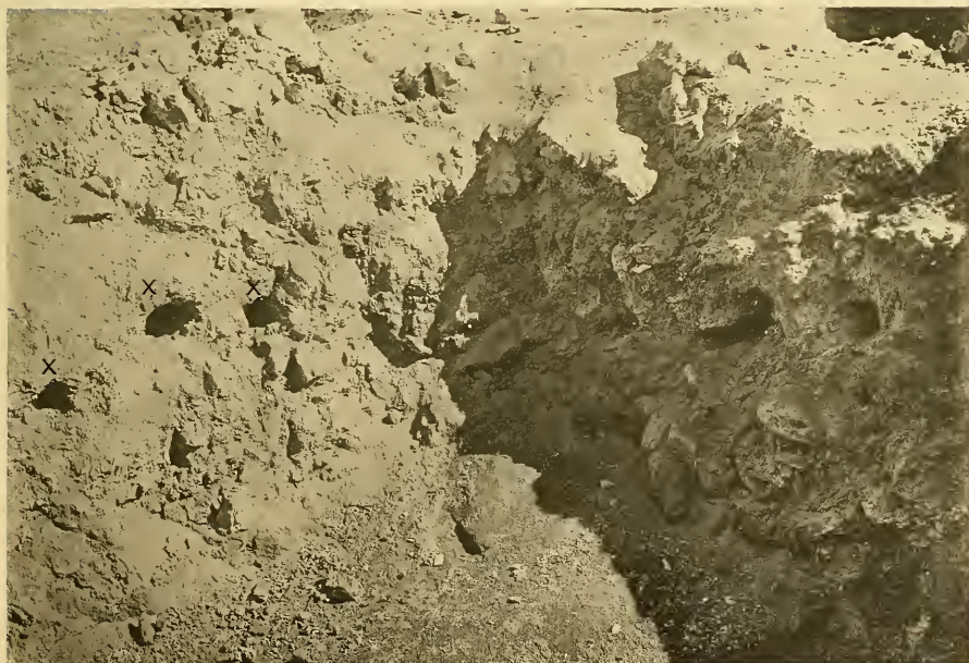
b. PG/777. INTERIOR OF THE CHAMBER SHOWING (X X X) THE HOLES IN THE STONWORK LEFT BY THE ROOFING-BEAMS. v. pp. 53, 233
