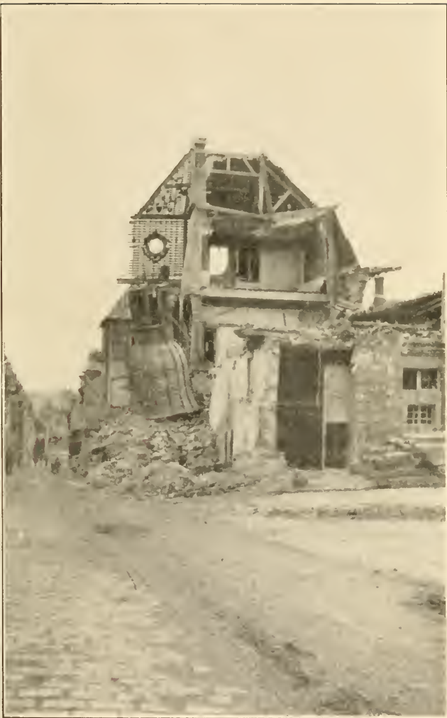
RUINS OF A HOUSE IN ROYE. PEOPLE ARE LIVING IN THE LOWER RIGHT-HAND CORNER
