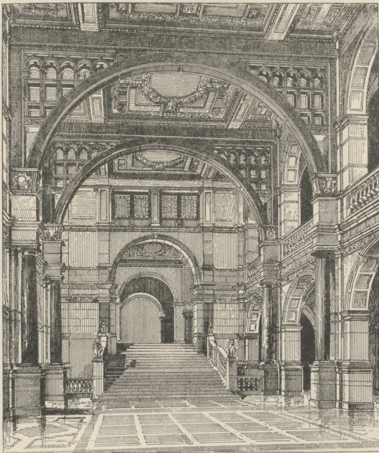
FIG. 11.—Staircase, Imperial Institute. (Collett.)
