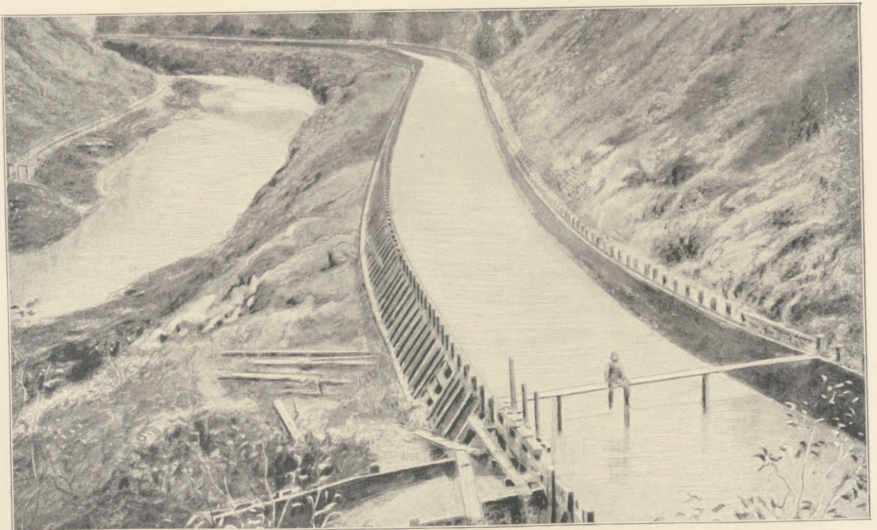
WOODEN AQUEDUCT OR FLUME.
