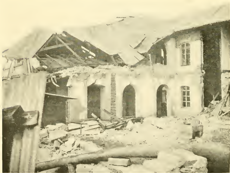
The Overturned Tower of Carmen Church, Cartago. The Wrecked Schoolhouse next to Weldon's Hotel.
