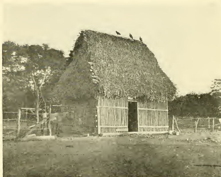
Plaza, Bare Hills and Schoolhouses, Bolsón. Bamboo House with Palm-thatched Roof at Bolsón. Sawing Stage in left background.
