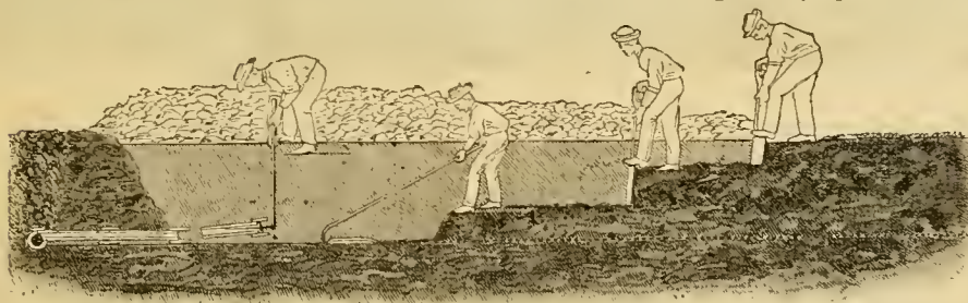
Fig. 6.—OPENING THE DITCH AND LAYING THE TILES.
