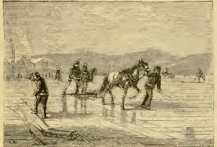
Fig. 2.—MARKING AND CUTTING.
