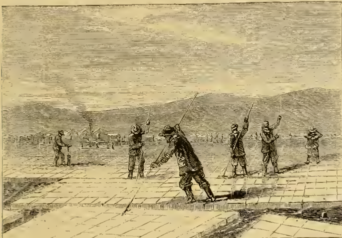
Fig. 3.—SAWING AND BARRING OFF.
