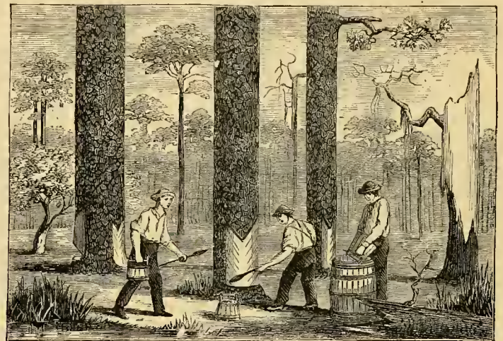
Fig. 2.—DIPPING THE CRUDE TURPENTINE.
