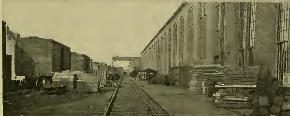
FIG. 72.—SIDE VIEW OF THE PAINT AND FREIGHT CAR SHOPS. PAINT SHOP AT THE RIGHT. FIG. 74.—ONE DAY'S OUTPUT. FIG. 73.—THE FINISHED CAR, READY FOR WEIGHING. FIG. 71.—STORAGE OF MATERIAL ALONG THE NORTH SIDE OF THE CAR SHOP.
