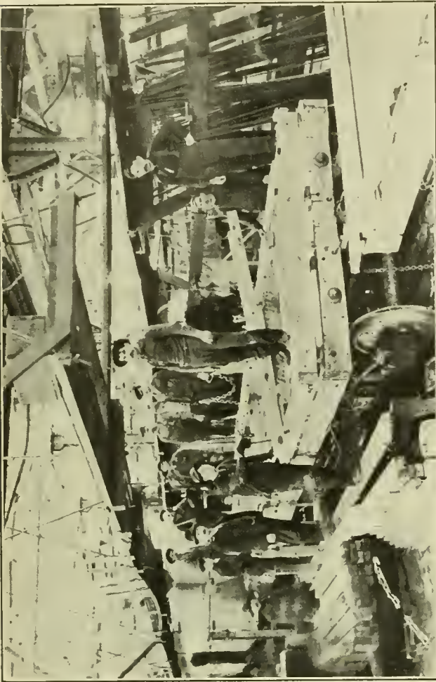
FIG. 63.—FOURTH STAGE—THE ROOF FRAME IS ABOUT TO BE RAISED.
