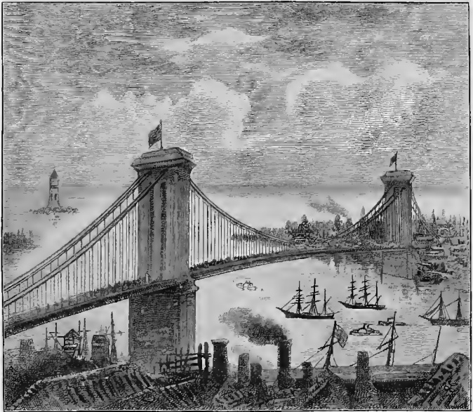
FIG. 18.—BROOKLYN SUSPENSION BRIDGE, THE LARGEST IN THE WORLD.
