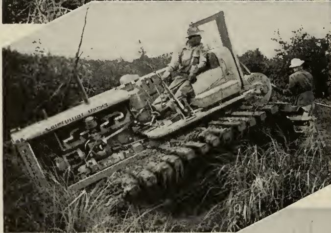
FIG. 13, above: Only the winch power of the head tractor makes possible the plowing-in of cable here. FIG. 14, left: Oak "swamp grousers" on caterpillar tracks increase the supporting surface. FIG. 15, below: The skid under the plow helps to support the down thrust of the tongue
