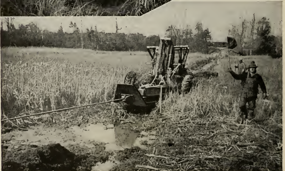
FIG. 13, above: Only the winch power of the head tractor makes possible the plowing-in of cable here. FIG. 14, left: Oak "swamp grousers" on caterpillar tracks increase the supporting surface. FIG. 15, below: The skid under the plow helps to support the down thrust of the tongue
