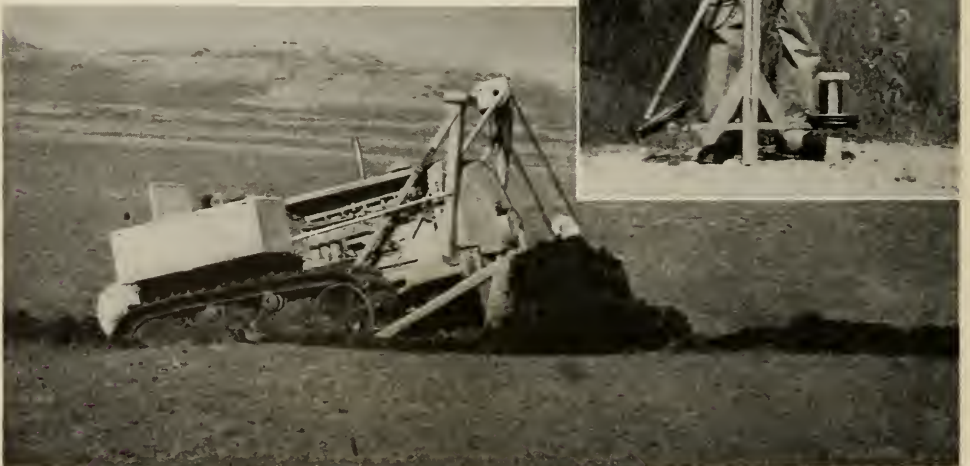
FIG. 8, right: "Buried treasure" detector—an electrical device which accurately locates underground pipes and cables both laterally and in depth. FIG. 9, below: A bulldozer at work. Leveling off sharp dips in uneven ground makes the subsequent passage of the plow train easier
