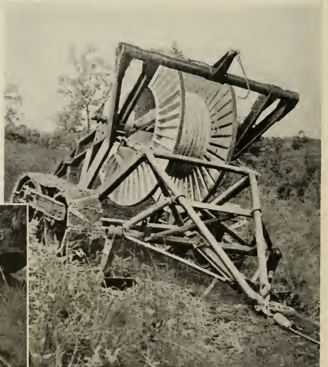
FIG. 21, right: Release of the relay winch has halted the rear trailer. The bullet-nose connector is shown at the end of the trailer tongue, at the lower right. FIG. 22, below: This keeper, under the axle of the front trailer, receives the bullet-nose connector, which is held by tension on the rope from the tractor ahead
