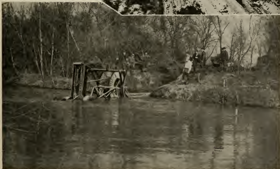
FIG. 16, above: The skid under the trailer gives additional support over soft ground. FIG. 17, right: Here the problems are depth and density of mud, weight of equipment, supporting area, and winch power. FIG. 18, below: The plow continues to bury cable as it is winched across the river
