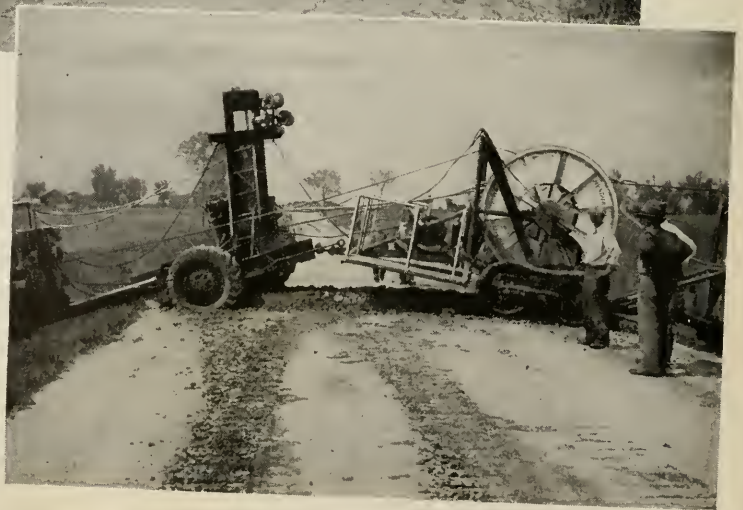
FIG. 12. A bulldozer "eased off" the sharp drop of the ditch banks in preparation for a square crossing of this road. Road surface and shoulders and ditch banks are always restored to their original condition
