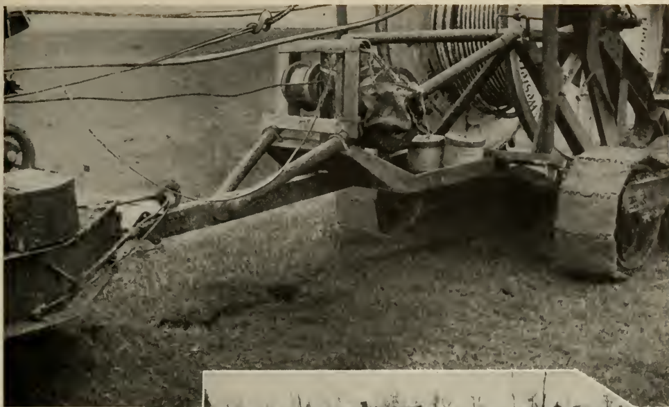
FIG. 16, above: The skid under the trailer gives additional support over soft ground. FIG. 17, right: Here the problems are depth and density of mud, weight of equipment, supporting area, and winch power. FIG. 18, below: The plow continues to bury cable as it is winched across the river
