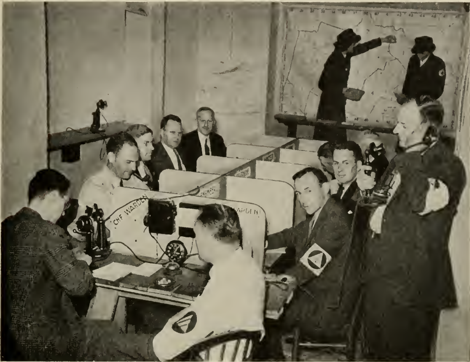
THE CONTROL ROOM OF A CONTROL CENTER
