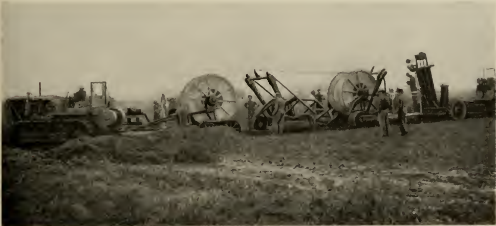
FIG. 30. CHANGING REELS ON THE REAR TRAILER
