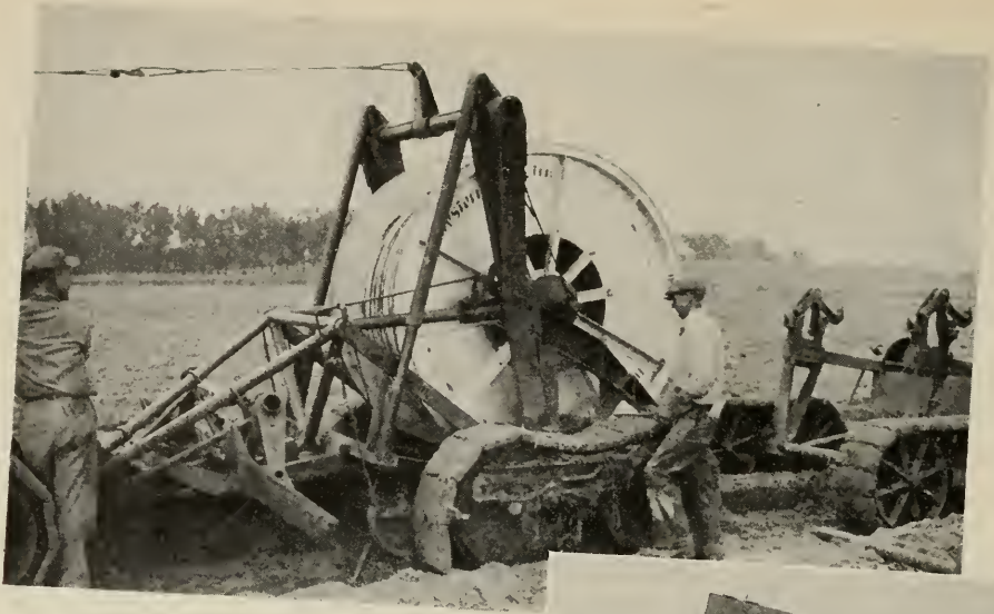
FIG. 23, above: Loading a reel of cable onto a trailer. The yoke is being pulled up by a line from a multi-drum tractor winch, and the latches will catch the spindle after another foot of travel. FIG. 24, right: The share of the cable-laying plow is in its upper position, so that the cable can be fed through it at the start of a laying operation. FIG. 25, below: This is how twin cables feed out through the foot of the plow share and are pulled through and staked before the train moves ahead
