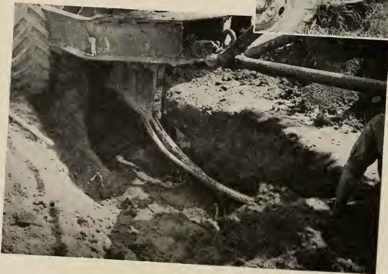
FIG. 23, above: Loading a reel of cable onto a trailer. The yoke is being pulled up by a line from a multi-drum tractor winch, and the latches will catch the spindle after another foot of travel. FIG. 24, right: The share of the cable-laying plow is in its upper position, so that the cable can be fed through it at the start of a laying operation. FIG. 25, below: This is how twin cables feed out through the foot of the plow share and are pulled through and staked before the train moves ahead
