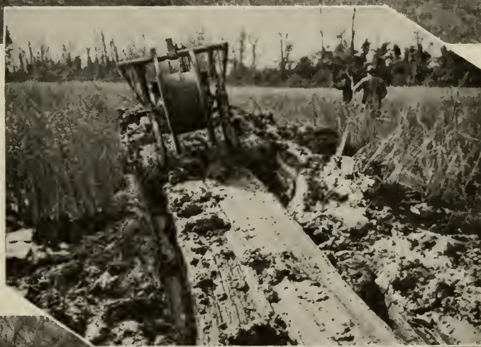
FIG. 16, above: The skid under the trailer gives additional support over soft ground. FIG. 17, right: Here the problems are depth and density of mud, weight of equipment, supporting area, and winch power. FIG. 18, below: The plow continues to bury cable as it is winched across the river
