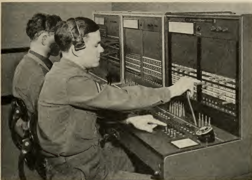
AN AIR RAID WARNING SWITCHBOARD
