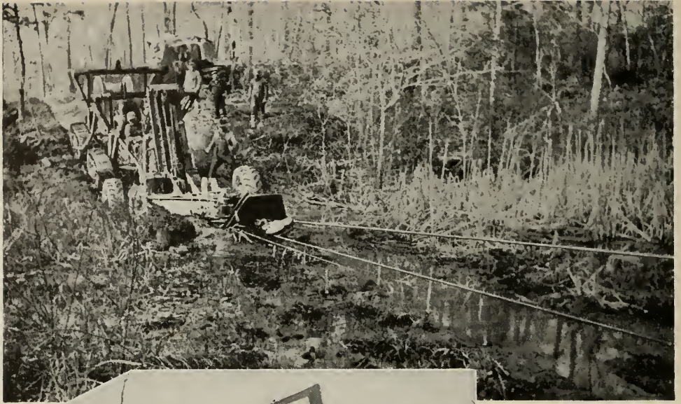
FIG. 13, above: Only the winch power of the head tractor makes possible the plowing-in of cable here. FIG. 14, left: Oak "swamp grousers" on caterpillar tracks increase the supporting surface. FIG. 15, below: The skid under the plow helps to support the down thrust of the tongue
