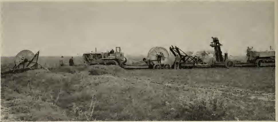
FIG. 29. CHANGING REELS ON THE FRONT TRAILER
