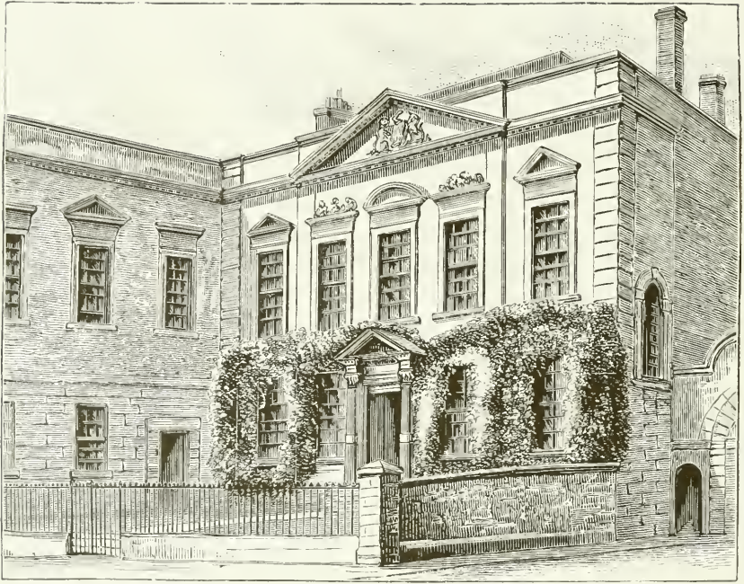
OLD CITY LIBRARY, KING STREET.
