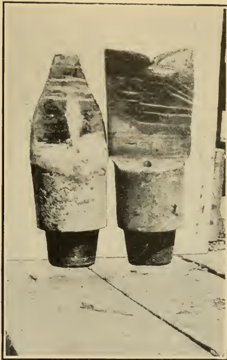
1. ROTARY BITS BEFORE AND AFTER DRILLING IN HARD SAND.
