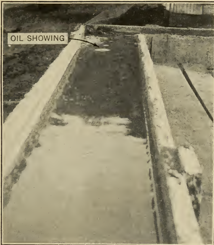
ROTARY DITCH WITH OIL SHOWING ON MUD STREAM.
