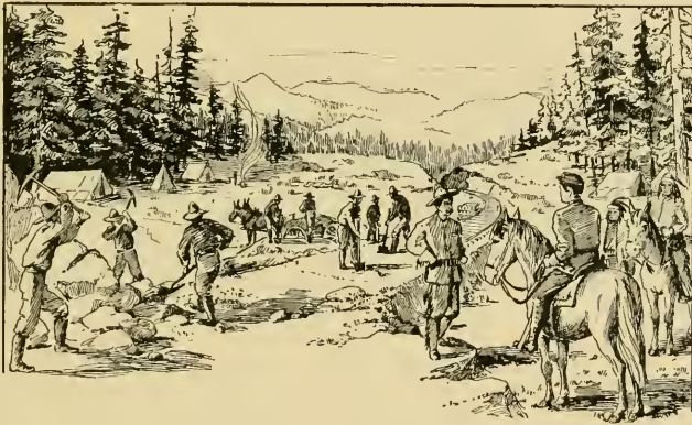
BUILDING THE FIRST TRANS-CONTINENTAL RAILROAD.
