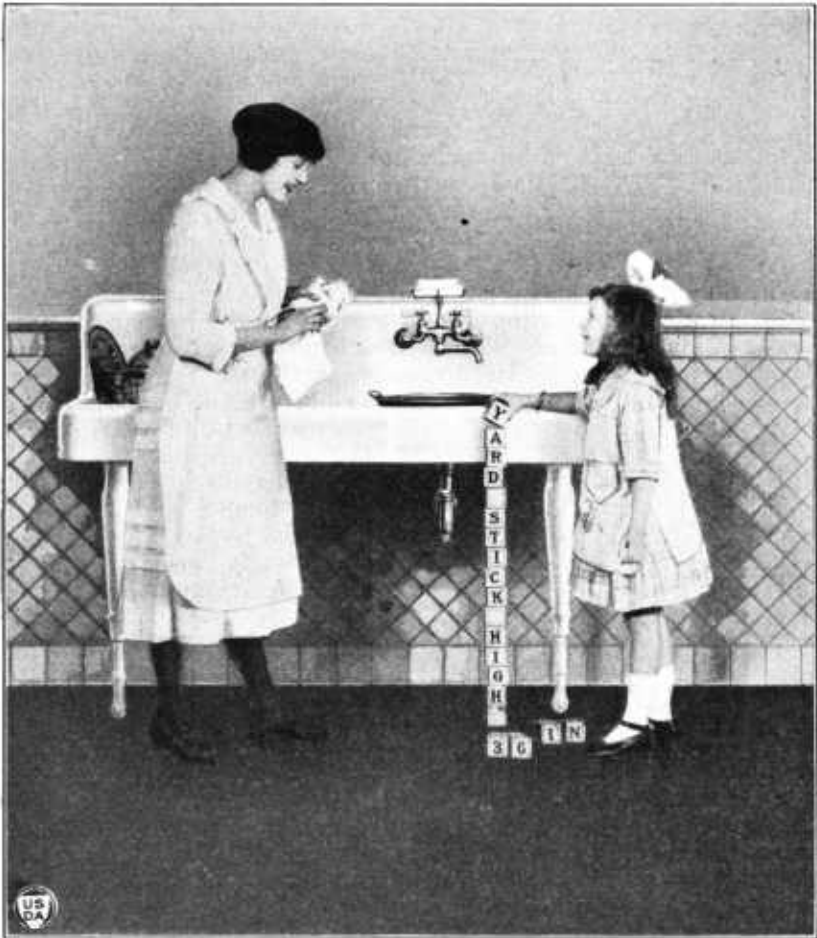
FIG. 29.—An enameled-iron apron sink with integral back and combination swing faucet. Every housewife should determine by experiment how high her sink should be set to give an easy, erect, working position; for a woman of average stature a favorable height to the top of the apron or rim is 36 inches (yard-stick high)
