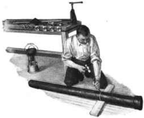
FIG. 9.—Cutting cast-iron soil pipe with a cold chisel
