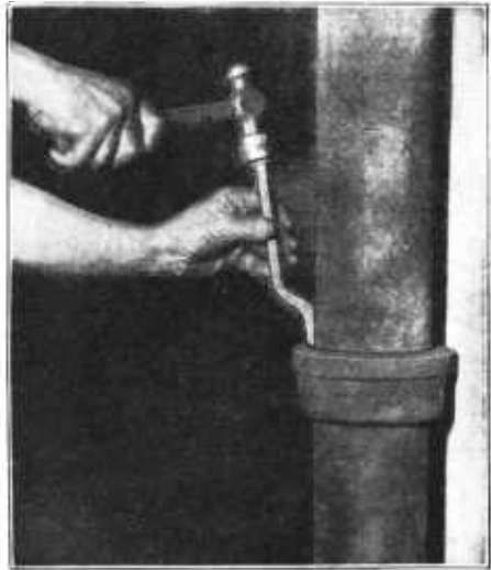
FIG. 13.—Calking a lead joint to make it air-tight and water-tight
